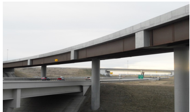
Figure 16: Curved Girder Bridge Example (Southbound Deerfoot Trail to Eastbound Stoney Trail NE, Calgary, Alberta)
