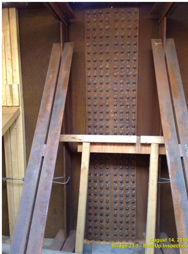
Figure 8: Field Splice [Courtesy of AECOM]
