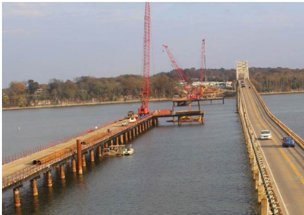
Figure 11: Lake Barkley trestle bridge installation.
