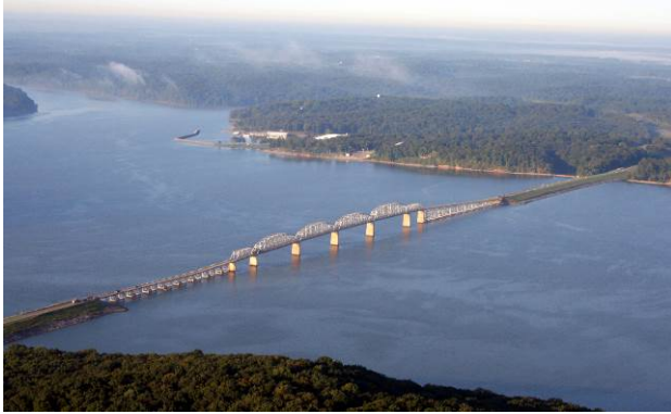
Figure 3: Existing Eggners Ferry Bridge.
