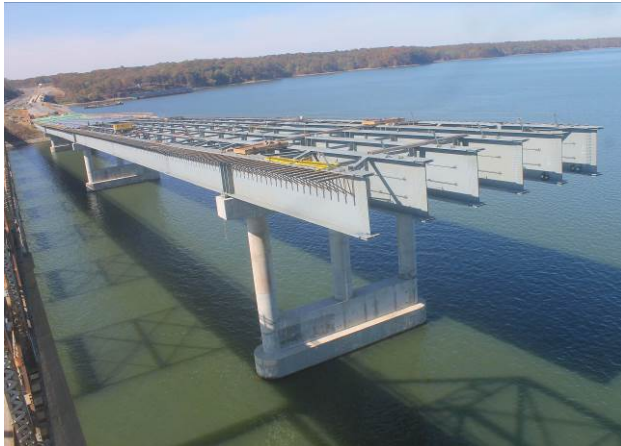
Figure 10: Kentucky Lake approach girders.
