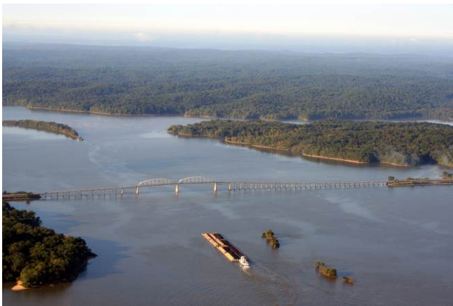
Figure 4: Existing Lawrence Memorial Bridge.
