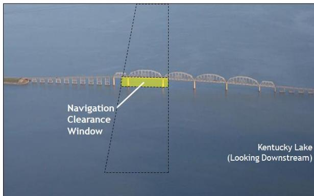
**Figure 4: Egner’s Ferry Bridge with Navigation Window of the New Kentucky Lake Bridge Shown**
