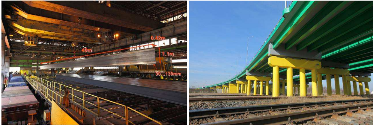
Figure 1: Left: view of rolled section at the rolling mill; Right: view of steel-concrete composite deck with rolled girders
