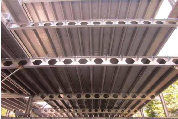
Figure 21: Angelina™ floor beams in combination with a specific composite floor beams with deep steel decking
