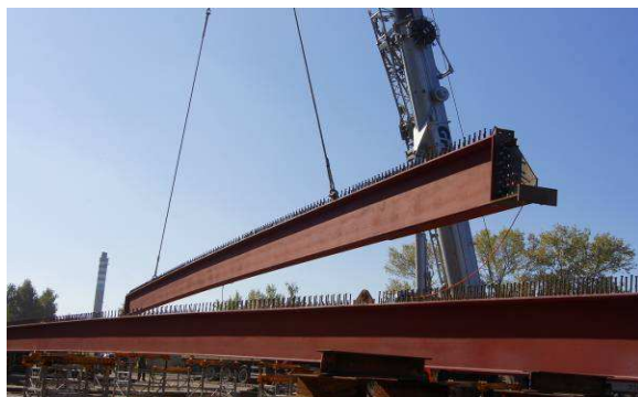
Figure 15: Fully-finished bridge girder on the construction site ready for installation [13]
