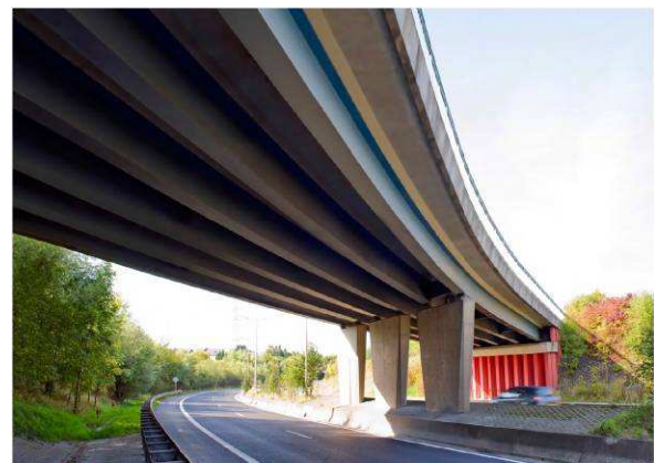
Figure 17: Composite bridge deck with plain curvature [6]
