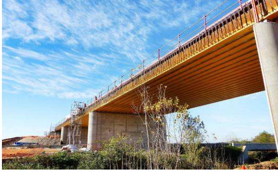
Figure 10: Filler beam deck before concreting [15]
