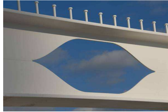
Figure 19: Innovative web opening design for Angelina™ beams [16]
