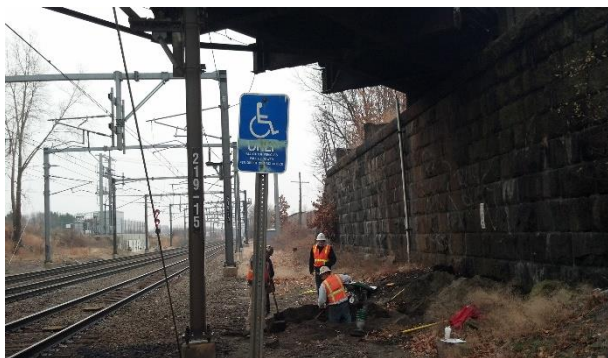
Figure 8: Test Pits to Discover Presence of Unknown Utilities
