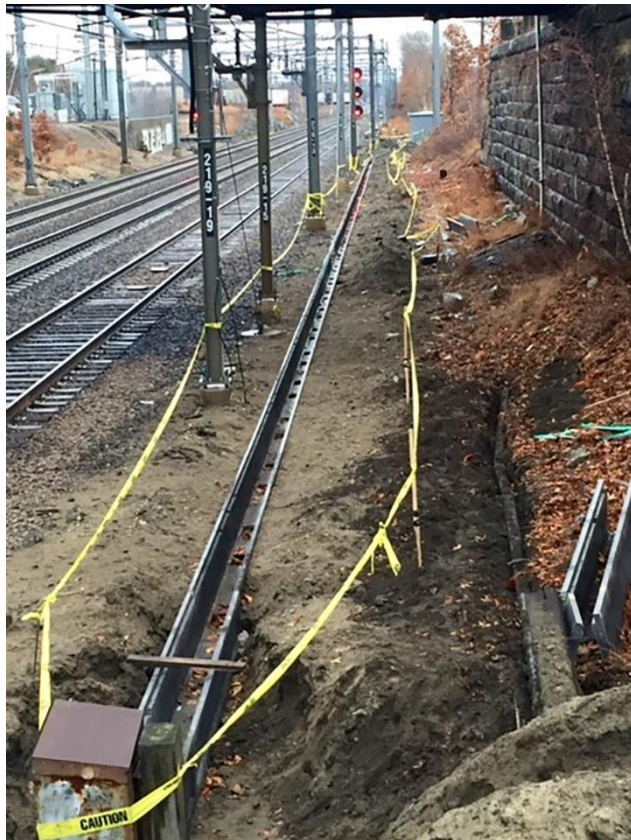
Figure 7: Relocation of Amtrak System Cables
