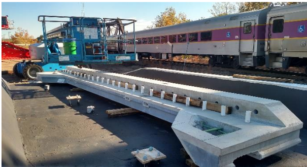
Figure 12: Prefabricated Backwalls
