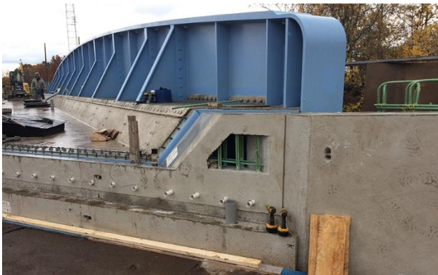
Figure 15: Backwall Placement
