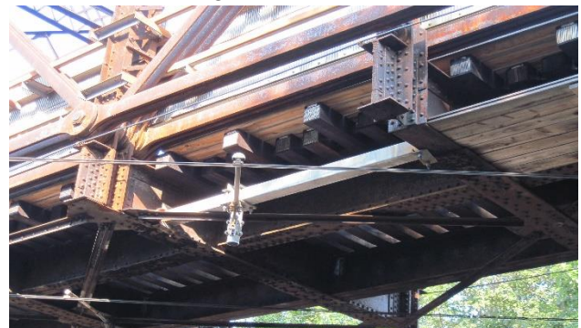
Figure 3: Truss Underside with Amtrak 25,000 Volt Overhead Catenary Wires
