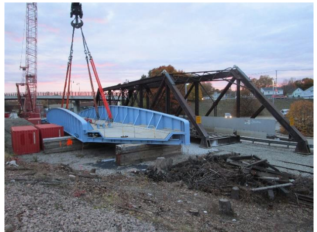
Figure 14: New Superstructure in Lifting Position
