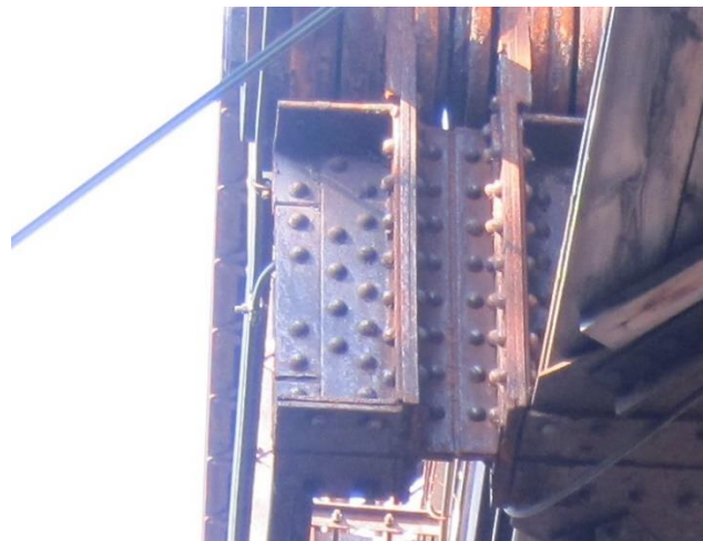
Figure 6: Cut-off Floor Beam Ends
