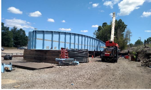
Figure 11: Prefabricated Steel Bridge Superstructure in Staging Area
