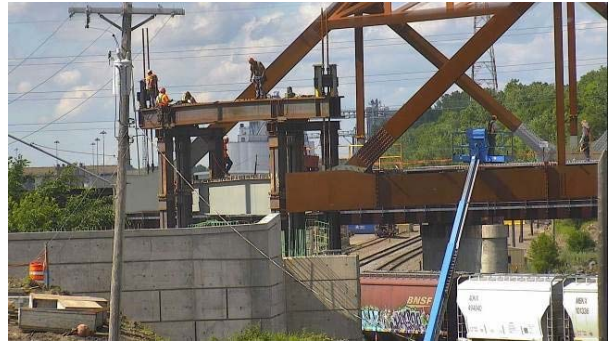
Figure 13 - Lowering New Truss onto Bearings
