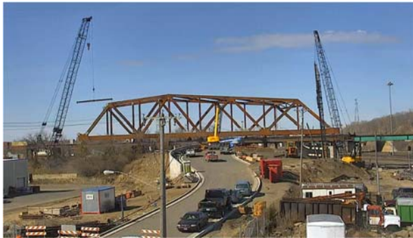
Figure 11 - Field Assembly of New Truss
