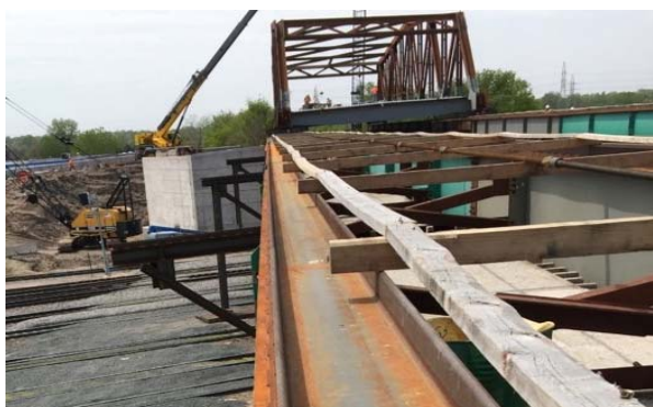
Figure 12 - Lateral Girder Launching System
