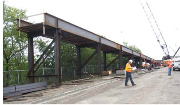
Figure 4 - Western Approach Embankment
