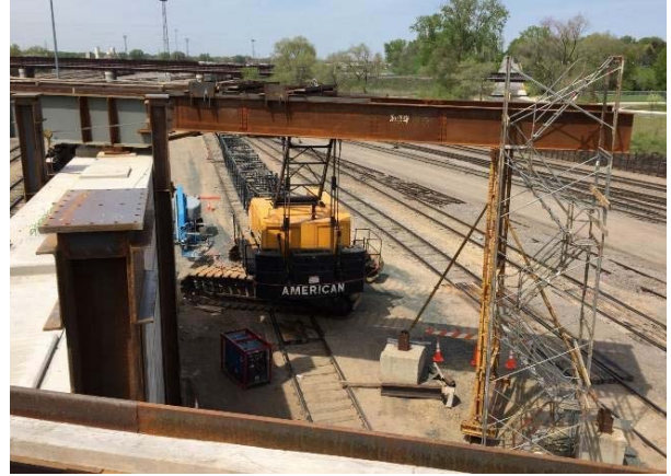
Figure 9 - Setup for New Truss Launch
