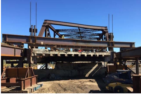
Figure 7 - Transverse Beam Setup
