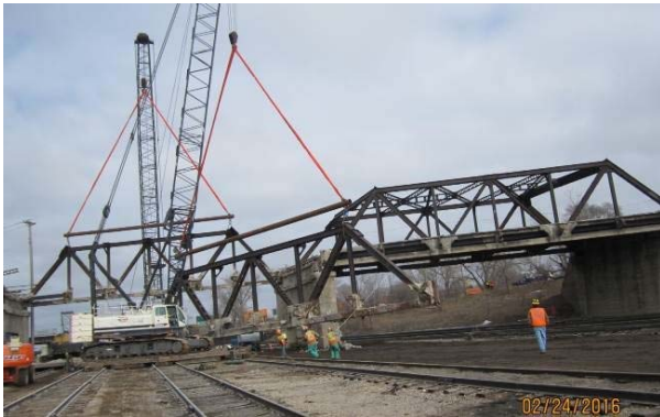
Figure 3 - Removal of Eastern Trusses
