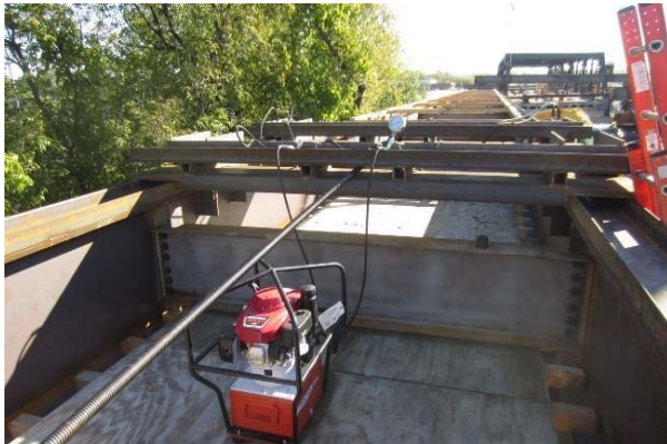
Figure 8 - Longitudinal Jacking Setup
