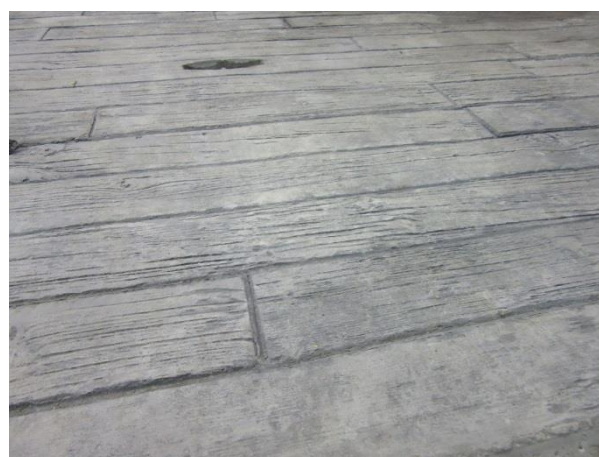
Figure 21 – Stamped Concrete Sidewalk Surface
