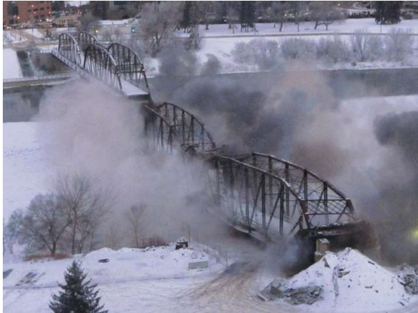
Figure 22 – Explosive Demolition of Spans 3 & 4
