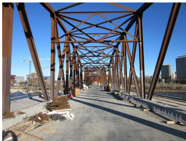
Figure 27 – Sidewalk Panels in Place
