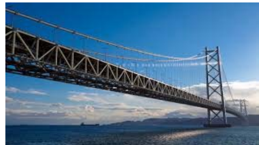
Figure 2: Akashi Kaikyo Bridge (Chou, 2011).
