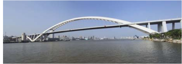
Figure 1: Lupu Bridge (GSG, 2013).
