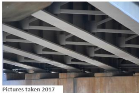
Figure 4. Virginia DOT; I-64 over Simpson Creek in Clifton Forge, VA. Repainted with PAS system in 2005. After 12 years in-service, <0.1% rusting over entire structure
