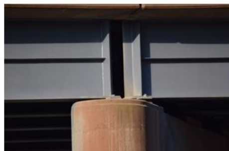
Figure 4. Virginia DOT; I-64 over Simpson Creek in Clifton Forge, VA. Repainted with PAS system in 2005. After 12 years in-service, <0.1% rusting over entire structure
