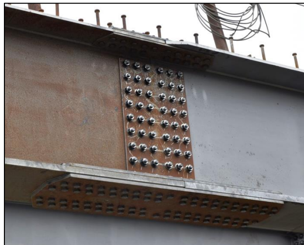
Figure 10. Rt. 340 Bridge bolted splice after installation of B8-2 bolts.
