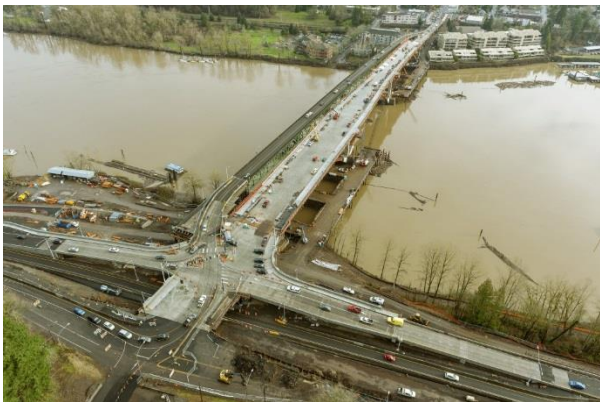
Figure 9: Detour Alignment During Construction
