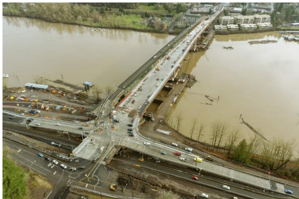
Figure 9: Detour Alignment During Construction
