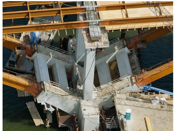
Figure 5: Y-Arm Extensions from Substructure
