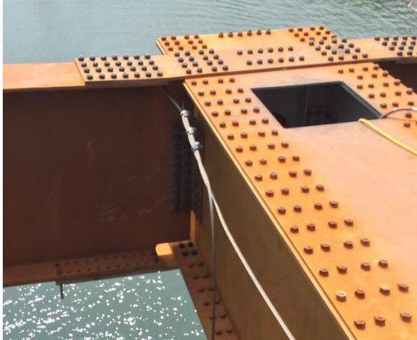
Figure 4: Girder to Spandrel Cap Connection
