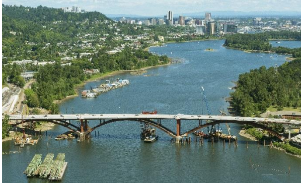
Figure 1: Sellwood Bridge South of Portland
