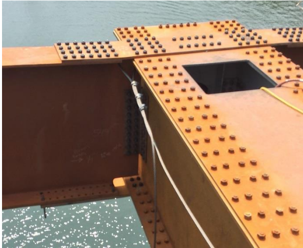
Figure 4: Girder to Spandrel Cap Connection
