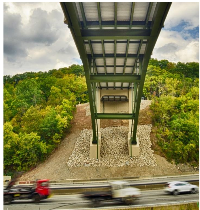
Figure 9: View of Vierendeel Bracing System
