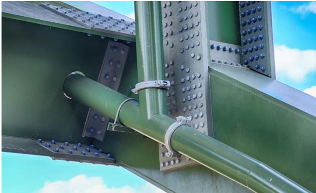
Figure 10: Spandrel and Vierendeel Strut Connections
