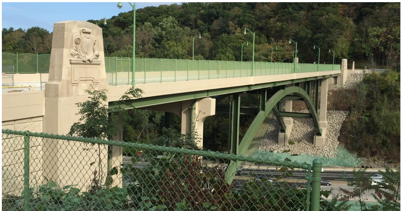
Figure 5: The New Steel Open Spandrel Arch in fall of 2017
