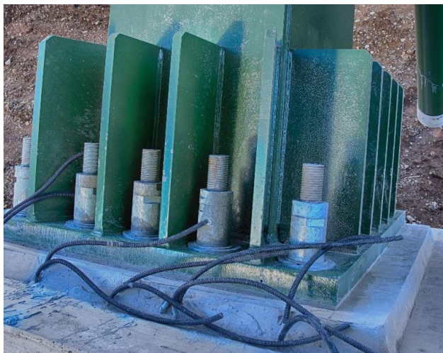
Figure 13: Grouted Base Plate Connection
