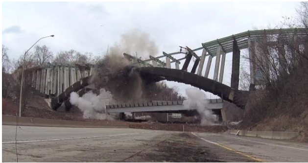
Figure 7: Implosion of the Existing Concrete Arch
