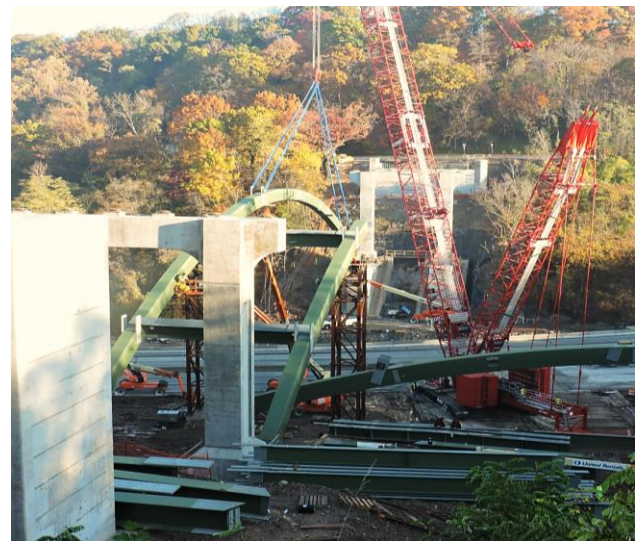
Figure 12: Erection of Arch Rib
