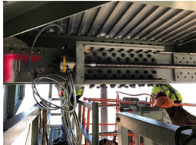
Figure 9: Post Tensioning Installation
