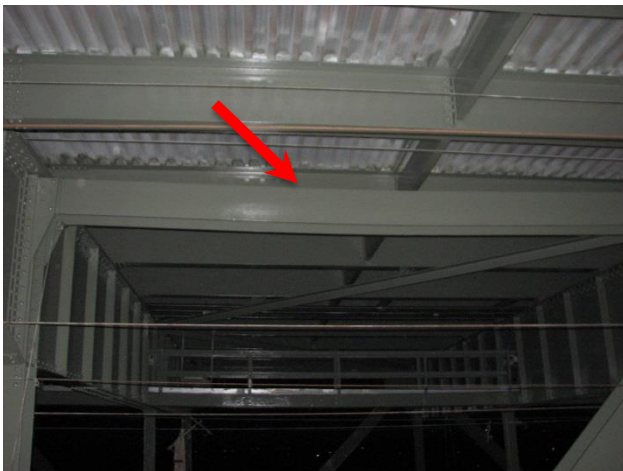
Figure 2: Installed Emergency Splice
