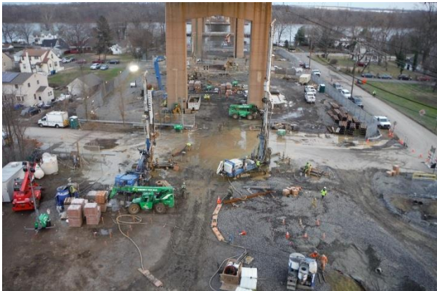
Figure 5: Micropile Installation
