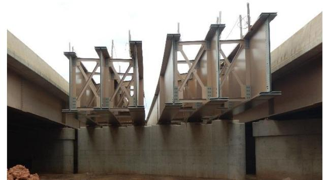
**Figure 15:** Broad Run girders during construction.
