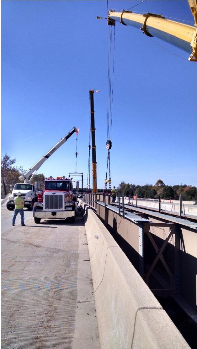
**Figure 16:** Broad Run girder erection.
