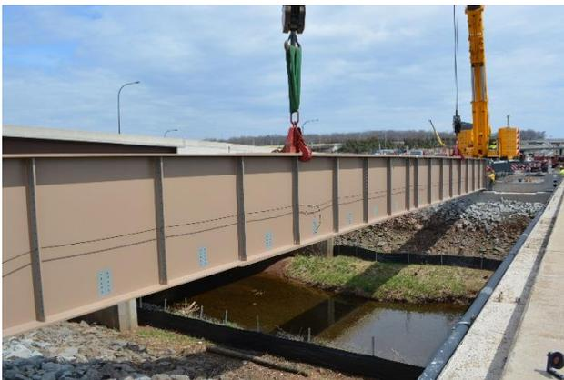
**Figure 11:** Girder erection over Horsepen Run.
