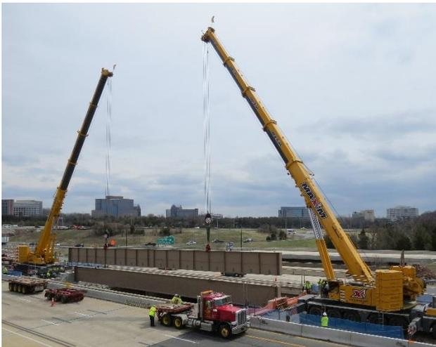
**Figure 10:** Girder delivery from adjacent bridge.
