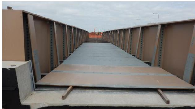
**Figure 12:** Placement of deck plates.
