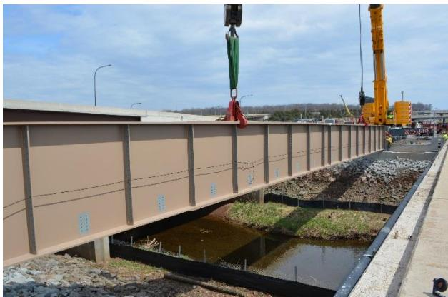
**Figure 11:** Girder erection over Horsepen Run.
