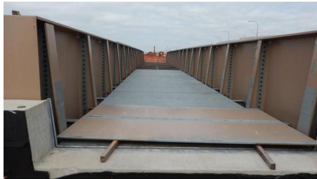
**Figure 12:** Placement of deck plates.
