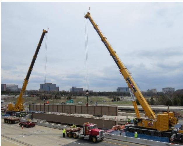
**Figure 10:** Girder delivery from adjacent bridge.
