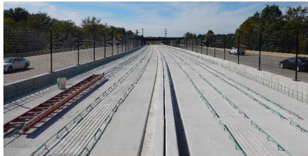
**Figure 17:** Finished concrete deck.
