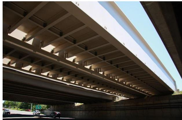
**Figure 7:** Completed steel framing.
