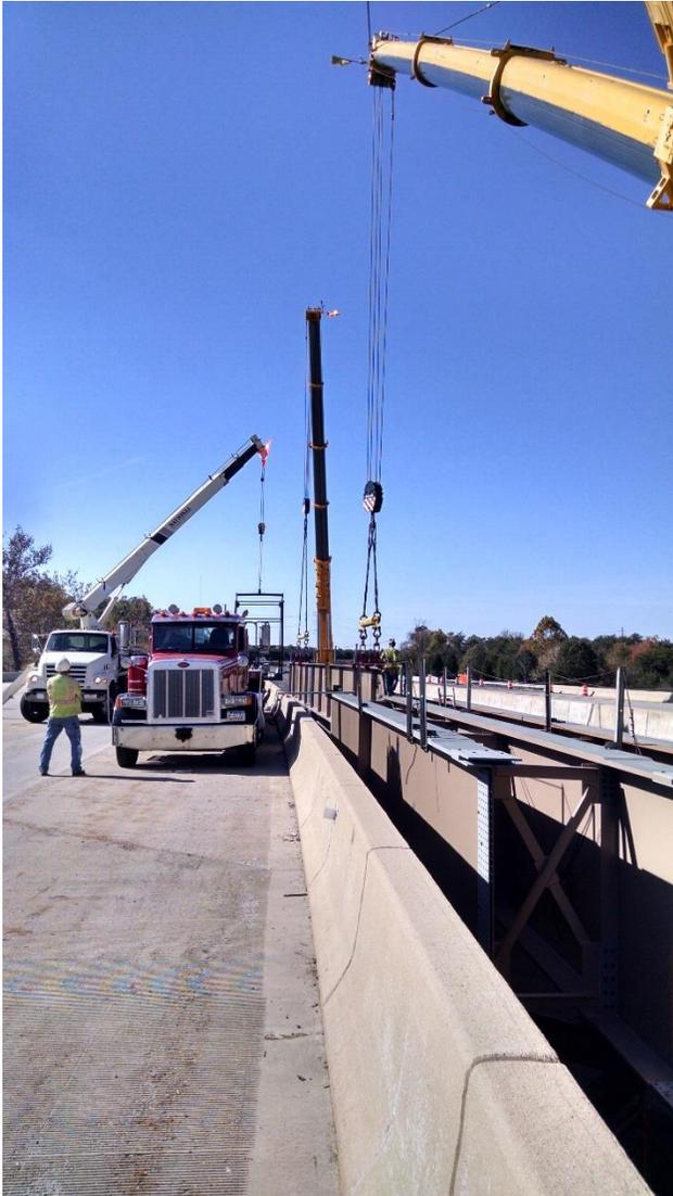
**Figure 16:** Broad Run girder erection.
