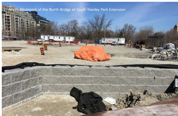
Figure 7. North Abutment of the North Bridge.
