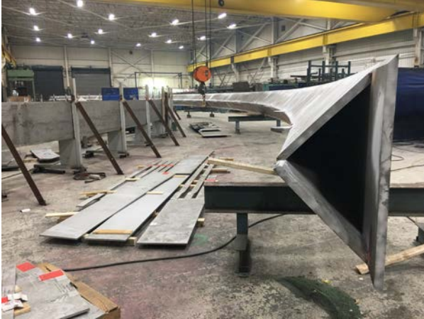
Figure 9. Steel fabrication of the arches..
