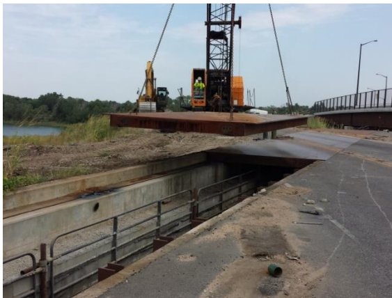
Figure 4: Steel span at the detour bridge
