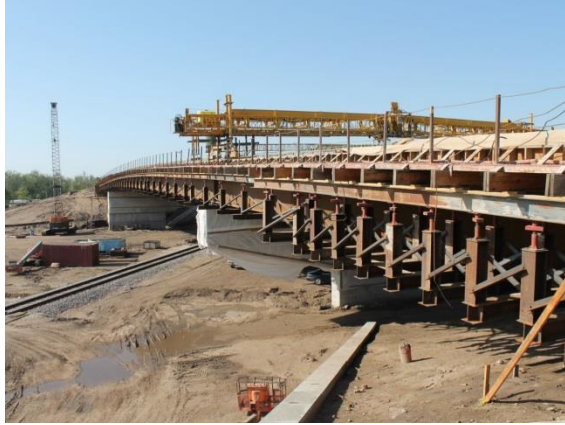
Figure 5: Extra length on needle beams
