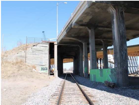
Figure 3: GRS wall with steel span
