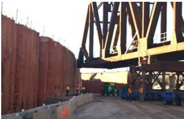
Figure 12: Truss being moved past the drilled shaft wall into south “pocket”.
