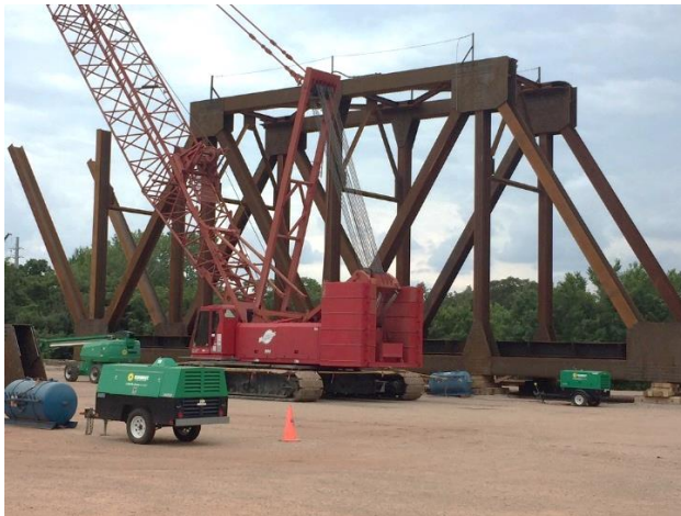
Figure 10: Truss erection from the center point with blocking at each panel point.
