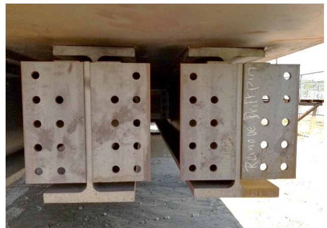
Figure 5: Flexibility in stringer connections.
