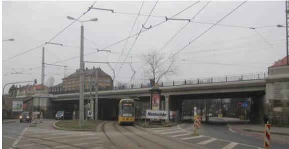
Figure 24: Example of Filler Beam with monolithic connection to the intermediate pier [16]
