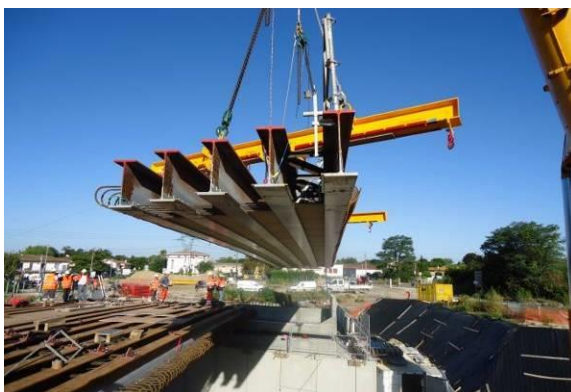
Figure 18: Lifting of beam packages on bridge supports
