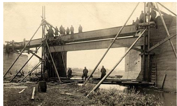
Figure 3: First filler beam bridge with 1m tall beam (HEB1000), Fentange, Germany 1917.
