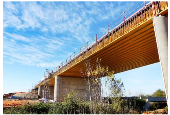
Figure 20: Filler beam deck during construction phase
