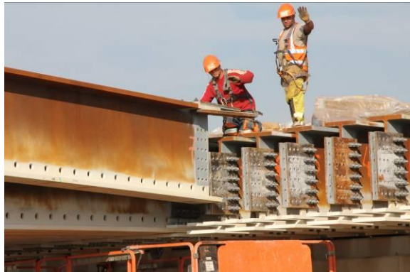
Figure 22: Installing of filler beam girder with bolted connection splice
