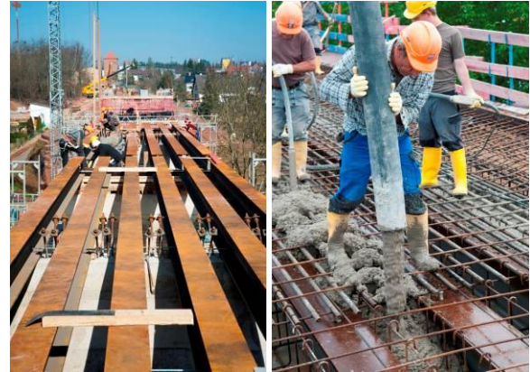
Figure 19: Filler beam deck concreting
