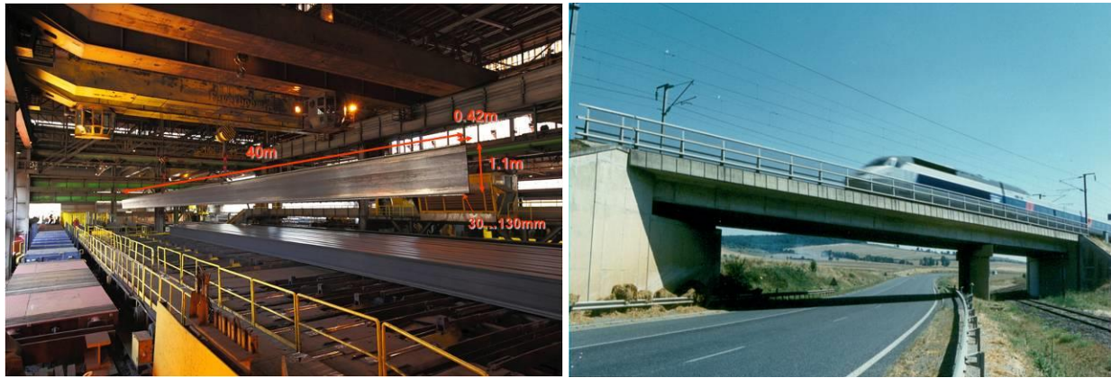
Figure 1: Left: view of rolled section at the rolling mill; Right: view of steel-concrete composite deck with rolled girders – East LGV line Paris- Strasbourg, RN3 overpass at Pomponne
