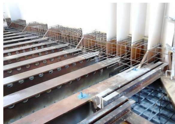
Figure 26: Cross girders for Half-through decks with lateral girders
