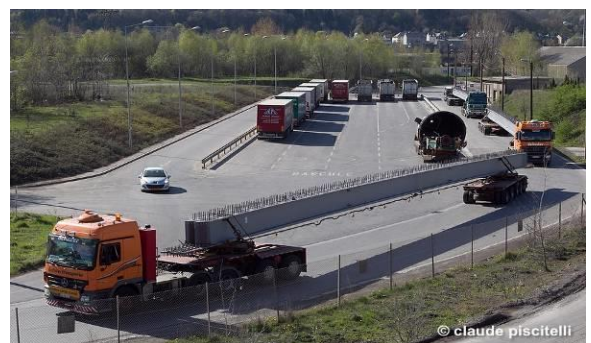
Figure 16: Exceptional road transport of 42.5m beams, roadway Bridge B6N in Magdeburg, 2011, Germany.
