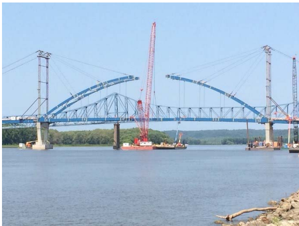
Figure 8 – Cantilever Arch Erection
