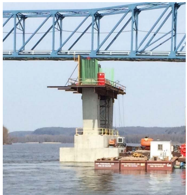
Figure 9 – Completed Waterline Footing
