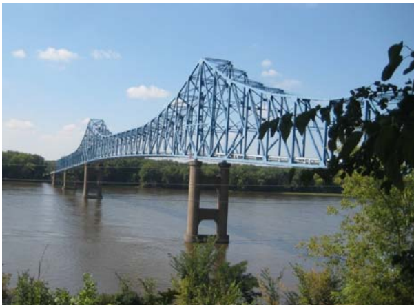
Figure 2 – Old Bridge Truss Spans
