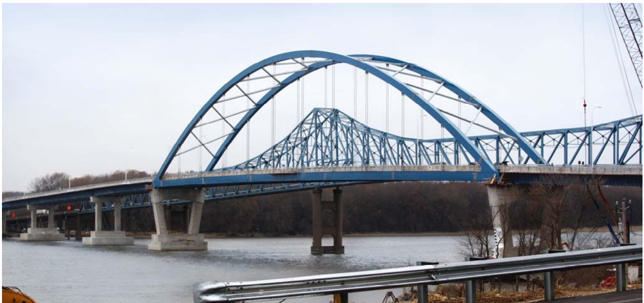
Figure 1 – New Arch Bridge
