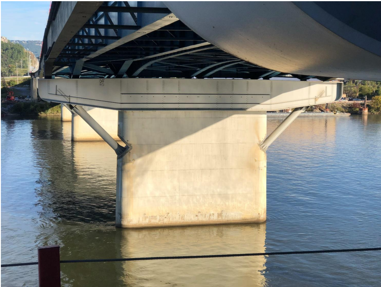
Figure 14 – Completed struts at pier 10
