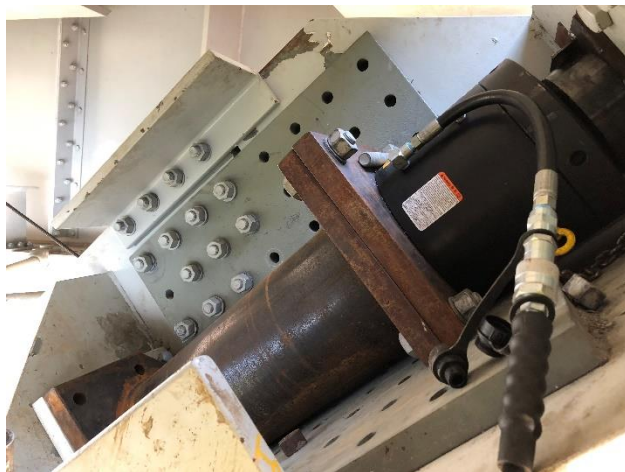
Figure 12 – Splice plate and jack in one quadrant of the cruciform
