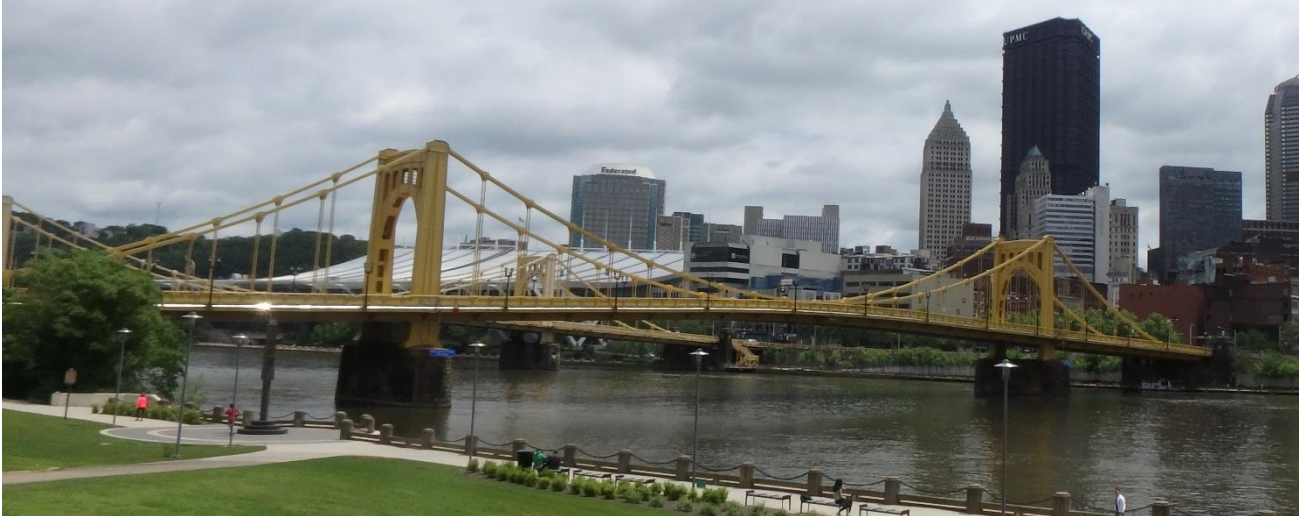
Figure 2: Elevation of the Andy Warhol Bridge (Looking Southeast Toward Downtown Pittsburgh)
