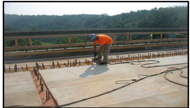
Figure 13: Providing two-way Composite Action
