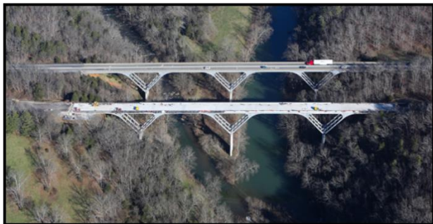
Figure 2: Bridge Aerial View
