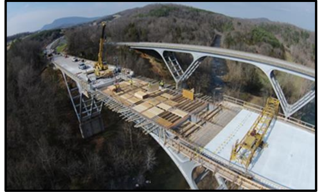
Figure 12: Deck Staged Construction
