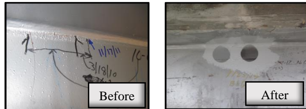
Figure 19: Fatigue Repair (type 6) at Web/Flange Weld
