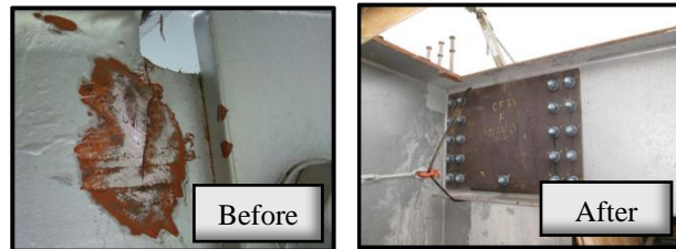
Figure 18: Fatigue Repair (type 5) at Floorbeam Coping
