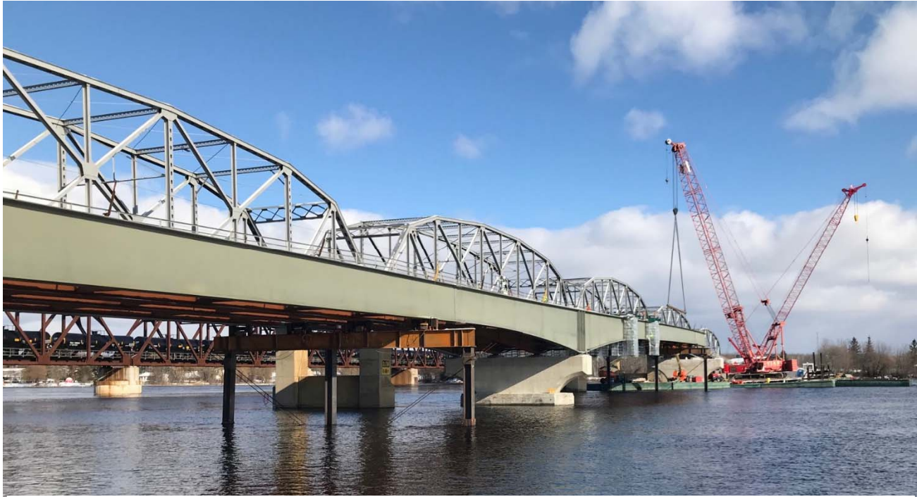
Figure 13: Girder Erection to Pier 3, Looking East
