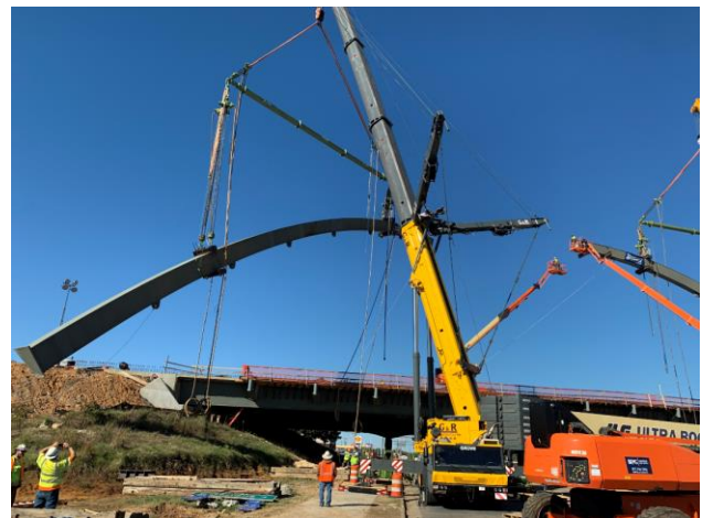
Figure 10: Swing Arch Sections 1 and 2 Into Position
