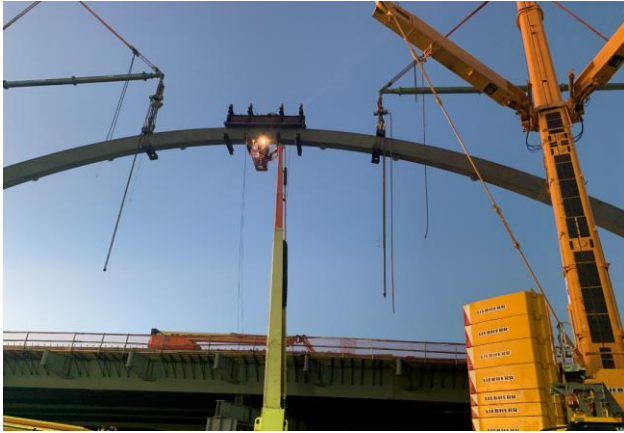
Figure 12: Strong Back in Position as Field Welding Begins
