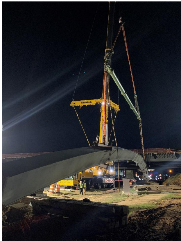
Figure 8: Rotating Arch Section 3 and 4 from Its Side to a Vertical Position
