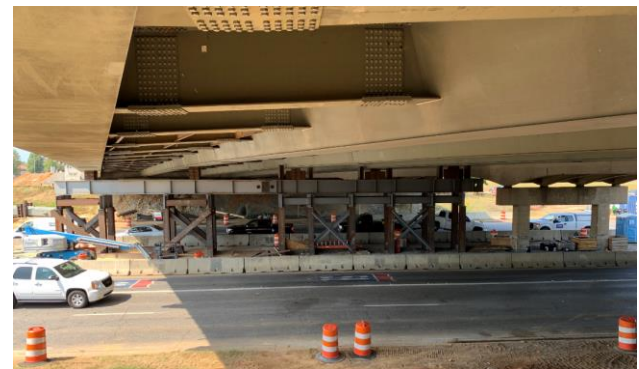
Figure 5: Installed Temporary Bent
