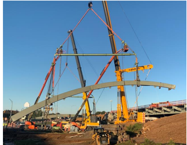
Figure 9: Raising the Arch Tip of Sections 3 and 4 to the Required Elevation by Modifying Sling Lengths with Air Hoists
