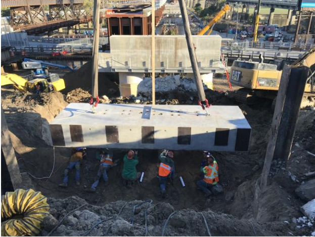
Figure 1: Welding of Abutment Cap to H-Piles During the Phase 1 Changeout
