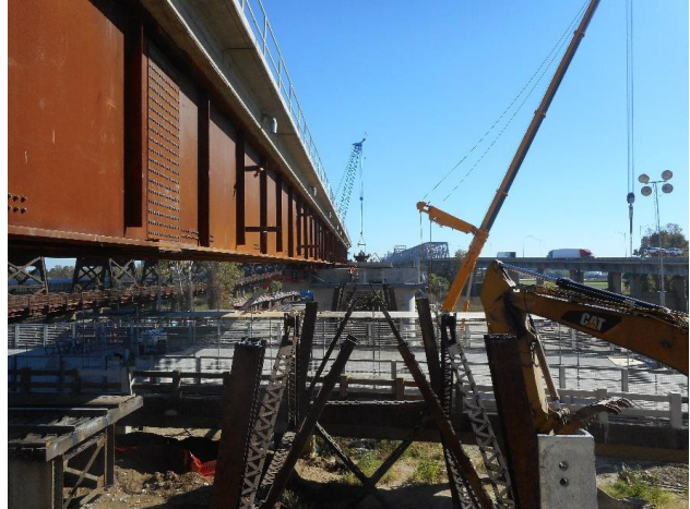
Figure 4: 176-6" Span Roll-Ins During the Phase I Changeout
