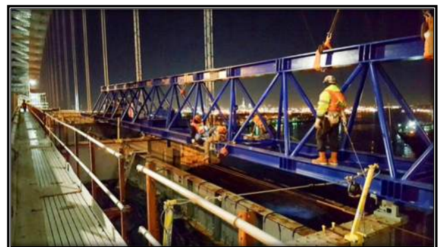
Figure 11 – Transfer Truss at PP20
