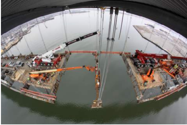
Figure 19 – Crane about to Remove First Floorbeam at PP20
