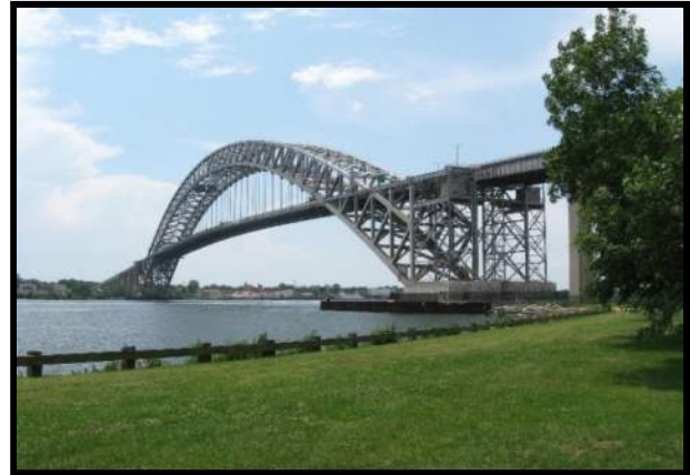
Figure 2 – Existing Bayonne Bridge Main Span
