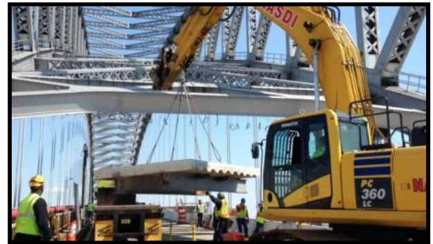
Figure 6 – Deck Demolition Operations
