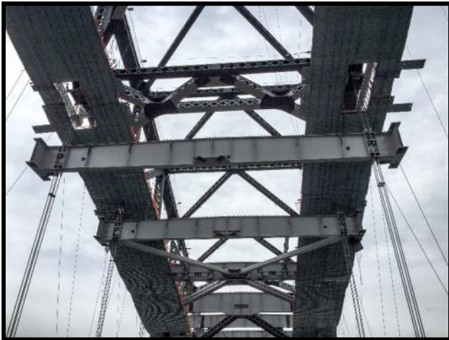
Figure 15 –PP11 and 12 with Permanent and Temporary Suspenders
