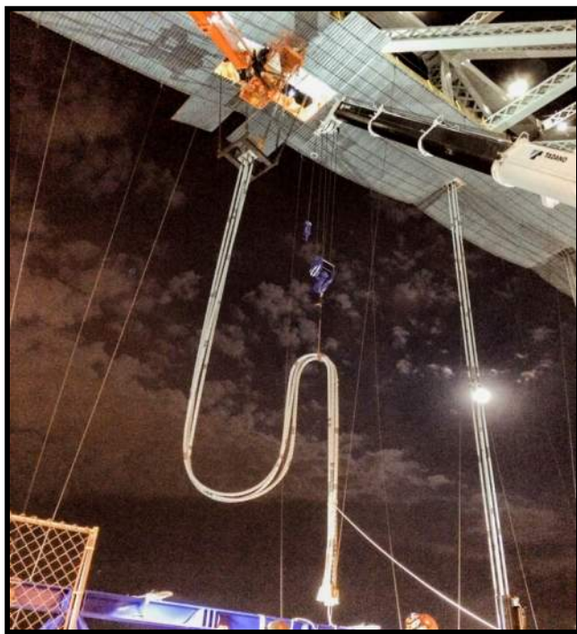
Figure 12 – Existing Suspender Removal
