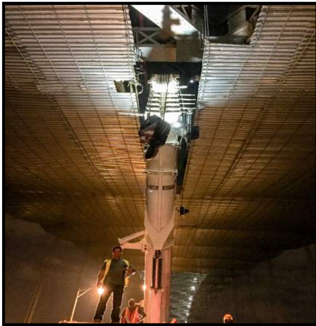
Figure 9 – Opening in Safe Span Shield with Crane Boom
