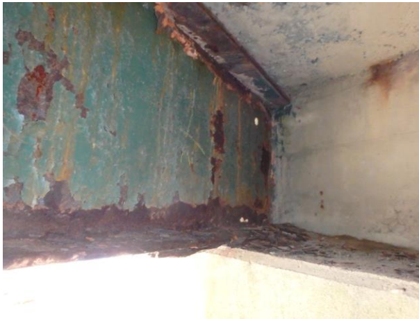
Figure 5: In-service condition of a girder in Bridge B.
