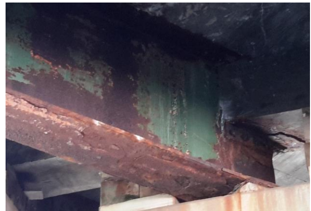
Figure 4: In-service configuration of Bridge A.
