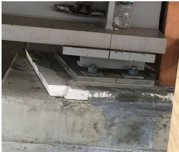
Figure 9: Disk Bearing Installation on the LaGuardia Project.
