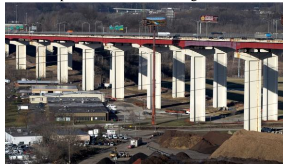
Figure 5: Existing Valley View Bridge
