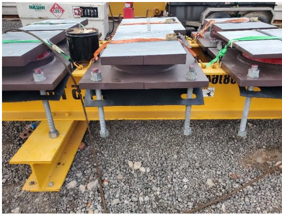
Figure 6: Disk Bearings ready for installation on the Valley View Jobsite
