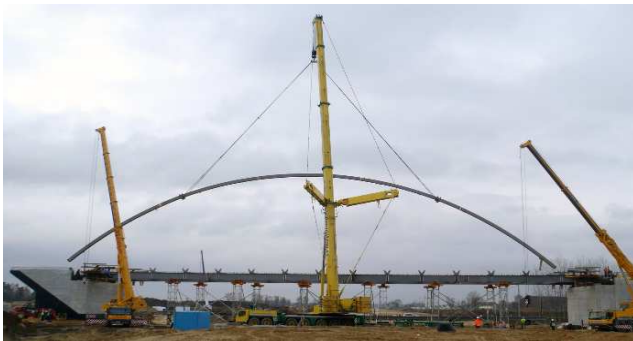
Figure 39: Erection of pre-assembled arch for WD-57
