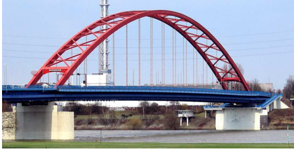
Figure 3: "Brücke der Solidarität" in Duisburg, Germany (1950), span 256m, with a Langer hanger arrangement [46].
