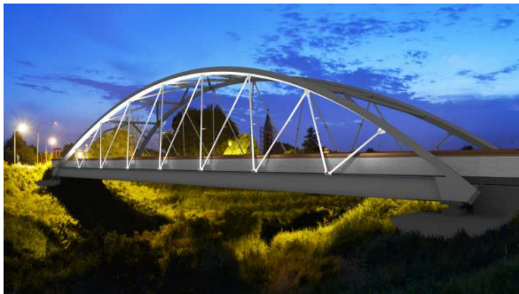
Figure 4: The new bridge over Panaro in Bomporto and Ravarino (Modena), (2018), span 80m, with a Nielsen hanger arrangement [42].
