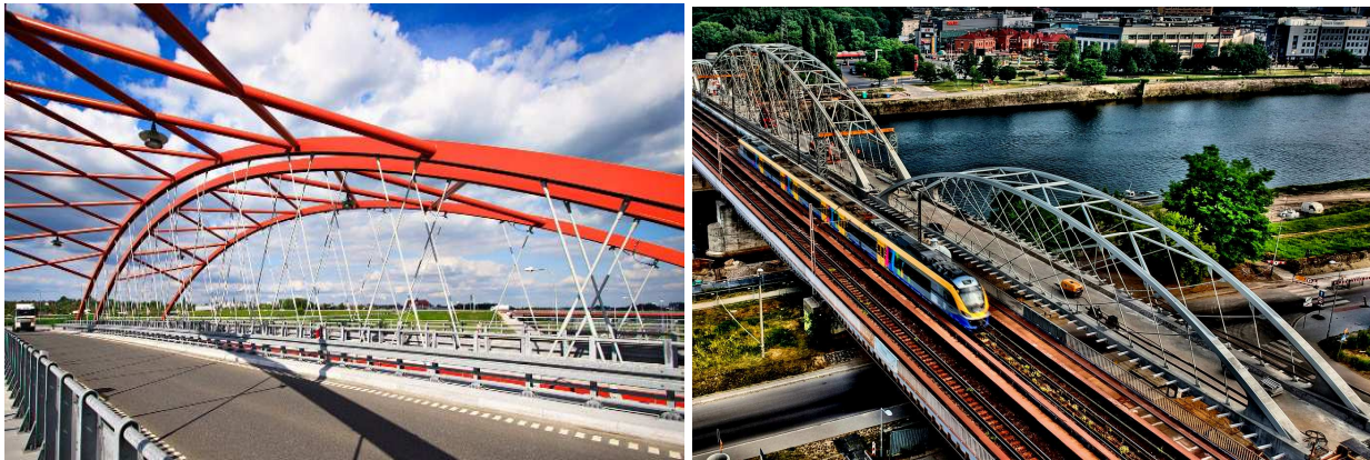
Figure 1: Left: Road bridge WD-431 over Highway A1 (Pyrzowice – Piekary) – span 62 m [32]; Right: Rail bridge E-30 over Vistola River in Krakow – main span 116m [39]
