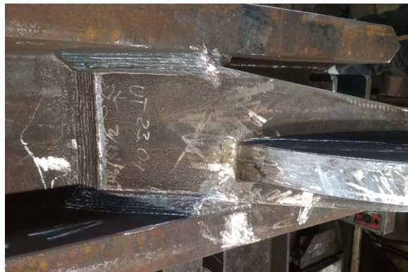
Figure 37: Details of Hanger attachment to the arch during fabrication
