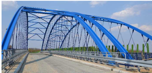
Figure 35: Bridge WD-137 over Highway A4 (Tarnów Rzeszów) – span 72 m.
