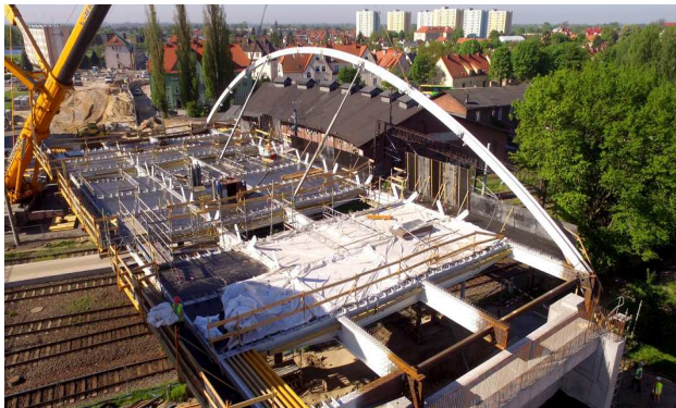
Figure 40: Erection of pre-assembled arch Bridge Zatorze in Elblag – Span 50m
