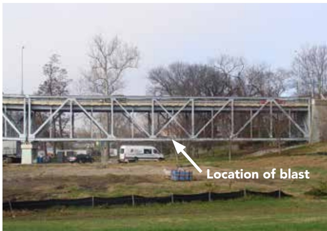
Fig. 1-3. Approach span of Milton Madison Bridge tested for redundancy.
