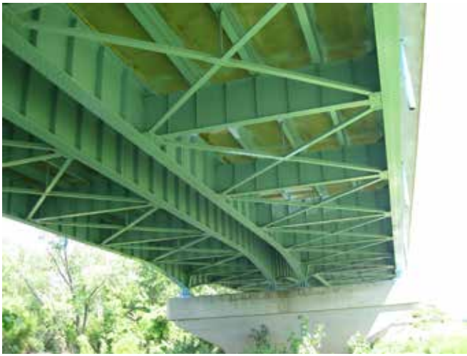
Fig. 4-6. Photo of the underside of the twin, two-girder bridges.
