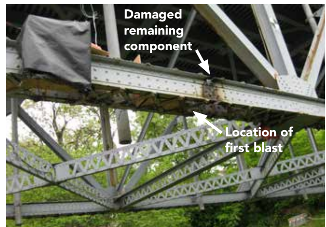
Fig. 1-4. Partially severed FCM, Milton Madison Bridge approach span.
