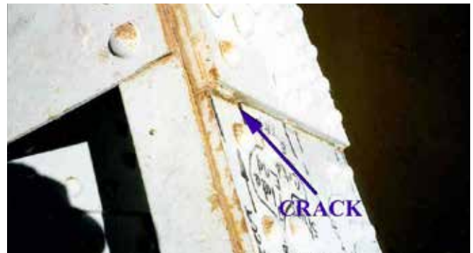
Fig. 1-2. Fractured tie girder plate, Hastings Bridge (Niemann, 1999).
