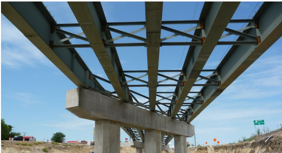
Figure 1-2, Example of Cross-Frames (TxDOT)
