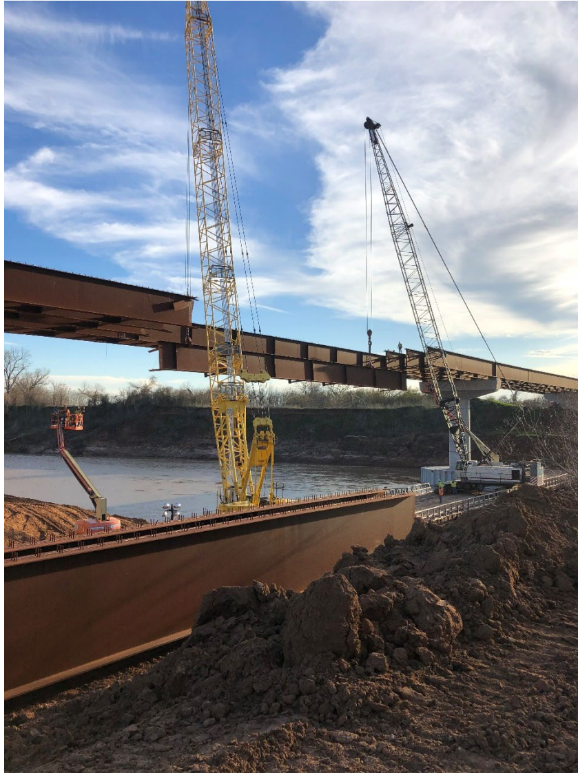
Figure 3-1, Erection of Drop-in Girder (TxDOT)
