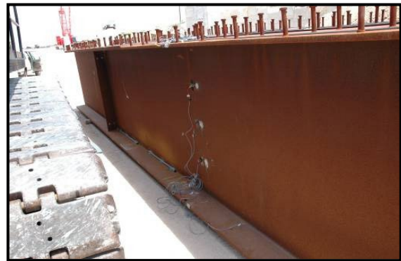
Figure 4-5, Girder Instrumentation (Helwig)
