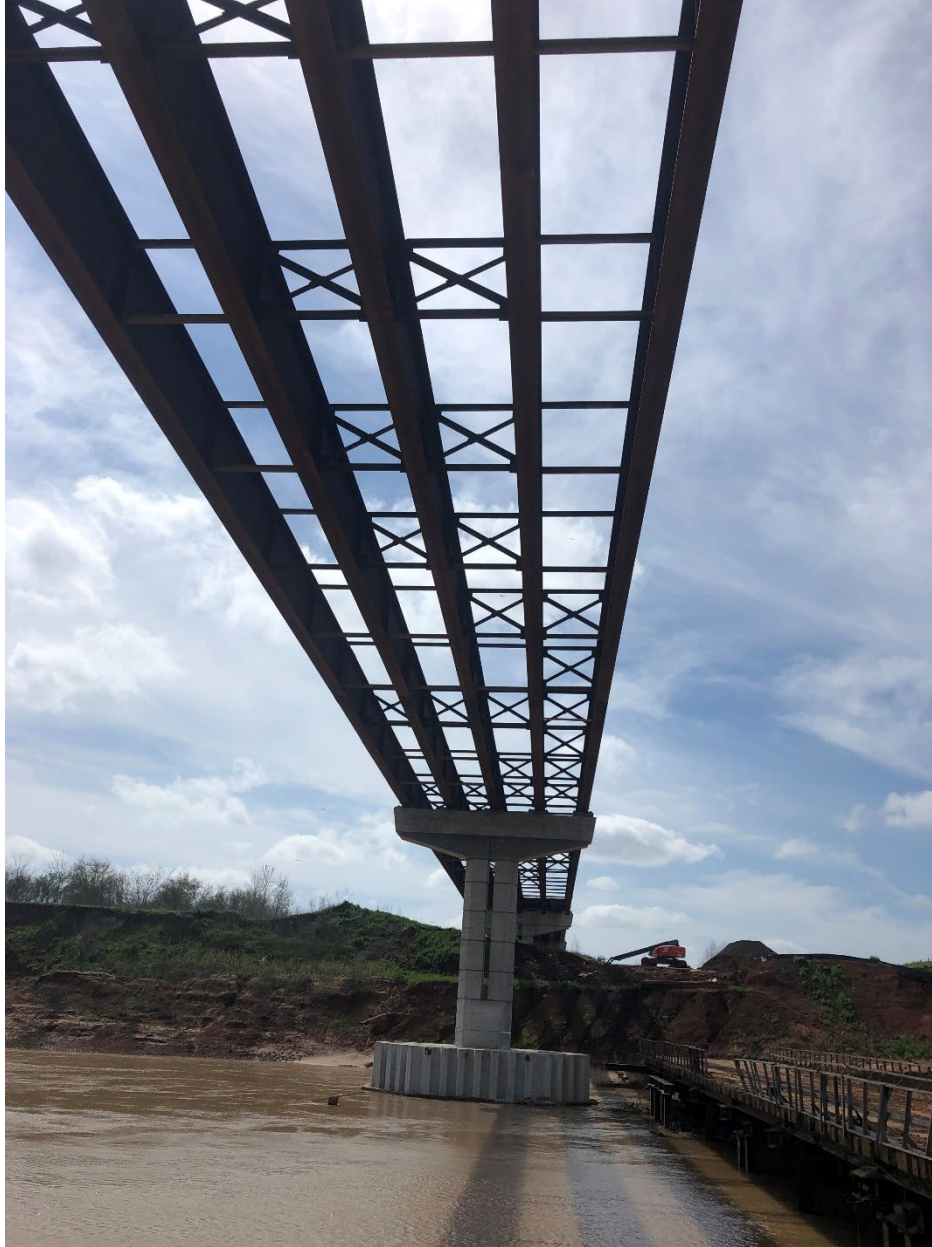
Figure 4-16, Completion of Steel Erection (TxDOT)
