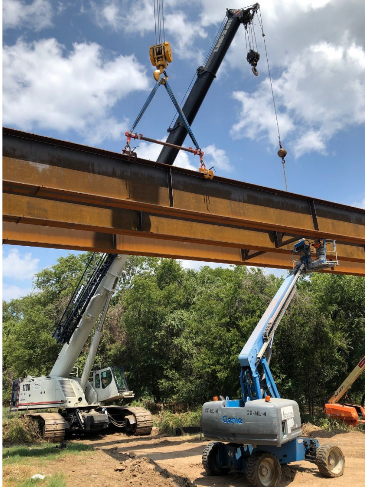
Figure 3-3, Partial Cross-frame Installation (Modjeski and Masters)
