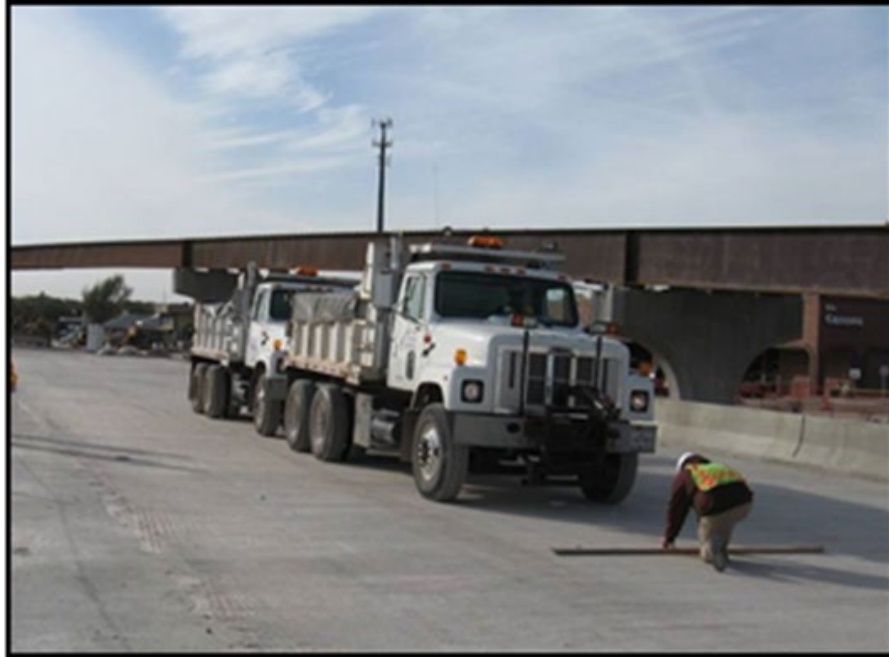
Figure 4-7, End-to-End Live Load Test (Helwig)
