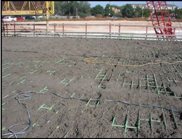
Figure 4-4, Pre-loaded Portion of Span 2 (Romage-Chambers)
