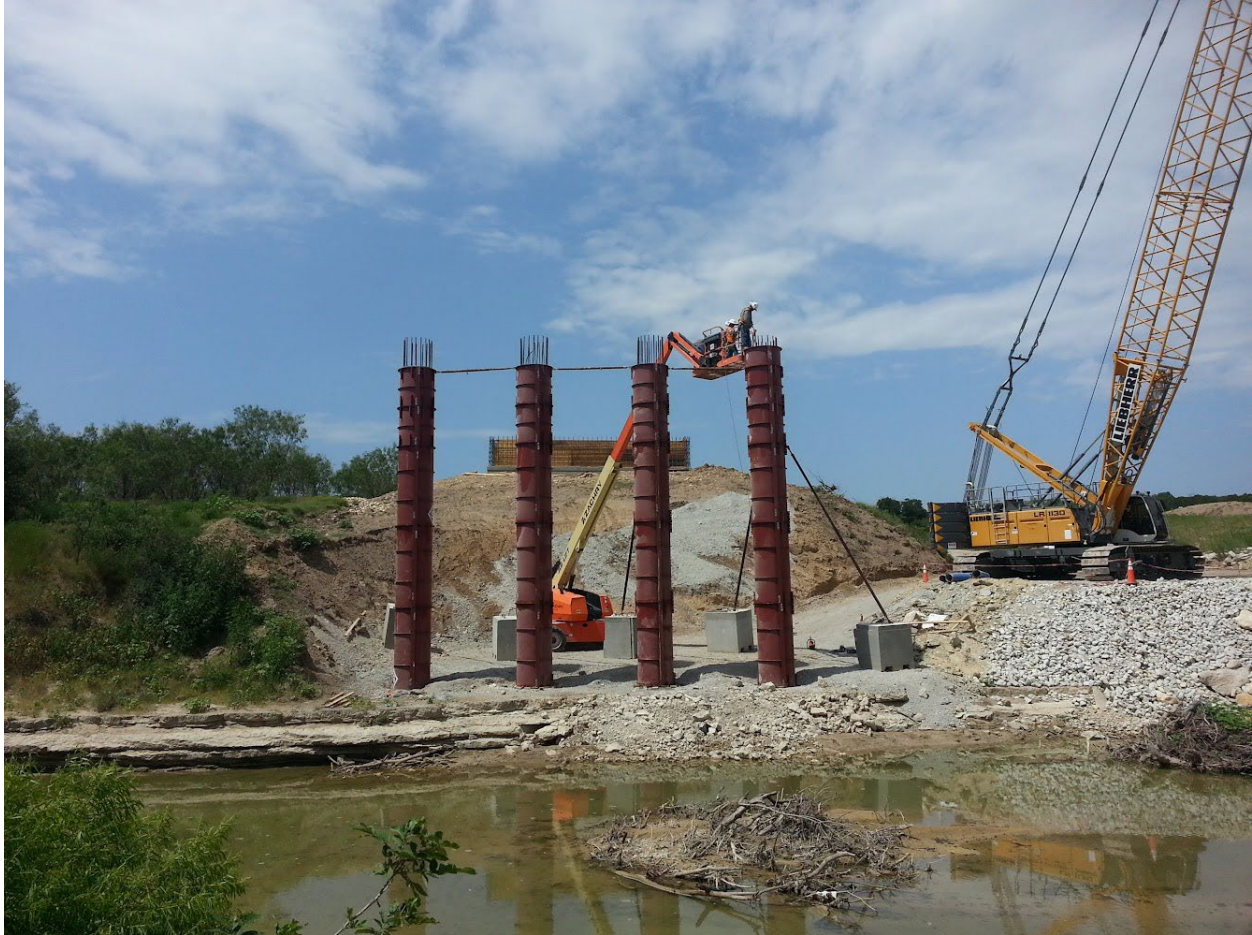
Figure 1-3, Lean-On Bracing Used for Column Formwork (Zachry Construction Corporation)
