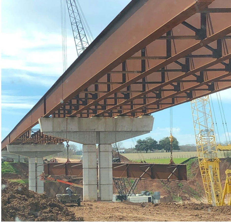
Figure 4-15, Drop-In Girder Section with Cross-Frames and Lean-On Braces Attached (TxDOT)
