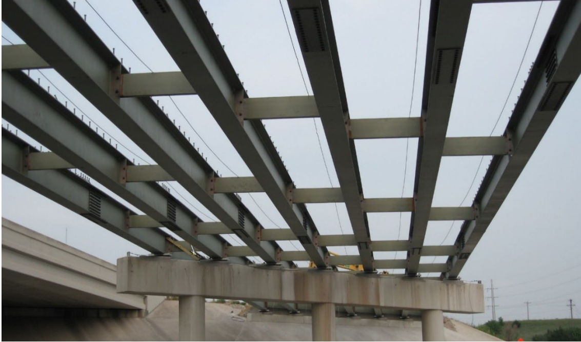
Figure 1-1, Example of Diaphragms (Modjeski and Masters)
