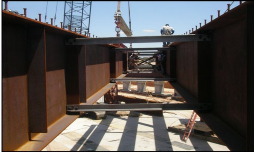
Figure 4-2, Lean-on Brace Struts seen during erection (Romage-Chambers)
