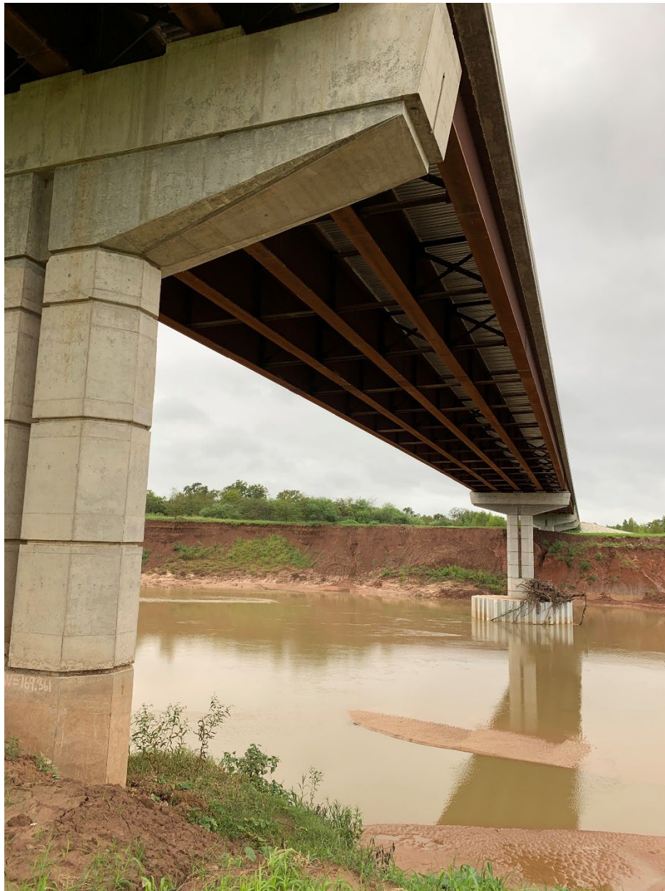
Figure 4-8, SH 155 at Brazos River Bridge (TxDOT)
