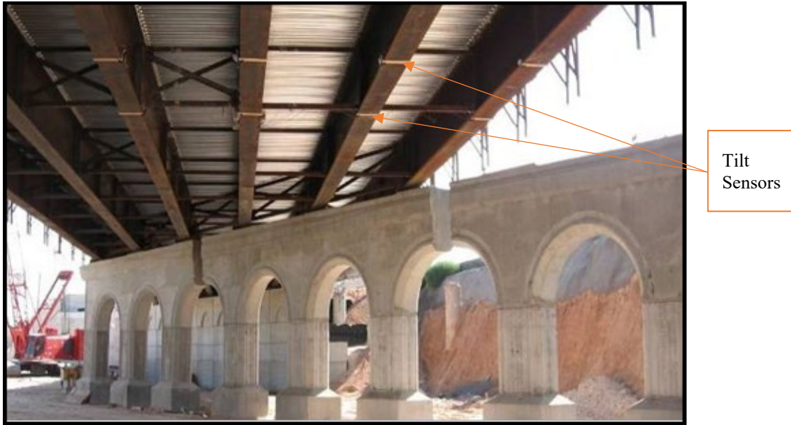
Figure 4-6, Tilt Sensors Installed on Bottom Flanges (Helwig)
