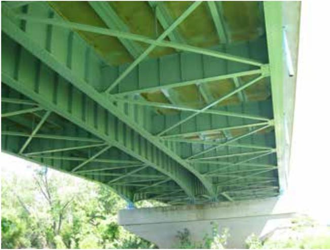
Fig. 4-6. Photo of the underside of the twin, two-girder bridges.
