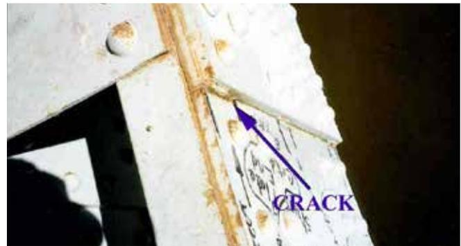
Fig. 1-2. Fractured tie girder plate, Hastings Bridge (Niemann, 1999).
