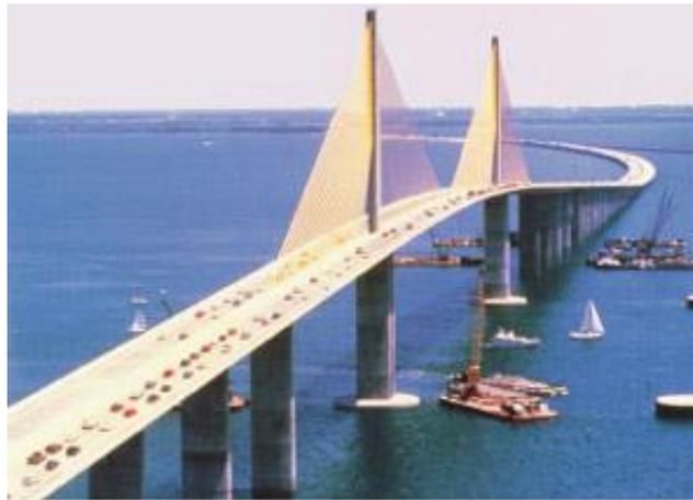
**Figure 15 Photo of a cable-stayed bridge with single column towers
