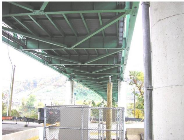
**Figure 8 Photo showing a typical stacked floor system**
