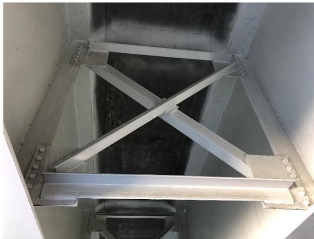
**Figure 1 Photo of a typical multi-girder system with x-type intermediate cross-frames**
