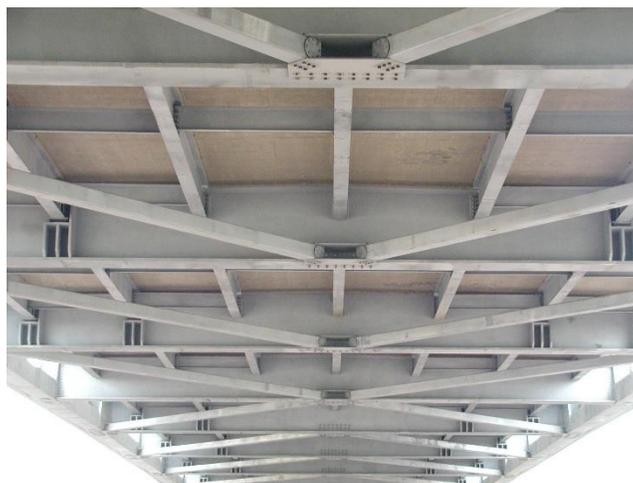
**Figure 9 Photo of a typical framed floor system**
