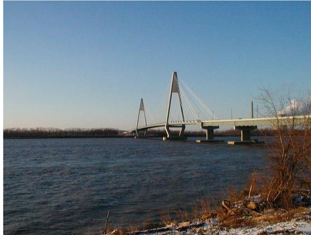
**Figure 13 Photo of a cable-stayed bridge with A-Towers
