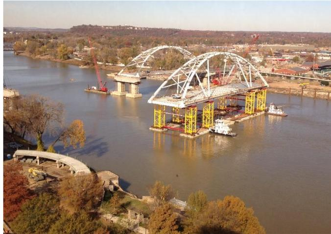
**Figure 18 Photo showing an arch being floated into place (Broadway Bridge over the Arkansas River near Little Rock Arkansas) (Credit: HNTB Corporation)**
