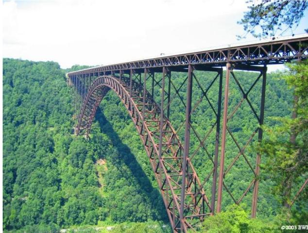
**Figure 10 Photo a steel deck arch bridge
