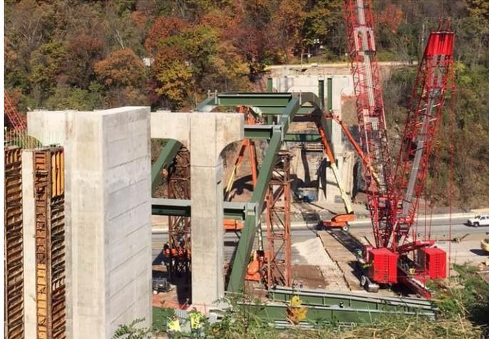
**Figure 19 Photo showing the erection of a deck arch (Greenfield Bridge over Interstate 376 near Pittsburgh, Pennsylvania) (Credit: HDR)**
