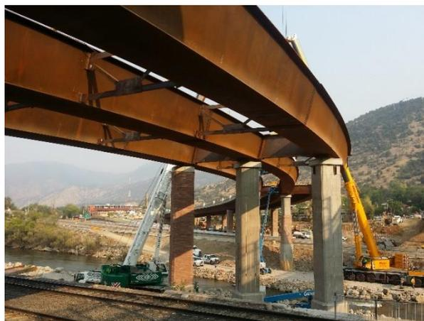
**Figure 3 Photo of a typical tub girder bridge under construction (Credit: RS&H)**
