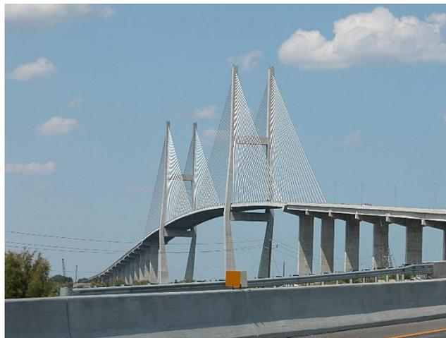
**Figure 12 Photo of a cable-stayed bridge with H-Towers
