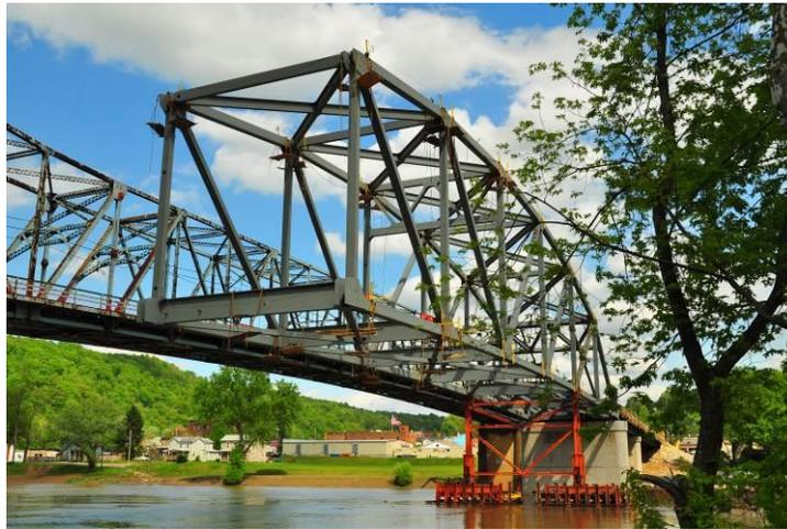
**Figure 17 Photo showing the cantilever erection of a truss (Point Marion Bridge over the Monongahela River in southwestern Pennsylvania) (Credit: HDR)**
