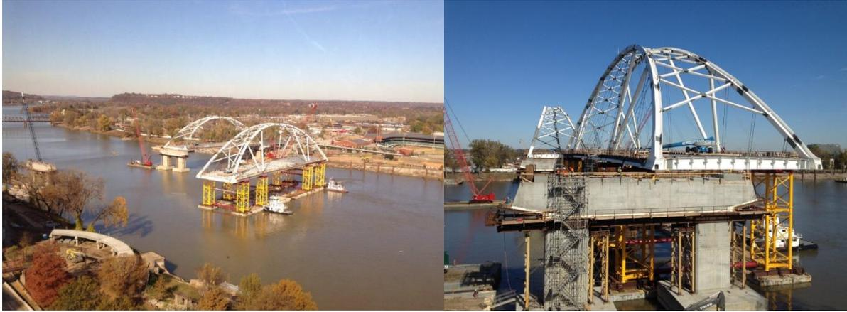
**Figure 19 Tied arch sliding laterally in place, by use of barges**
