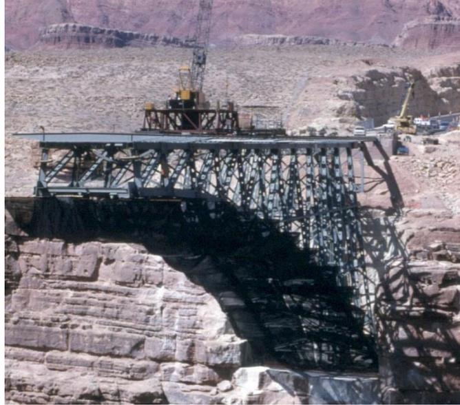
**Figure 16 Arch bridge erection using the floor system as an erection tie to the canyon wall**
