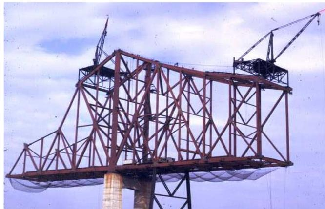
**Figure 14 Cantilever erection of a continuous truss using derricks**
