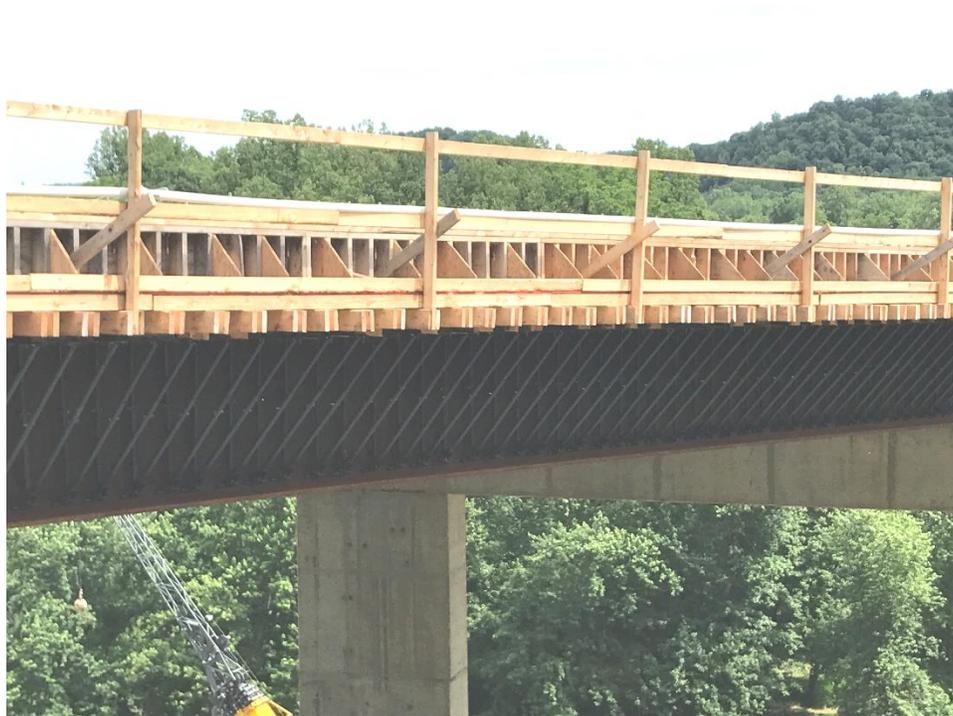
**Figure 21 Typical overhang brackets**
