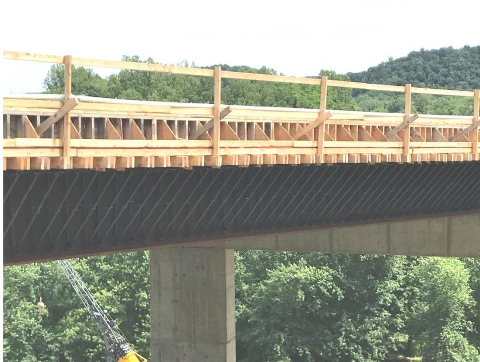
**Figure 21 Typical overhang brackets**
