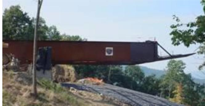
**Figure 11 I-girder bridge launching**
