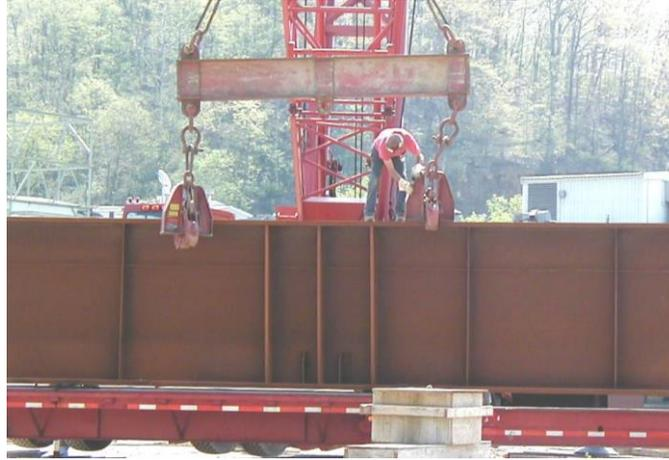
**Figure 9 Use of a spreader beam for I-girder erection**
