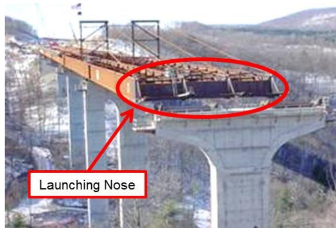
**Figure 12 I-girder launch with launching nose and cable tie-backs**
