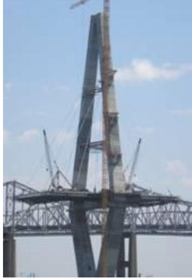
**Figure 17 Cantilever cable stayed bridge erection using deck mounted derricks**
