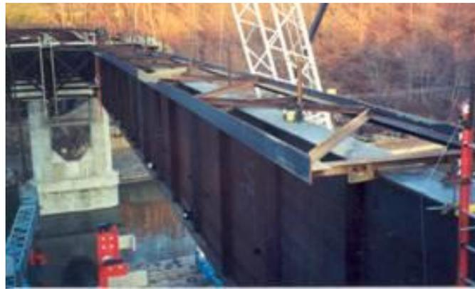
**Figure 25 Temporary top flange stiffening truss**
