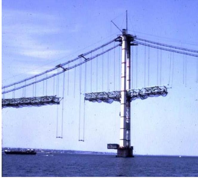
**Figure 18 Suspension bridge erection using cable travelers**
