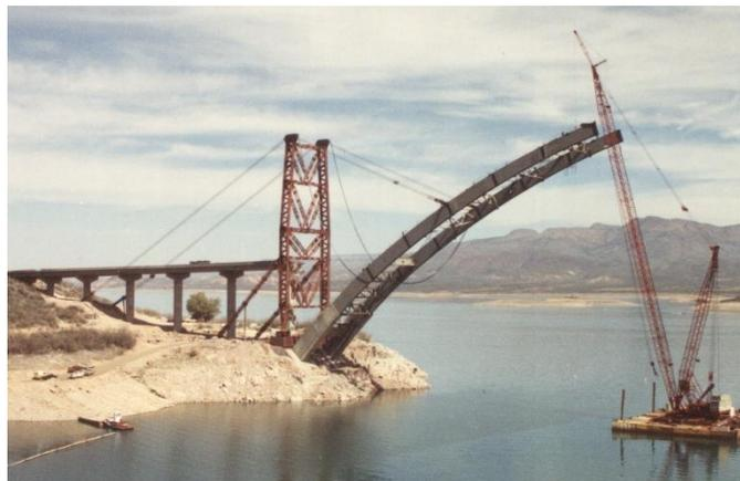
**Figure 15 Arch erection using stay towers and cables**
