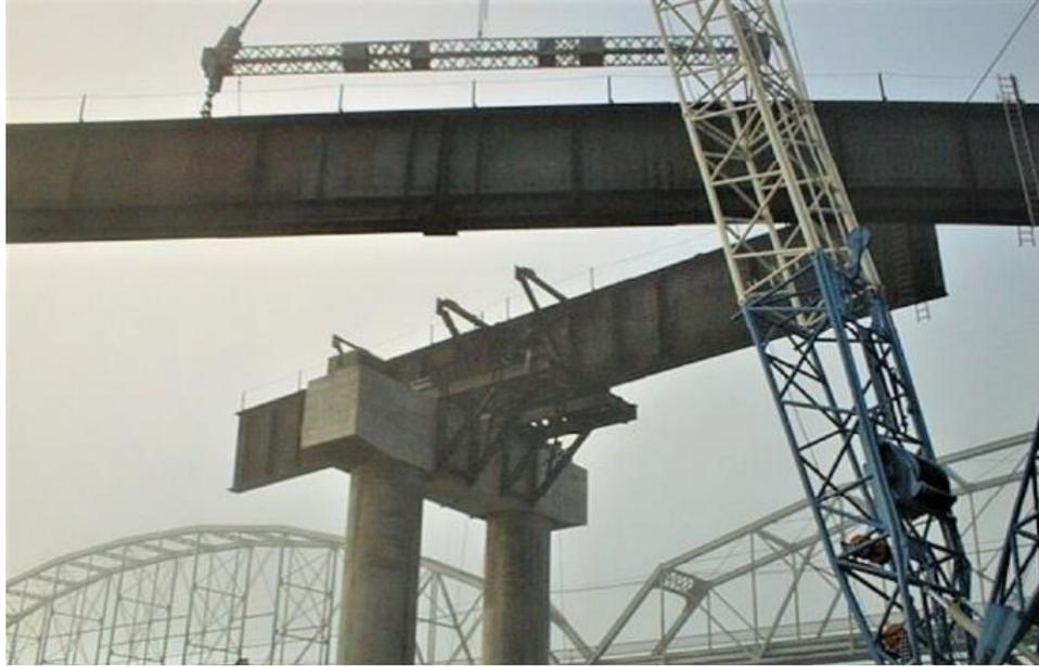
**Figure 8 Pier brackets in an I-girder bridge**
