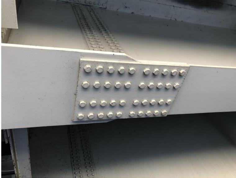
**Figure 2 Photograph of a Steel Plate I-Girder Bolted Field Splice at a Flange Width Transition**
