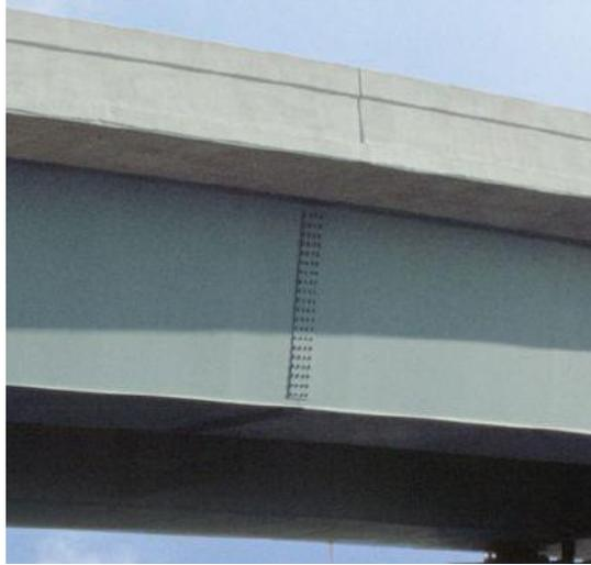
**Figure 10 Photograph of a Box Girder Field Splice**
