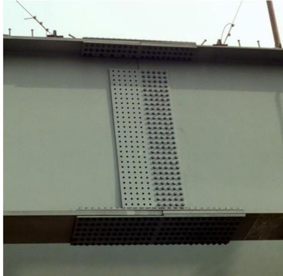
**Figure 6 Photograph of a Field Splice for a Long Simple Span Steel I-Girder**
