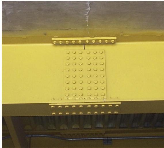
**Figure 9 Photograph of a Rolled Beam Field Splice**
