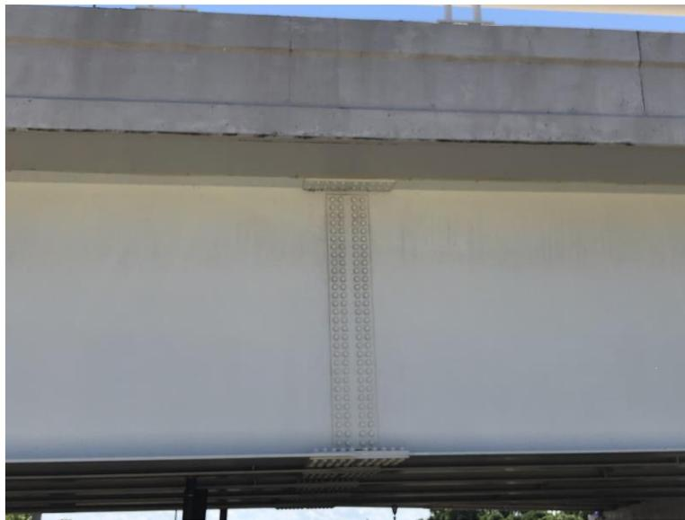
**Figure 1 Photograph of a Steel Plate I-Girder Field Splice**
