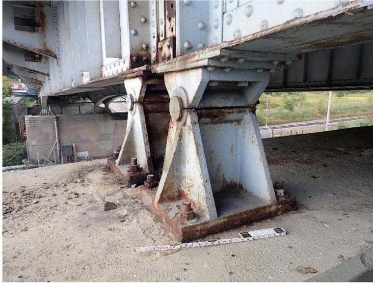
**Figure 4 Fixed Mechanical Bearing (courtesy HDR)**
