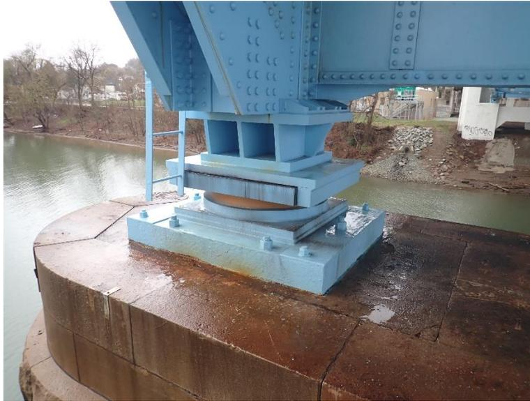
**Figure 2 Pot Bearing (courtesy HDR)**
