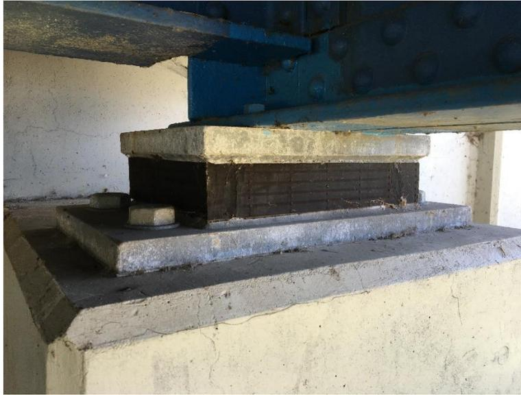
**Figure 1 Elastomeric Bearing (courtesy R. J. Watson)**
