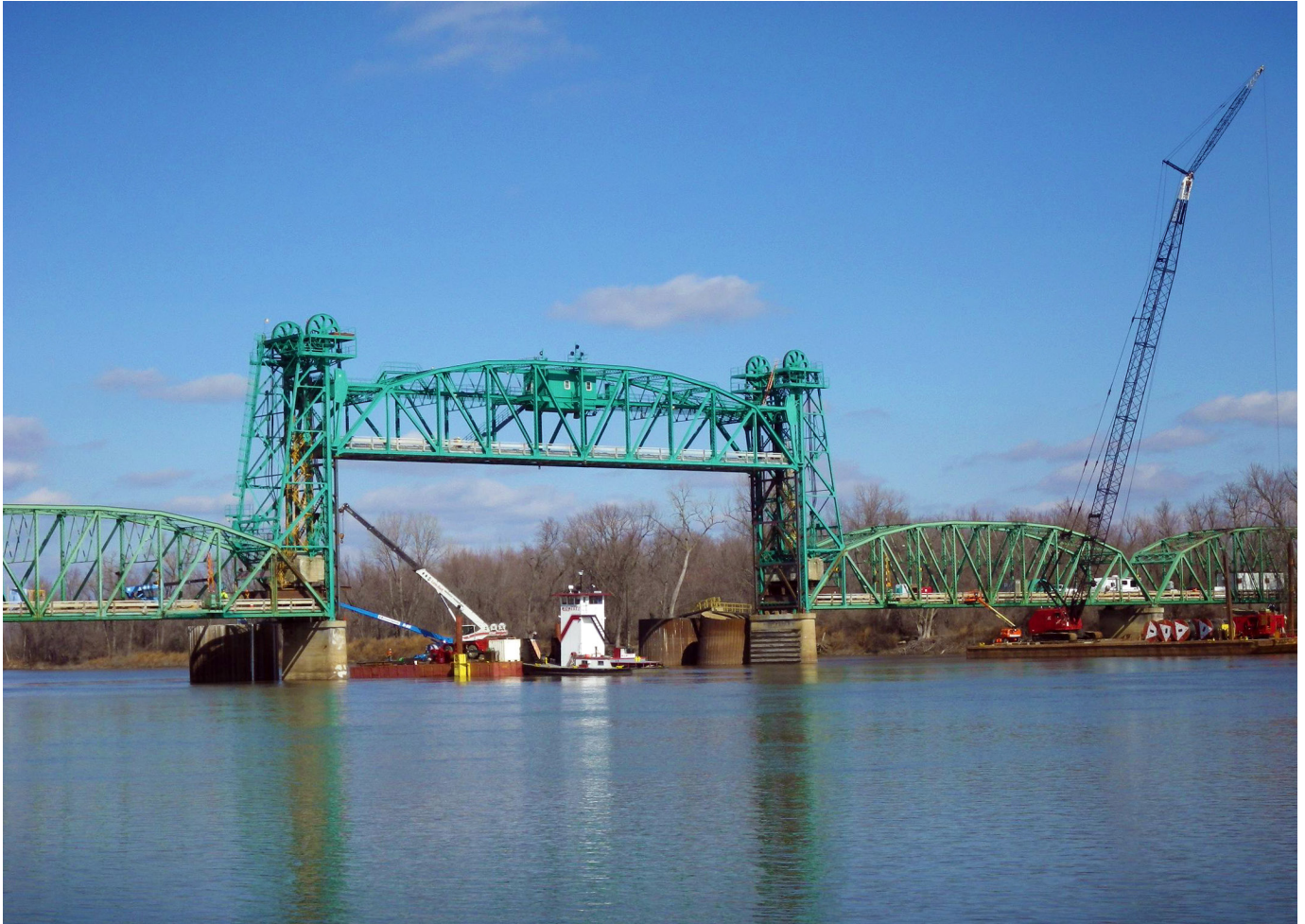
▲ The lift span was supported in the open position, thus allowing barge traffic to continue during the rehabilitation work.
