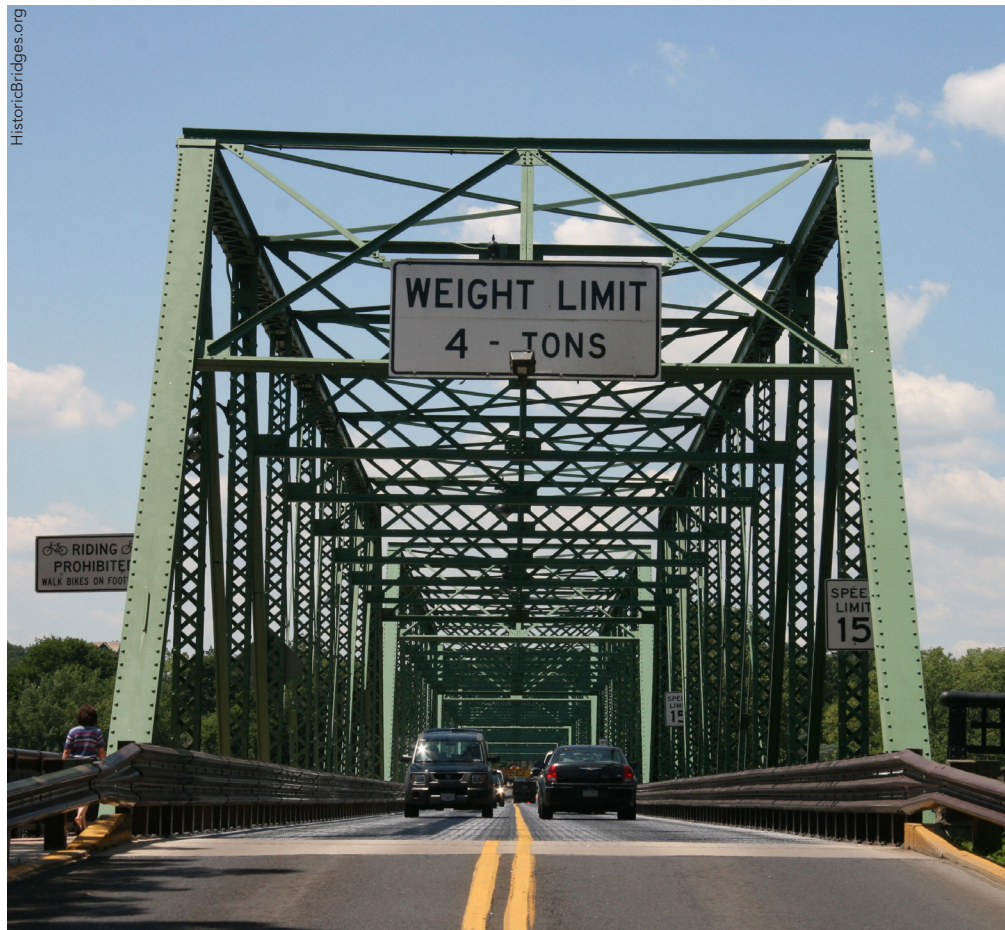
▲ The New Hope-Lambertville Bridge opened in 1904 and currently carries 14,000 vehicles across the Delaware River daily. Each of the bridge's six spans measures 171 ft, and the total length is about 1,050 ft. Vertical truss members measure 27 ft in height, and abutments date back to the original 1814 bridge.
