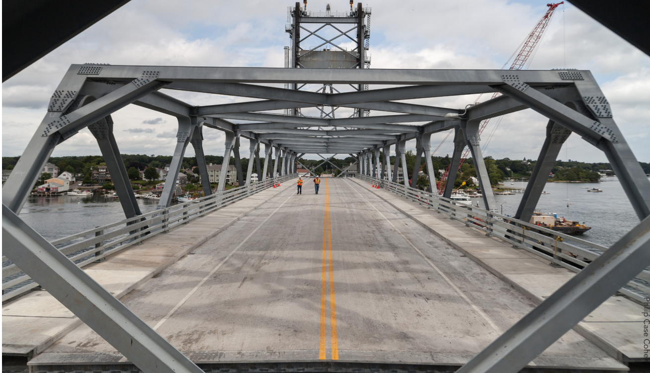
▲ The design features two 11-ft through lanes, two 5-ft shoulders for bicyclists, two 6-ft sidewalks and overlooks at both flanking spans.
