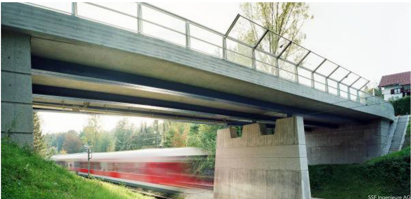
▼ Finished Pöcking Bridge.
