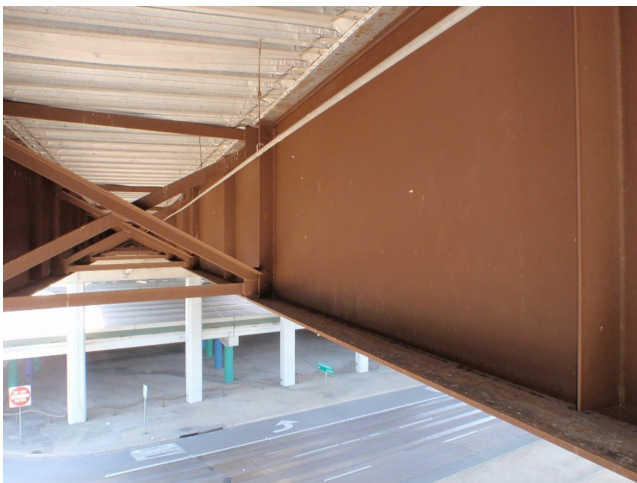
◀ Favorable performance of a UWS overpass.
