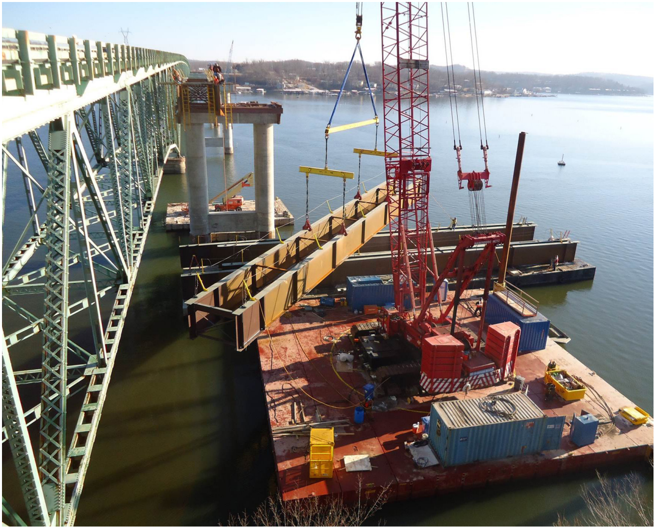
▲ The new structure comprises two plate girder units with six typical spans of 265 ft.
