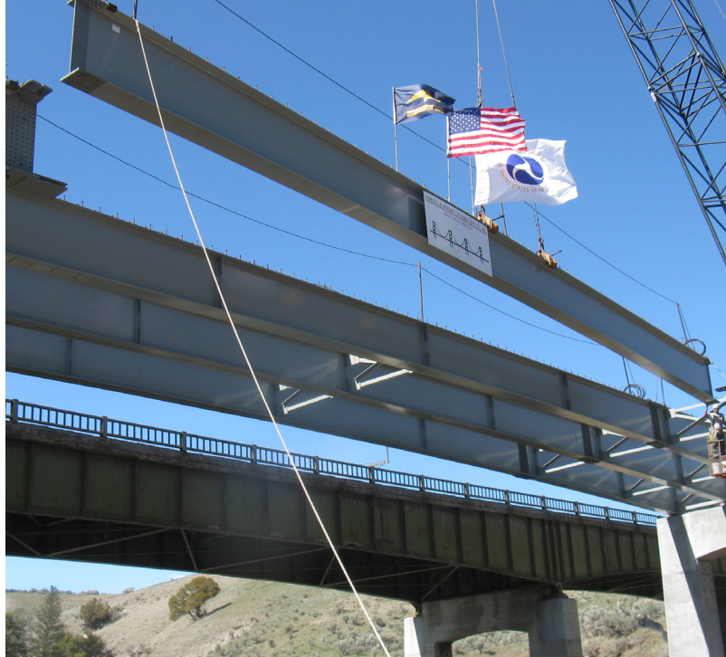
Setting the middle section of the last girder.
