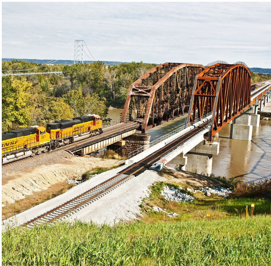
▲ High Steel provided 1,213 tons of fracture-critical steel for the railroad truss, while Capital Contractors provided 2,046 tons of plate girders for the approach spans.
