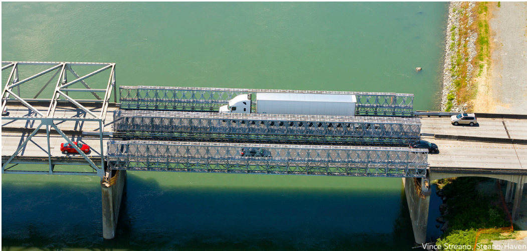
◀ Temporary spans were erected, and the bridge reopened only 23 days after the collapse.
