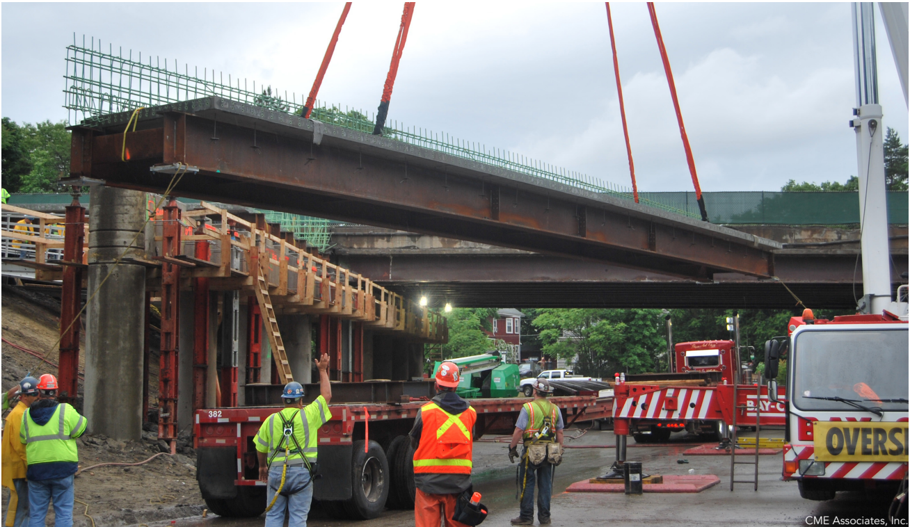
▲ The 93Fast14 Project in Medford, Mass., demonstrated the viability of modular steel bridge construction by replacing 41 spans in ten 55-hour weekend work periods.
