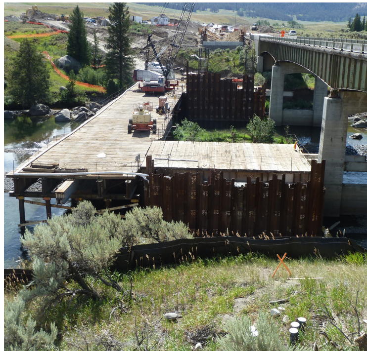
An independent platform was built to carry all construction equipment and materials across the river.
