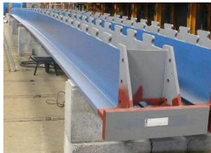
◀ Steel fabrication of the Pöcking Bridge.
