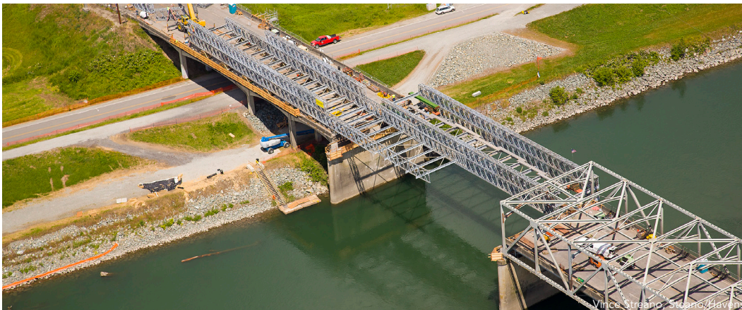
◀ Erection of the temporary spans.
