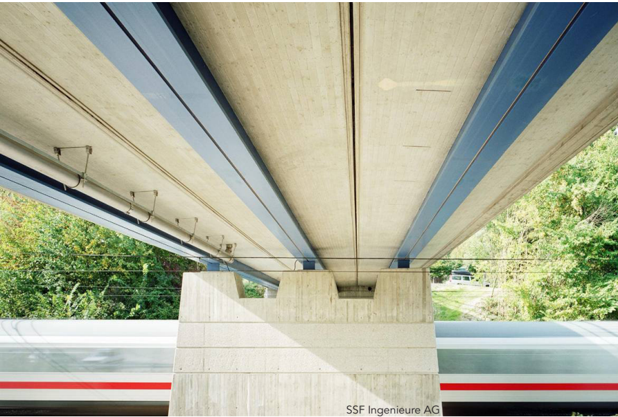
▲ View beneath the Pöcking Bridge (Germany) with Precobeam elements.
