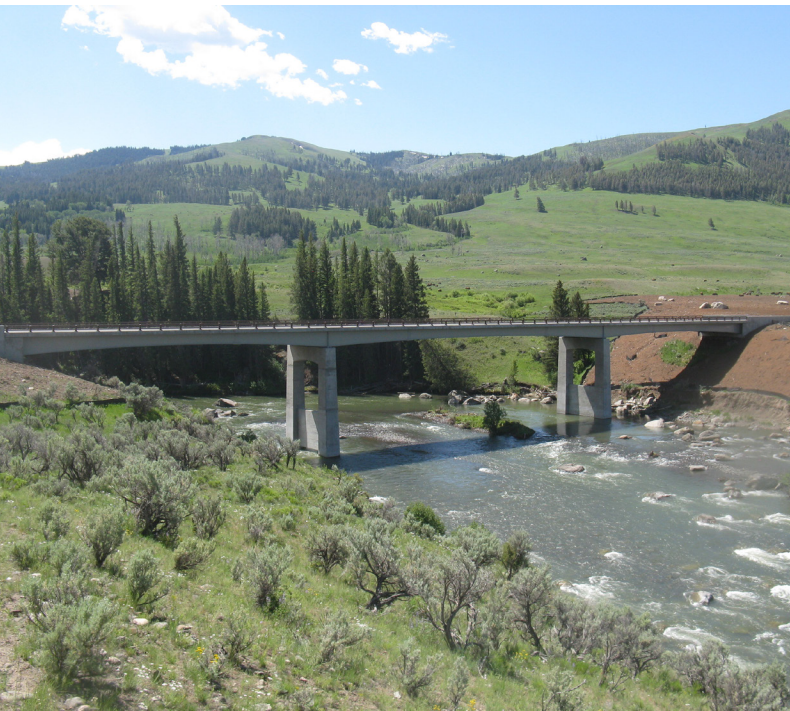
The new Lamar River Bridge is a two-lane, 420-ft-long, 33-ft, 4-in.-wide, three-span (127.5 ft-165 ft-127.5 ft) steel plate girder bridge.
