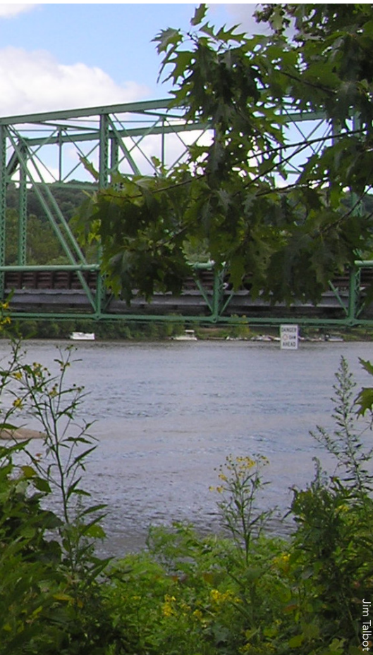
▲ The New Hope-Lambertville Bridge opened in 1904 and currently carries 14,000 vehicles across the Delaware River daily. Each of the bridge's six spans measures 171 ft, and the total length is about 1,050 ft. Vertical truss members measure 27 ft in height, and abutments date back to the original 1814 bridge.
