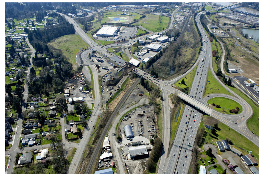
▲ An aerial view of the project site (looking southwest) shows the project with excavation underway prior to pushing the new bridge into place.
