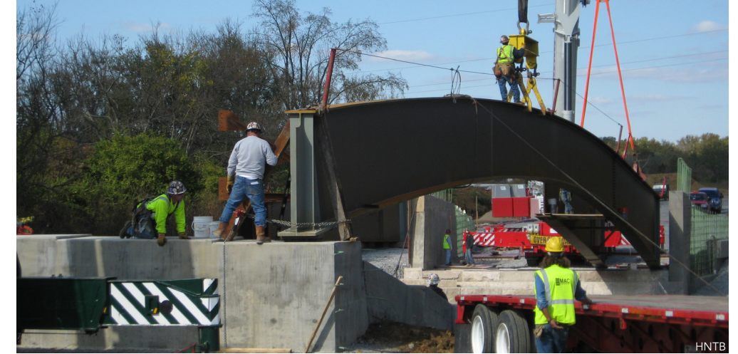
▼ The bridges are inspired by the arc of a deer leaping over a fence. ▲ The staging and laydown area was limited, but the contractor was able to place cranes next to the rear of the abutments and hoist the field sections out over the river. ▼ Crossframe drawings for the Thornton Bridge.
