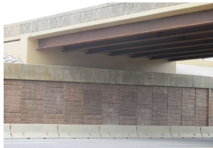
▲ Mechanically stabilized earth (MSE) walls were constructed in front of the abutments in order to minimize the span lengths, yet still provide for future Interstate widening.
