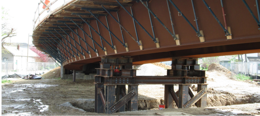
◀ The 60-in.-deep box girders for the Jeffersonville approach had spans as long as 160.67 ft.
