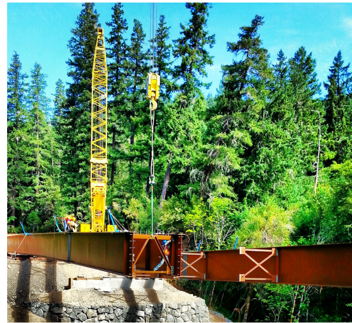
▲ The bridge consists of four 189-ft, 4-in. spliced girders, 7 ft deep, with a 110-ft long midsection and two 37-ft, 2-in. end sections.
