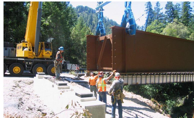
▼ Installing the new Hurdy Gurdy superstructure; the original bridge is visible just below the new steel.
