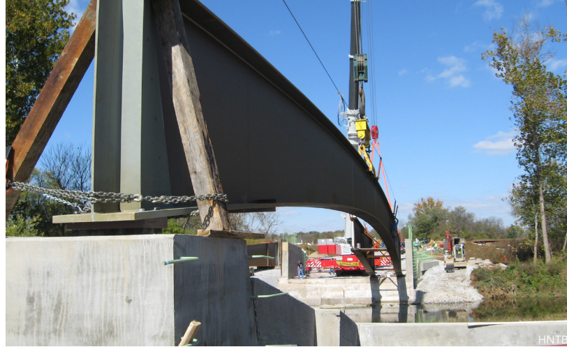
▲ The bridges are composed of haunched welded steel plate girders fabricated from M270 Grade 50W weathering steel. ▼ A model of one of the bridges.
