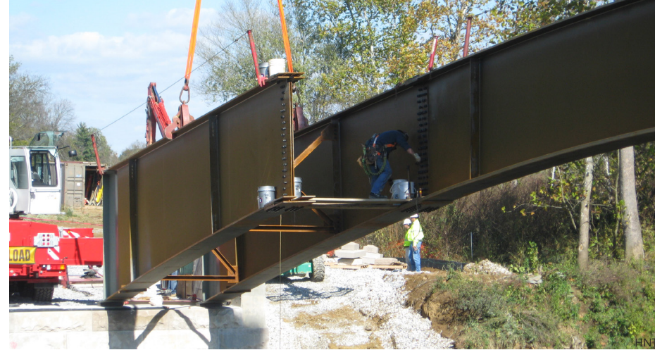
▲ A second girder following the first one.
