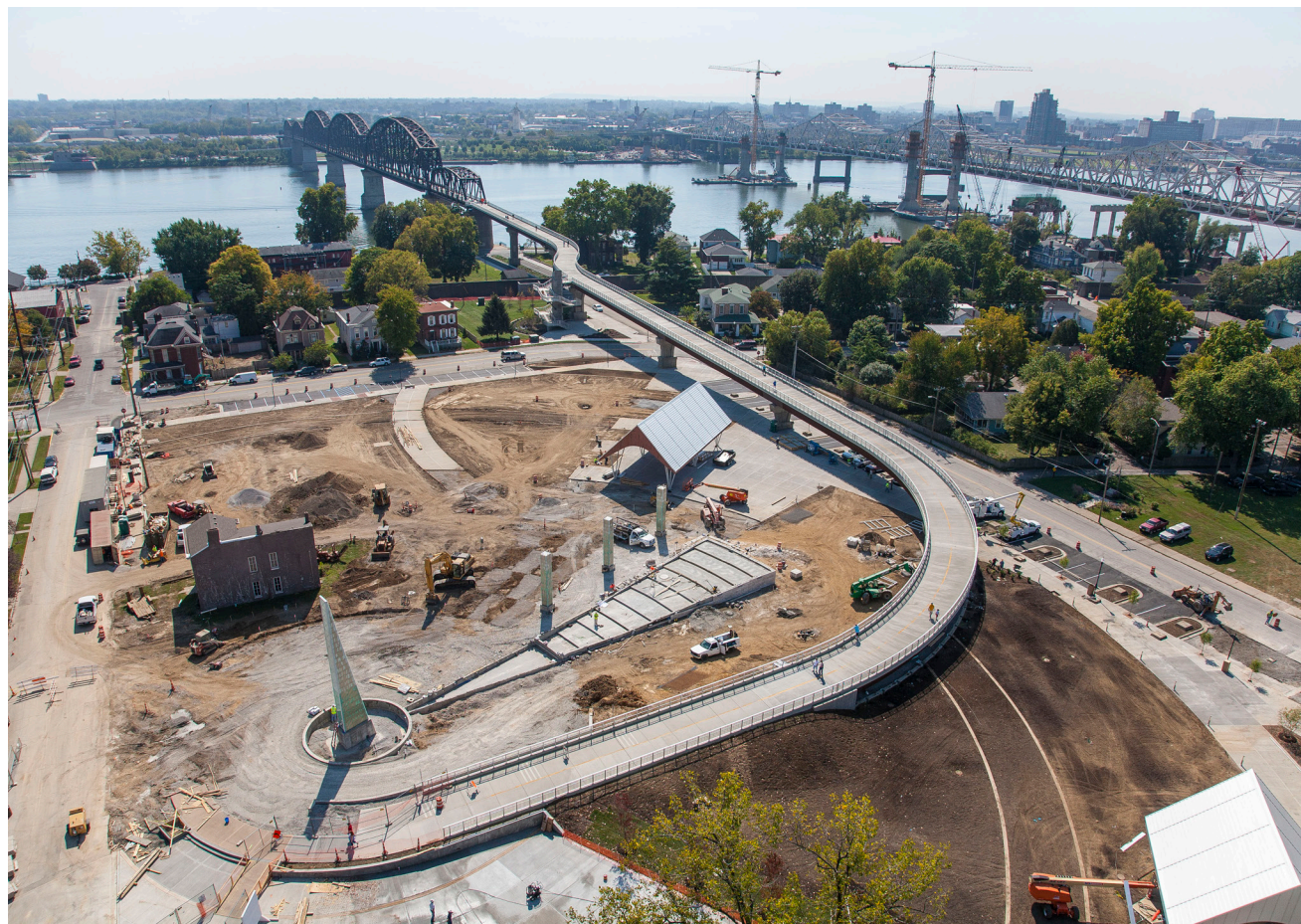
▲ ▼ While steel box girders are often used on curved long-span highway bridges for stability and structural efficiency, they are not generally used on pedestrian bridges. However, this girder type was chosen for the Jeffersonville approach because the girder fascia and bottom soffit create a streamlined look through the S-curve span and the sharp 90° curve at the end of the bridge.
