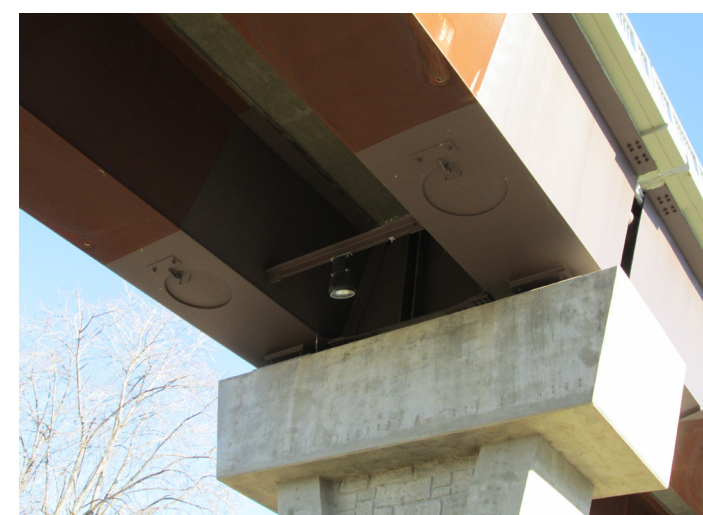
◀ ▼ The portions of the girders immediately above the piers are painted to prevent staining caused by runoff from the weathering steel as it develops its patina.
