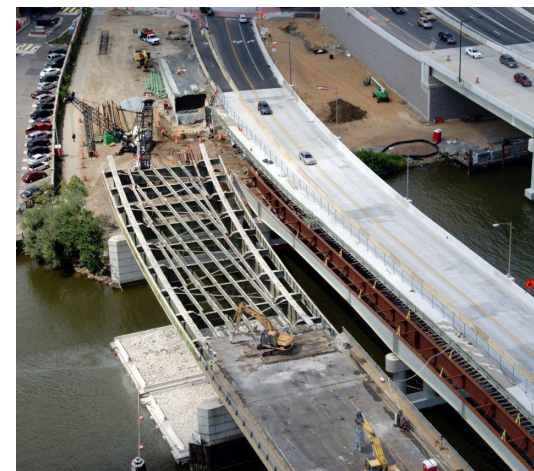
Stage 2 framing and closure bay with an upward load on G1 (jack stand) and downward load on G1 (concrete block).
