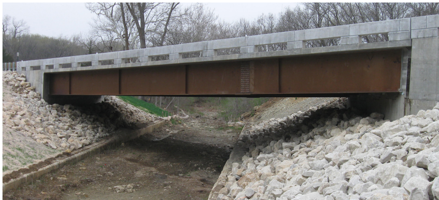
▼ The final girder layout of the new bridge was a single span of 112 ft, using five girders at a 9-ft spacing; the steel plate girders are made from weathering steel.
