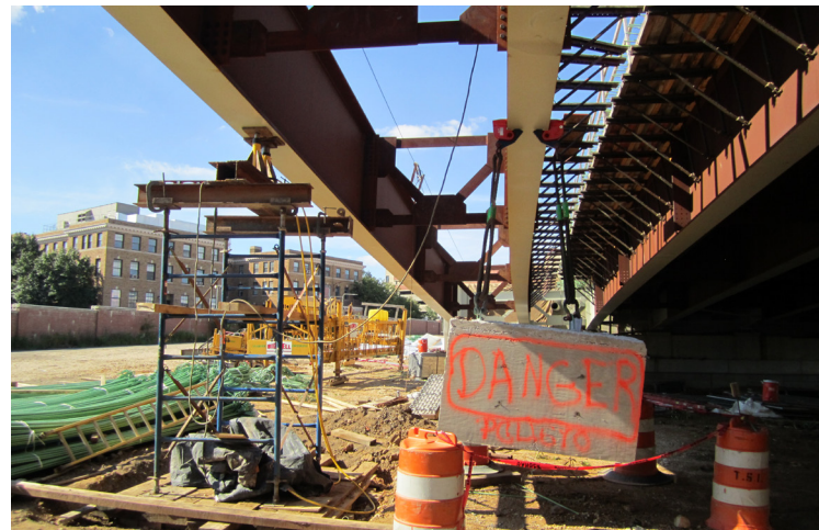
Stage 2 framing and closure bay with an upward load on G1 (jack stand) and downward load on G1 (concrete block).
