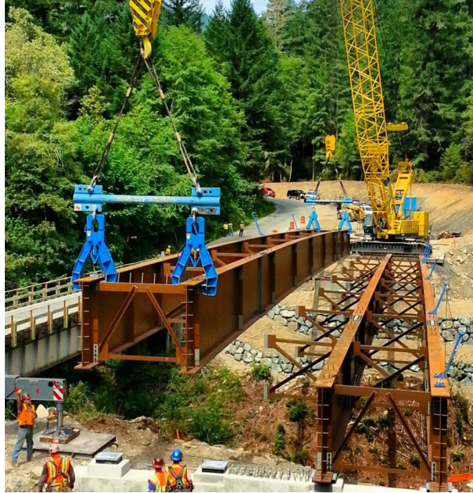
▲ The Hurdy Gurdy Creek Bridge spans were placed with two cranes, one on each side of the river.
