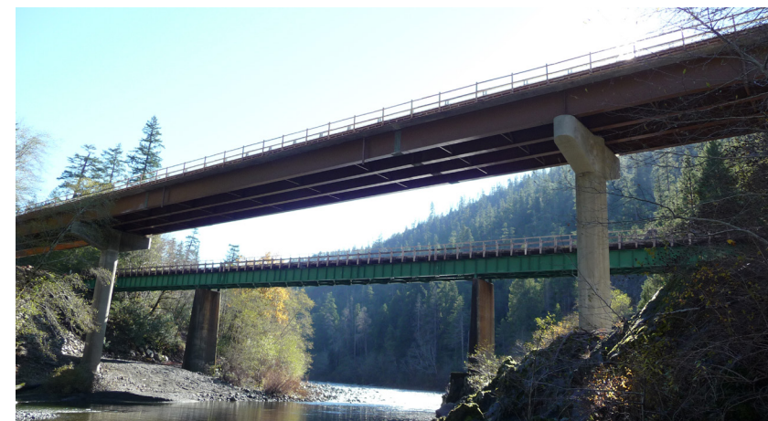
▲ The new design increased the crossing's width to 31 ft, 4 in., providing a clear roadway width of 28 ft.
