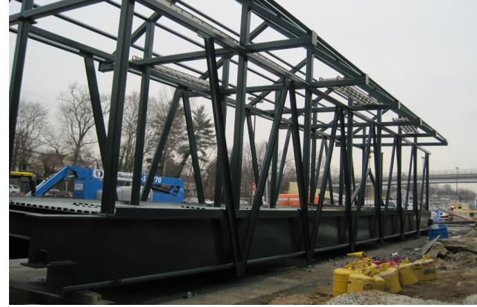
▲ The preassembled pedestrian bridge before erection.
