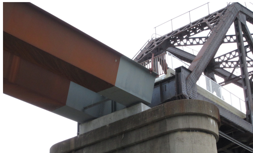
◀ The girders also house the utilities, which would have detracted from the clean lines if mounted on the outside.
