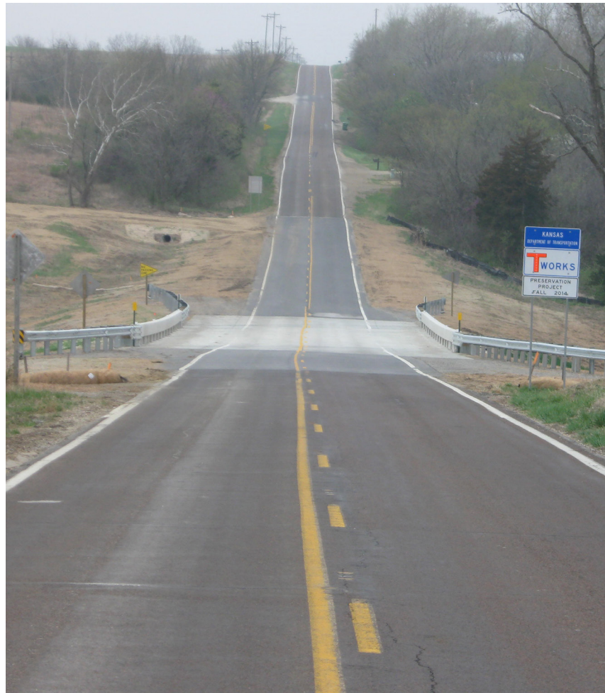
◀ The bridge crosses Blacksmith Creek near Topeka, Kan.
