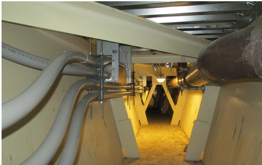
◀ The girders also house the utilities, which would have detracted from the clean lines if mounted on the outside.
