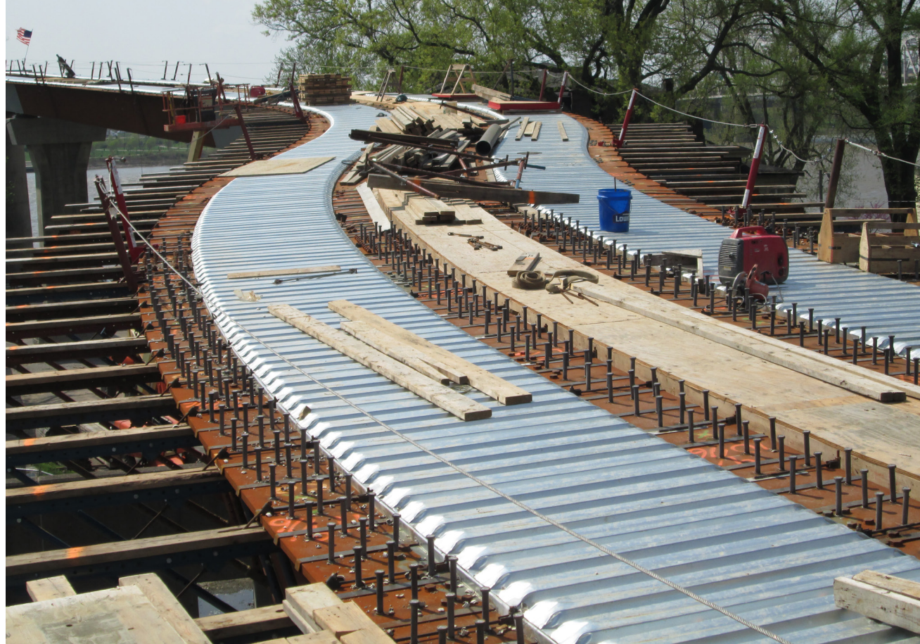
▲ ▼ While steel box girders are often used on curved long-span highway bridges for stability and structural efficiency, they are not generally used on pedestrian bridges. However, this girder type was chosen for the Jeffersonville approach because the girder fascia and bottom soffit create a streamlined look through the S-curve span and the sharp 90° curve at the end of the bridge.
