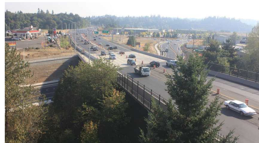
▼ The new OR 213 bridge after it was moved into place and traffic was reopened four hours earlier than originally scheduled.
