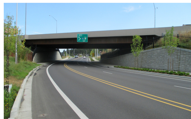
▼ The completed OR 213 bridge, as seen from Washington Street below. The new roundabout can be seen in the distance, directly east of the bridge.
