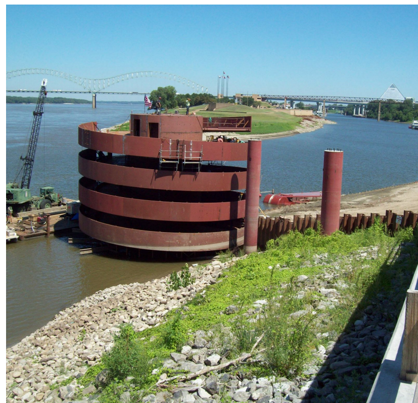
▲▼ Framing for the helical ramp consists of 55 HSS12×10×½ columns at the perimeter of a 24-ft-diameter core with ¼-in. steel plate forming the steel cylinder surface.
