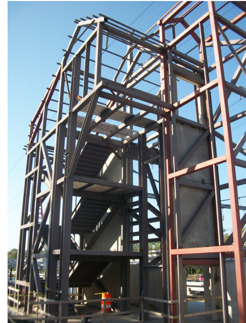
East tower framing with interior precast panels. ▶
