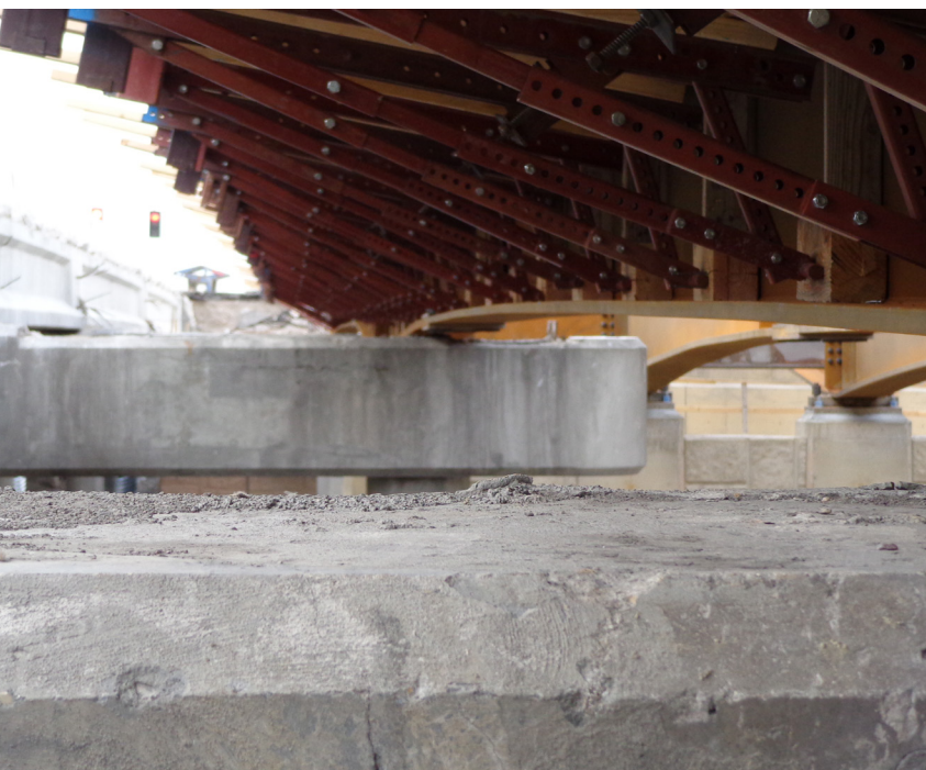
▲ Mechanically stabilized earth (MSE) walls were constructed in front of the abutments in order to minimize the span lengths, yet still provide for future Interstate widening.
