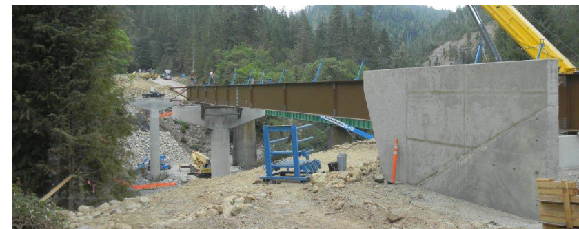
▼ The superstructure rests on two piers, 48 ft tall and 52 ft tall, as it crosses the river.
