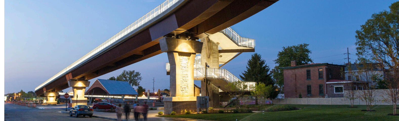
▲ A stair tower (50 ft from top of footing to highest point) provides access to the Ohio River Greenway and Jeffersonville waterfront 1,000 ft south from where the bridge lands at the Big Four Station.
