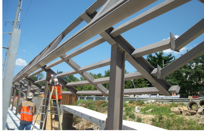
▲ Welding the canopy steel.
