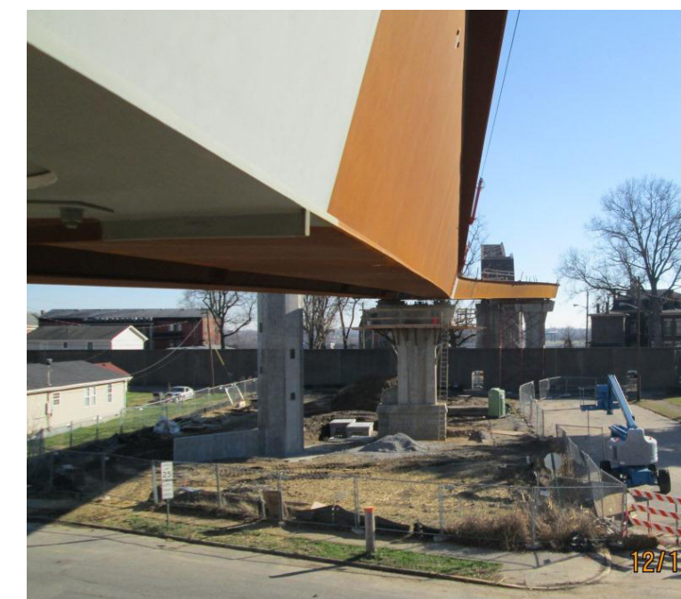
◀ Special details at the pier diaphragms ensure easier passage of the drain piping and conduit.
