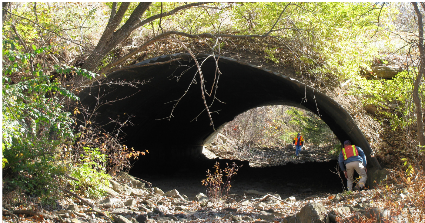
▲ The old, arched culvert had a maximum height of 12 ft in the center and a maximum width of 30 ft at the bottom.
