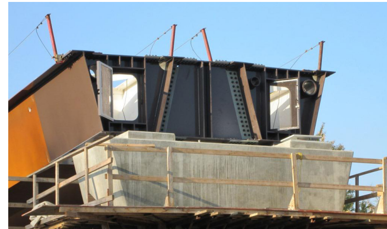
◀ Special details at the pier diaphragms ensure easier passage of the drain piping and conduit.
