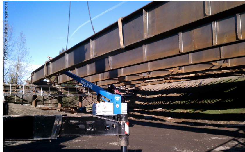
▲ Crews place the girders of the new OR 213 bridge. The girders are fabricated from ASTM A709 Grade 50 weathering steel and are 4 ft, 7½ in. deep.
