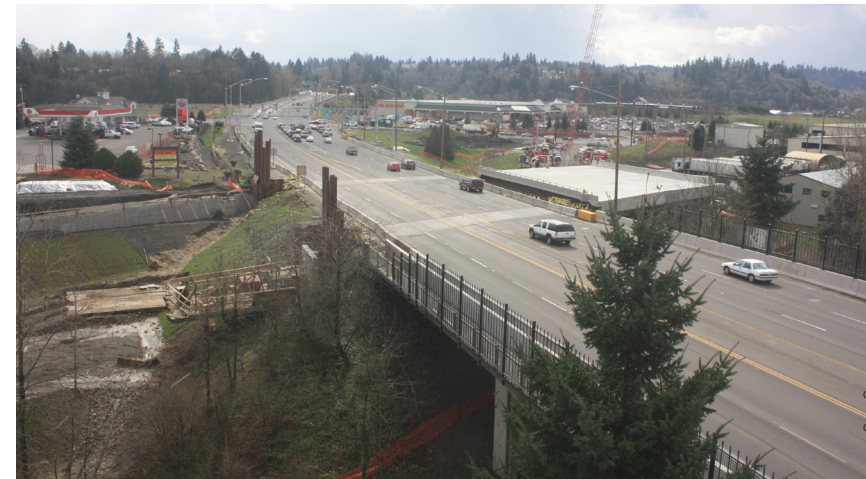
▲ A shot from the live project webcam shows the new bridge, which was constructed along the existing highway, shortly before crews pushed it into place.
