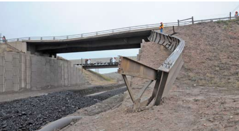
This 140-ft portable prefabricated modular steel truss bridge replaced the damaged span and allows for two lanes of traffic.
