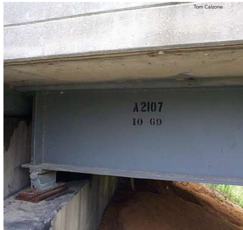
This 1999 photo shows the excellent condition of the inorganic zinc-rich coating on bridge A2107 in Missouri 30 years after its application.
