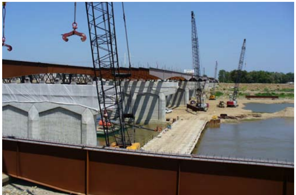
Divided into four units for planning purposes, the 3,210-ft Topeka Boulevard Bridge includes 24 spans ranging from as little as 70.5 ft to as much as 215 ft.
