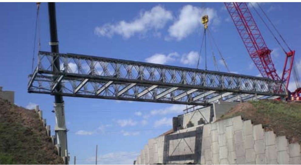
This 140-ft portable prefabricated modular steel truss bridge replaced the damaged span and allows for two lanes of traffic.
