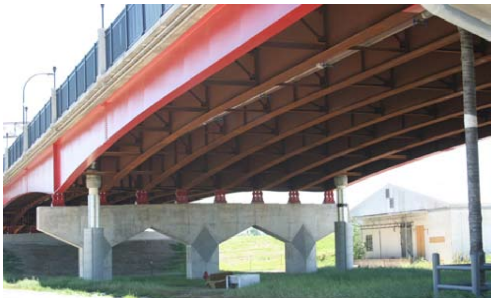
Although the bridge is constructed of weathering steel, the exterior girders and exposed bearing devices were painted for aesthetic reasons.
