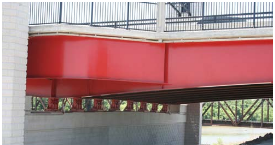
At least partly to maintain good aesthetics, observation deck extensions were added to the bridge at the gateway tower piers at the levee on each side of the river to harmonize with the widened substructure.
