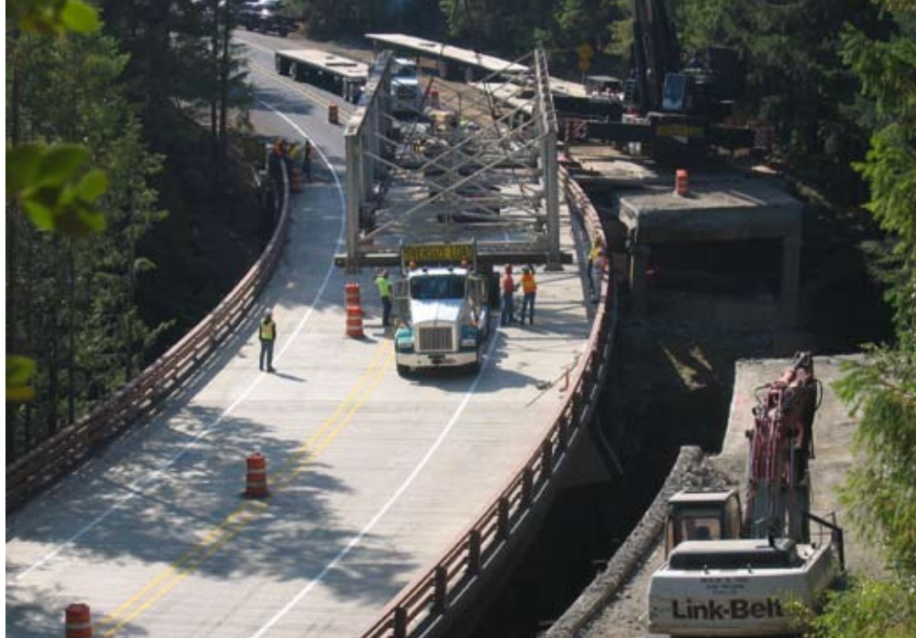
Above: To minimize disruption to its lead-based paint, the 100-ft truss from the old bridge was removed in one piece.
