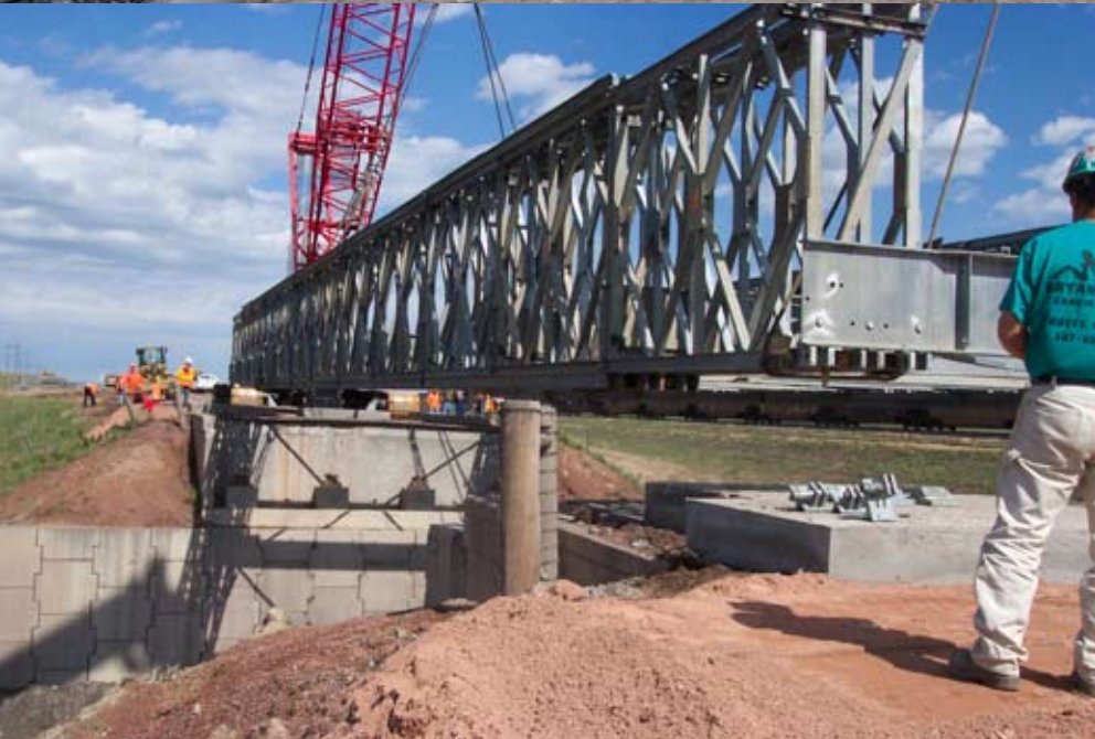
WYO 450 carries an average of 1,800 vehicles a day, and the best available detour around the damaged bridge was 32 miles long.
