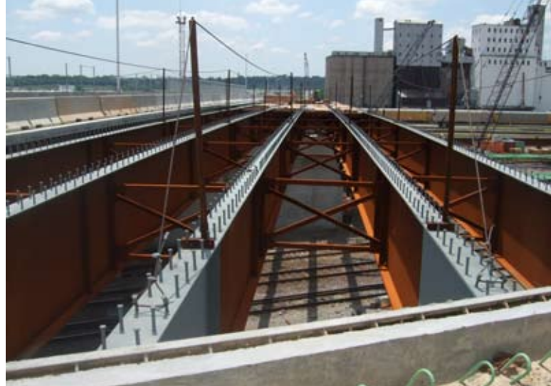
The new bridge provides the required 23-ft 6-in. minimum vertical clearance over the below railroad tracks.
