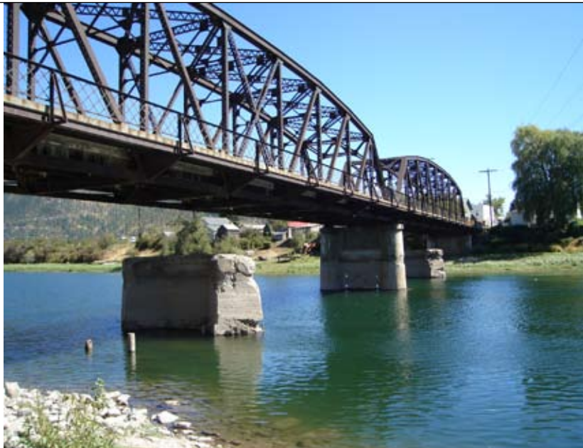
Above: Before, two 166.5-ft spans and four piers in the water.
