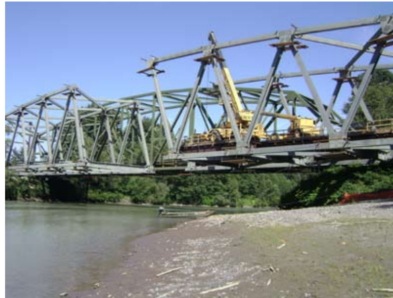
Because access for a large land-based crane was not available on the south shore of the Nooksack River crossing, the anchorage and backstay system had to support the weight of equipment as well as the truss weight.
