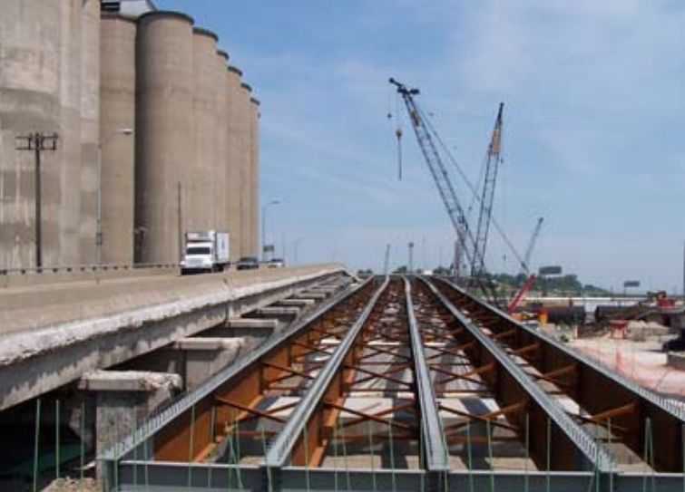
The new 7th Street bridge in Kansas City, Kan. is a 10-span two-unit steel plate girder bridge.
