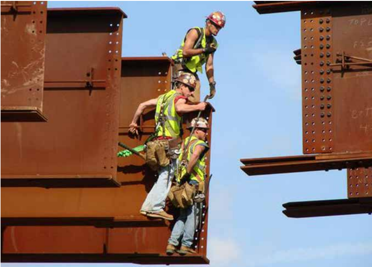
▲ Ironworkers prepare to field splice the plate girders on the West Virginia approach to the Blennerhassett Island Bridge, which used high-strength, high-performance 70 ksi weathering steel for maximum durability and improved ductility.
