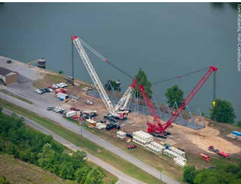
▲ The truss is assembled on the lakeshore...
