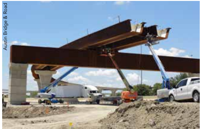
▲ Fig. 4: Steel box straddle bents were introduced to reduce the required spans of the superstructure over I-30.
