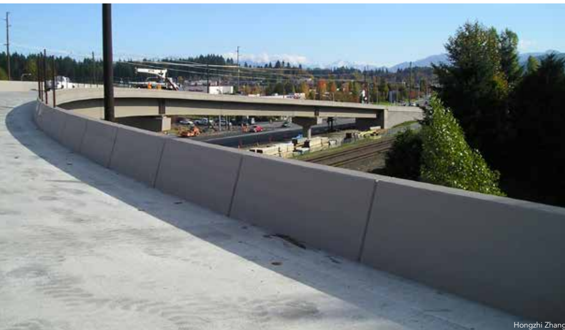
◀ The SR522 BNSF Flyover Bridge in November 2011, a month before it opened.
