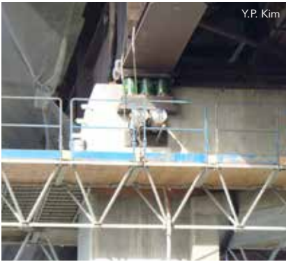
▲ Steel cylinders inserted through holes cored in the pier cap provided a base for hydraulic jacks, which lifted the girders to allow replacement of the original bearings with isolation bearings.
