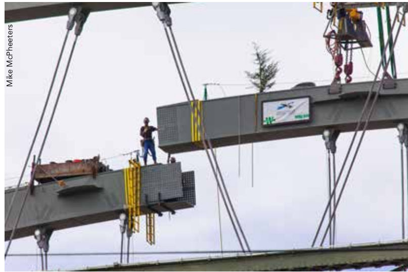
▲ The final arch rib, complete with topping out tree, being lifted into place.
