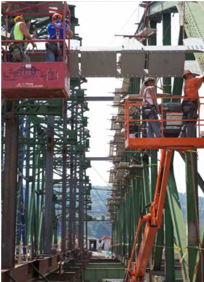
▼ Erecting the new steel. Approximately 120 tons were added.
