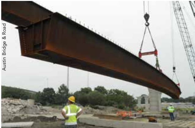
▲ Fig. 3: The contractor was able to bolt an entire span on the ground and lift it as one girder, eliminating the need for shoring towers.
