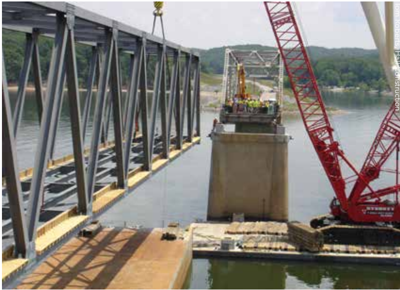
▲ The new section, shown here being lifted into place, weighs approximately 300 tons.
