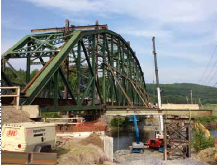
▼ Erecting the new steel. Approximately 120 tons were added.
