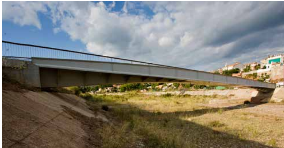
▲ Fig. 3. Matadepera pedestrian bridge.
