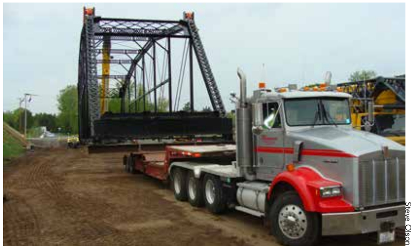
▲ In the spring of 2011 crews reassembled the truss on the ground near its new location, after which it was trucked into position for hoisting into place.
