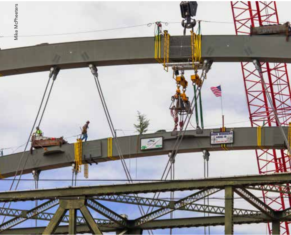
▲ The final arch rib, in place.
