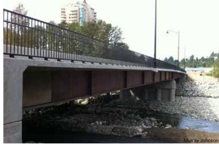
▲ The completed New Capilano River Bridge.
