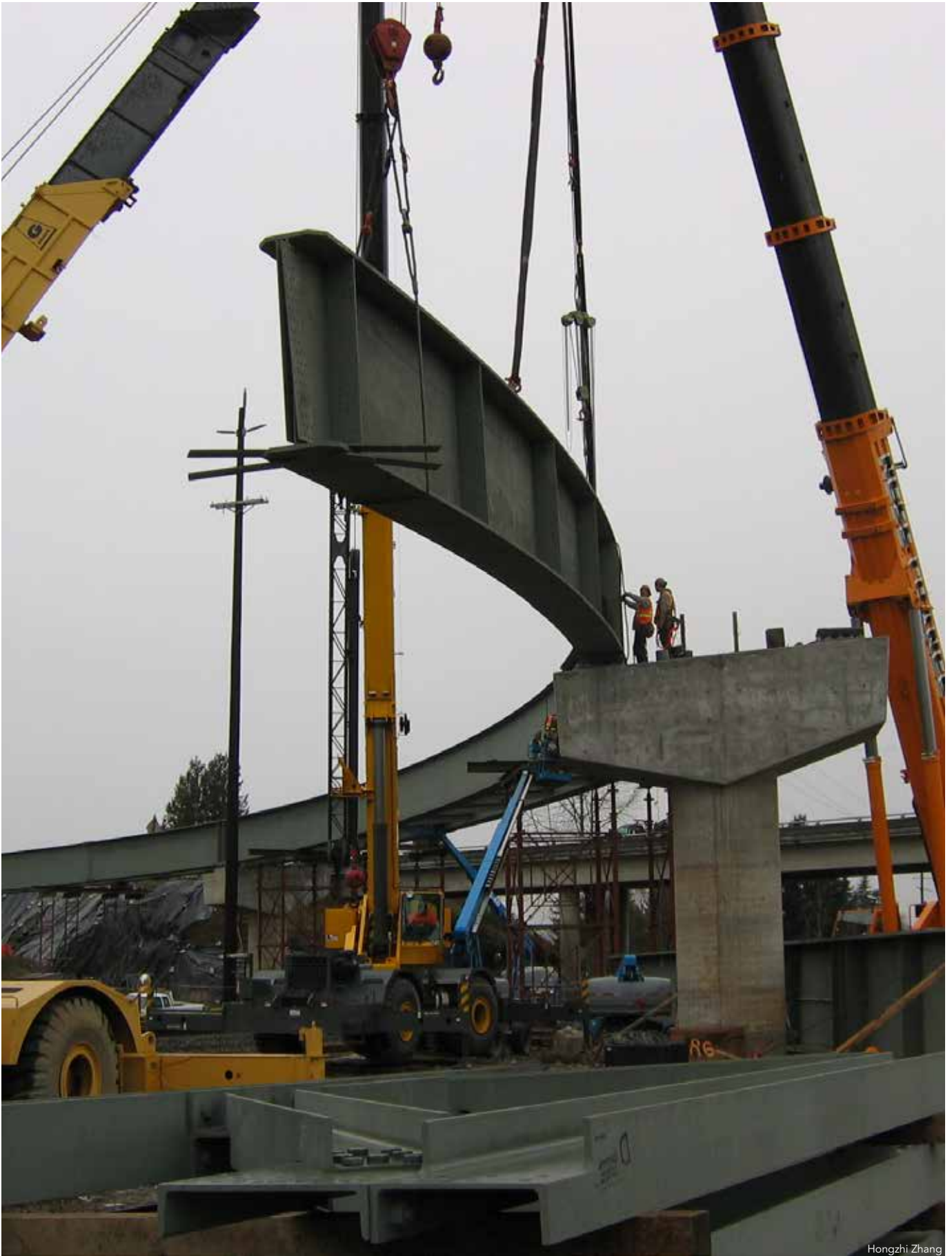
▲ Two cranes hold the curved girder during erection.
