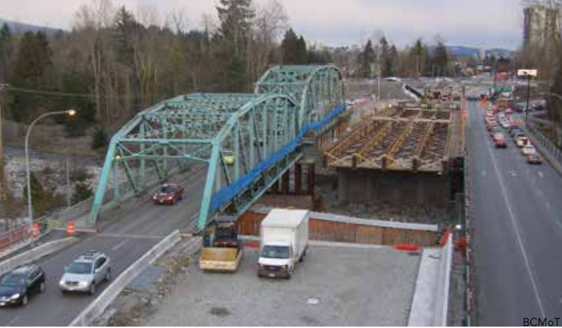
▲ New steel girders being launched from the Capilano River's east bank, over the river pier and closing in on west abutment.
