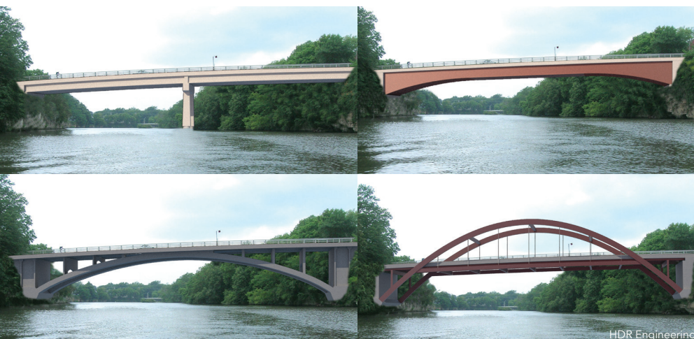
▲ The four bridge alternatives that were considered. Clockwise from upper-left: a prestressed concrete girder, a haunched steel girder, a partial through steel arch (the selected design) and a concrete deck arch.
