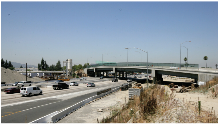
▲ The new bridge raises the vertical clearance from 15 ft to nearly 17 ft to meet current Caltrans requirements.
