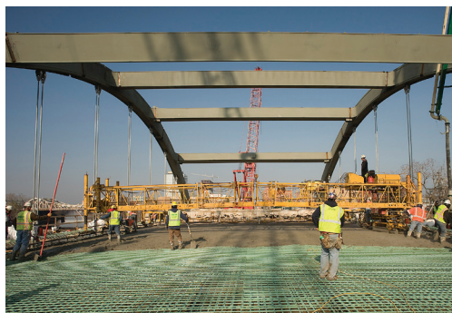
▲ Construction of the deck.
