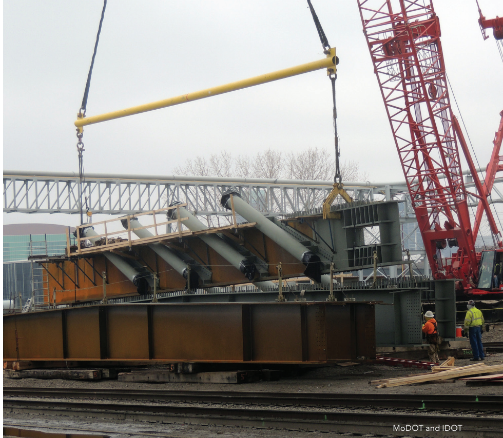
▲ All of the structural steel elements on the bridge are made of weathering steel.
