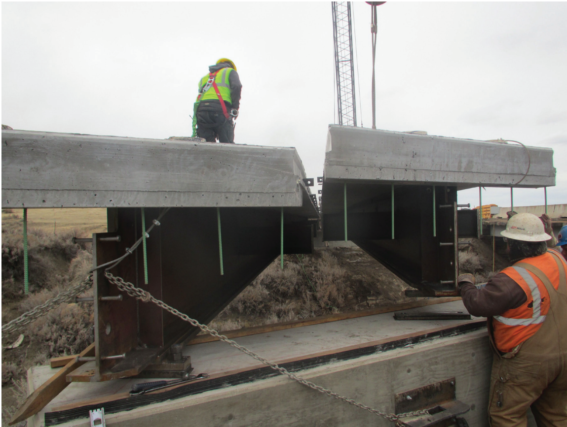
▲ The Maxwell Coulee Bridge was engineered into six modules, each approximately 7 ft by 110 ft and comprised of one girder, with diaphragm bracing and an 8-in. concrete deck.
