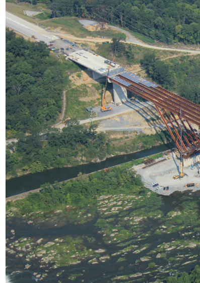
▲ The superstructure consists of a five-girder, four-substringer system supported by five lines of delta legs—one for each girder.
