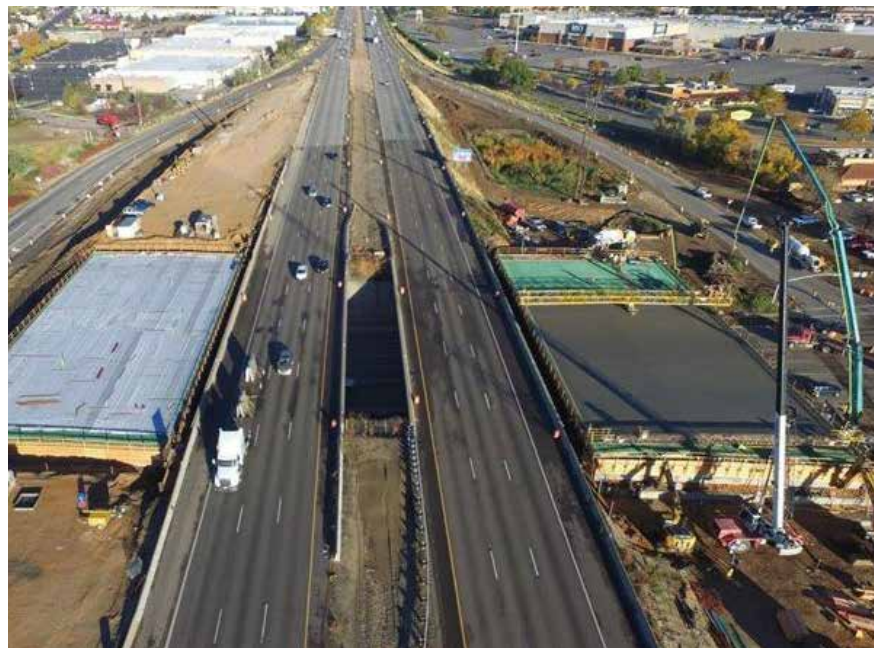
▼ The new superstructures were built next to the existing ones.
