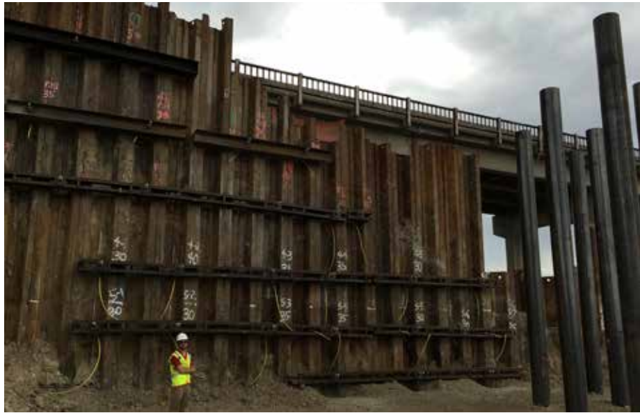
Temporary shoring to support the roadway near the proposed south abutment.
