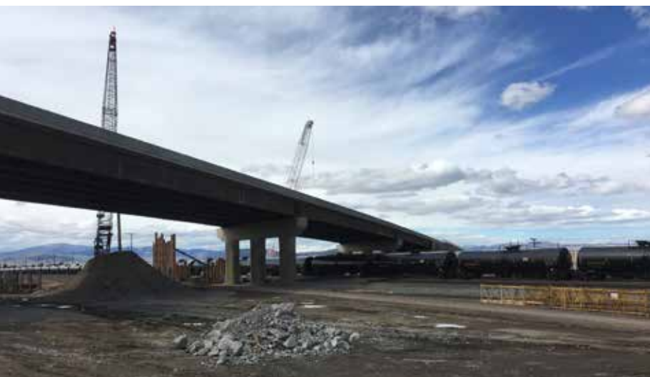
The chosen bridge span arrangement required three railroad tracks to be relocated in advance of construction.
