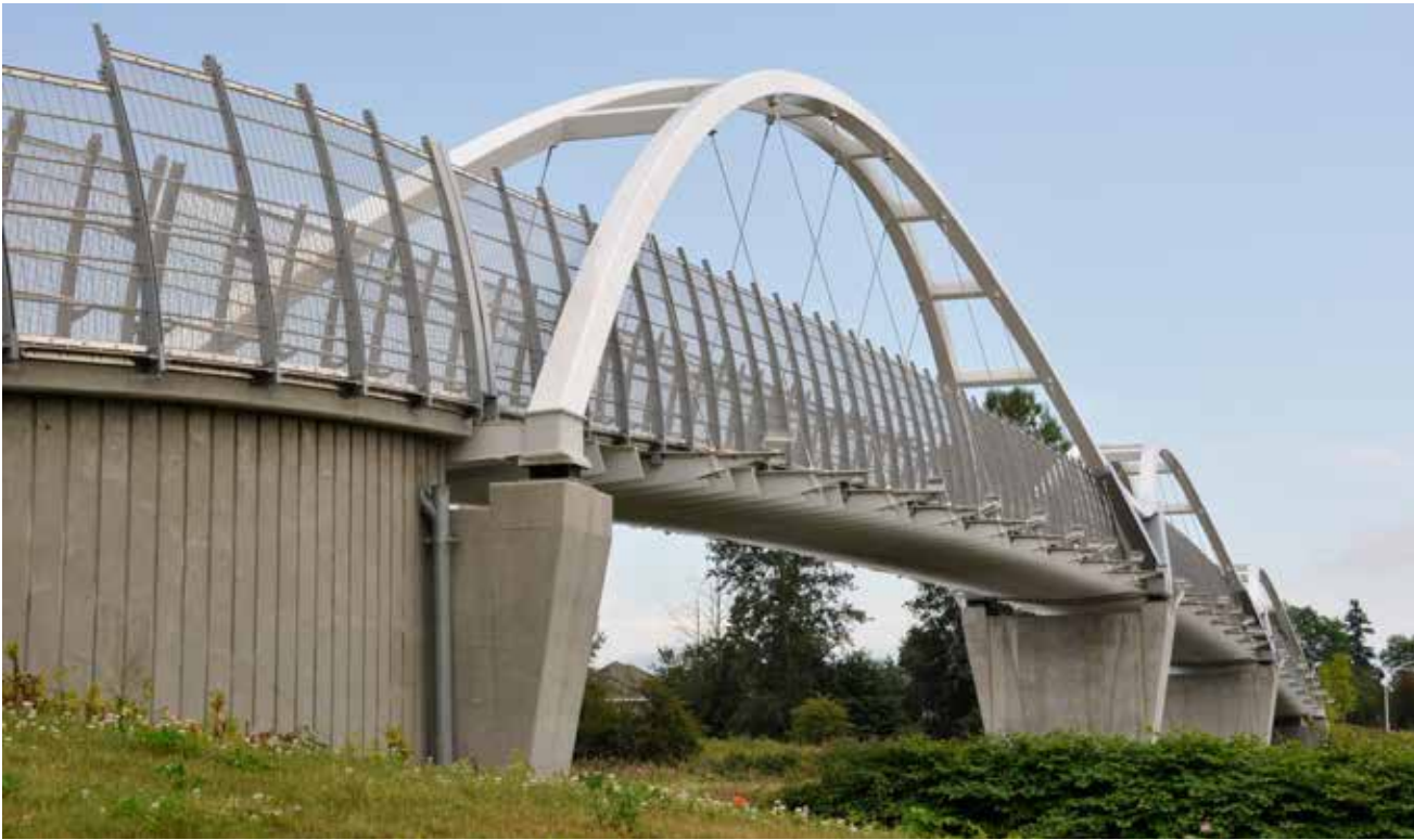
▲ This pedestrian bridge provides safe passage over a busy divided highway. A central support breaks the span. The deck is suspended from arched elements, and an artistic barrier prevents falls.
