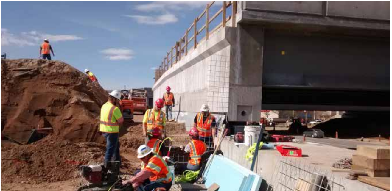
▲ Wing wall construction, following the slide.
