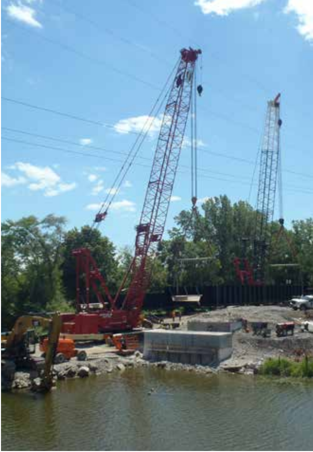
▲ Picking the new span up from the lay-down yard. ◀ Removing an existing span.
