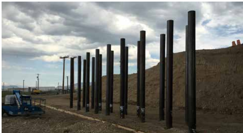
Crews had to deal with the area's relatively short seven-month construction season.
