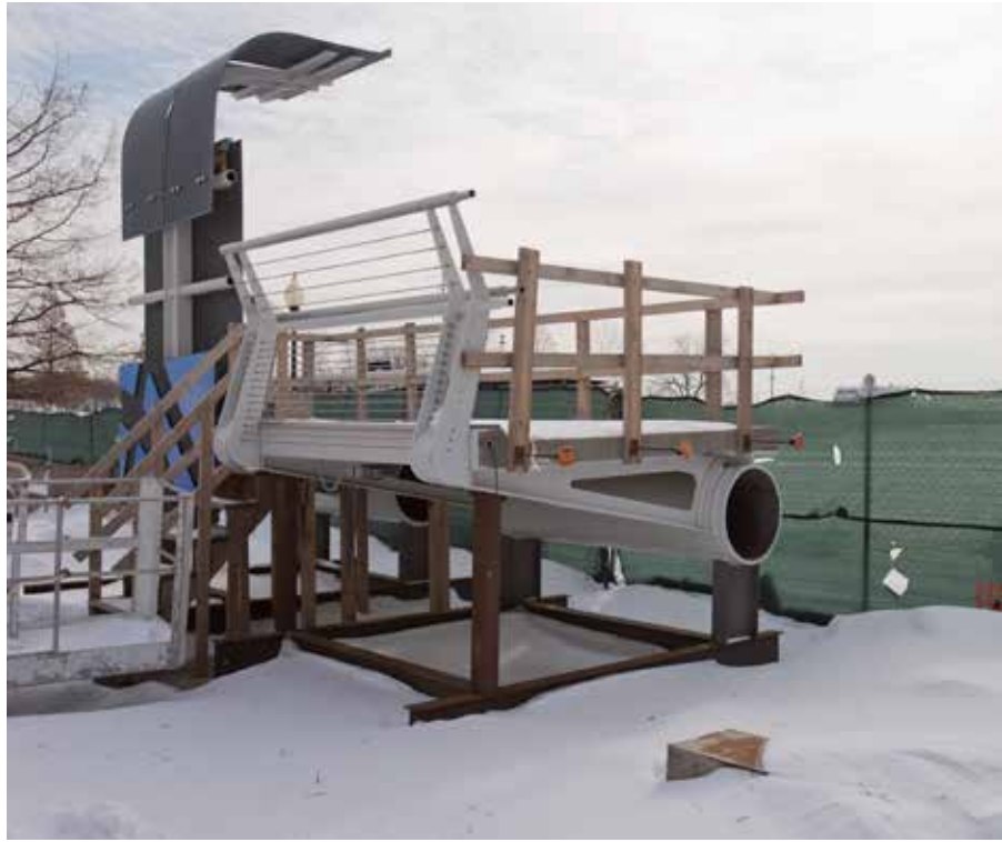
▲ A full-scale mockup of the spine, deck and railings was constructed on-site to refine the details.
