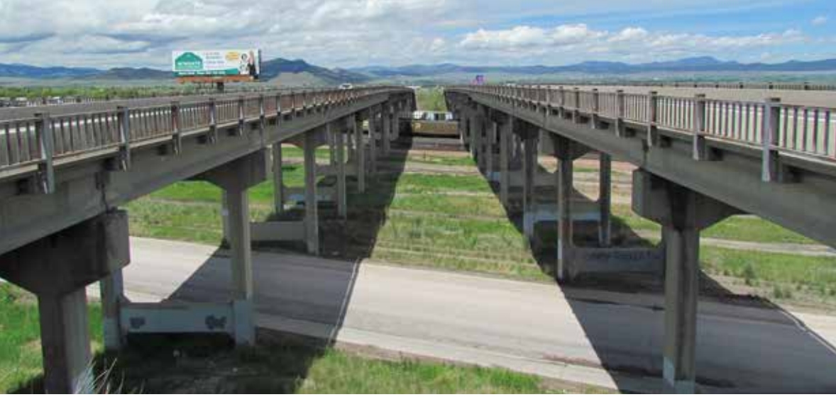
right: Driven steel piling was determined to be an adequate foundation type.
