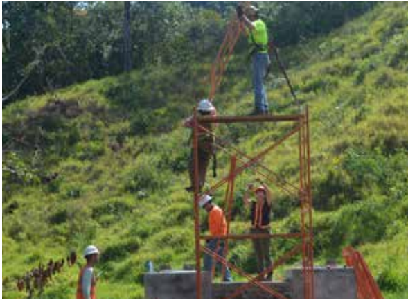
Patrick Montgomery and team putting together scaffolding.
