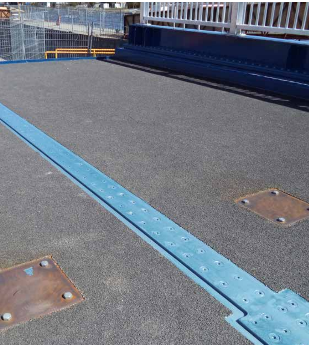
▲ A view of the longitudinal bolted splice between the orthotropic steel deck panels before asphalt was added. The panels were delivered with an anti-skid waterproofing membrane that was preinstalled by the fabricator for durability and worker safety during the wet winter months.
