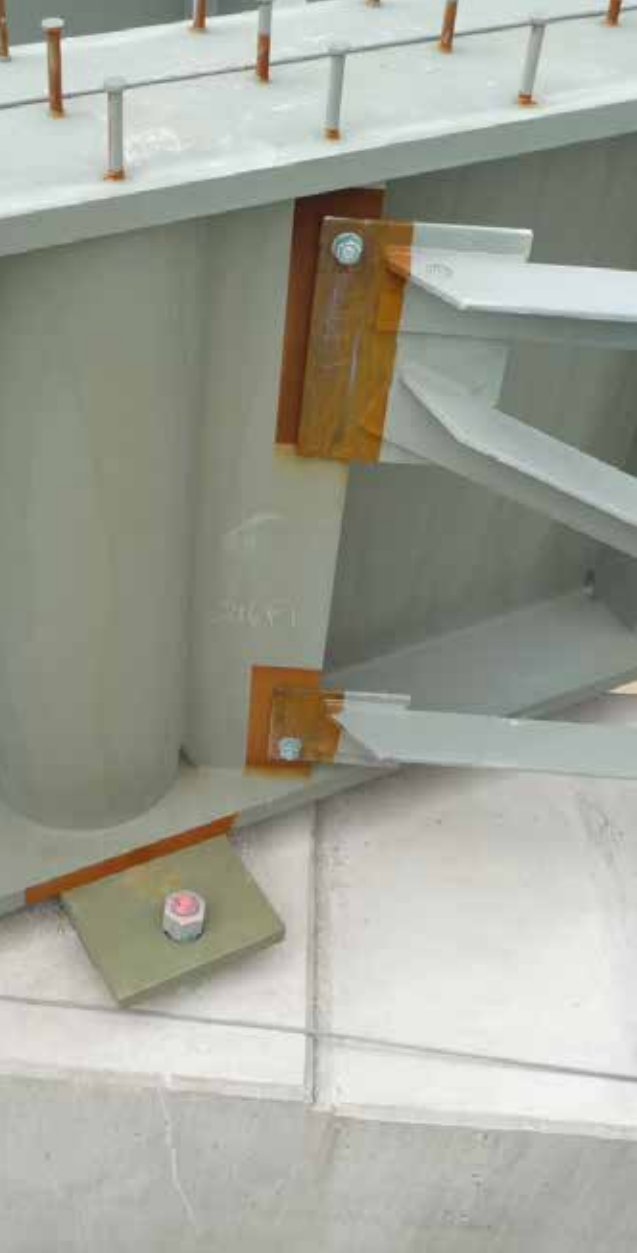
▲ An SPBS used for a cross frame connection along a highly skewed bent line.
