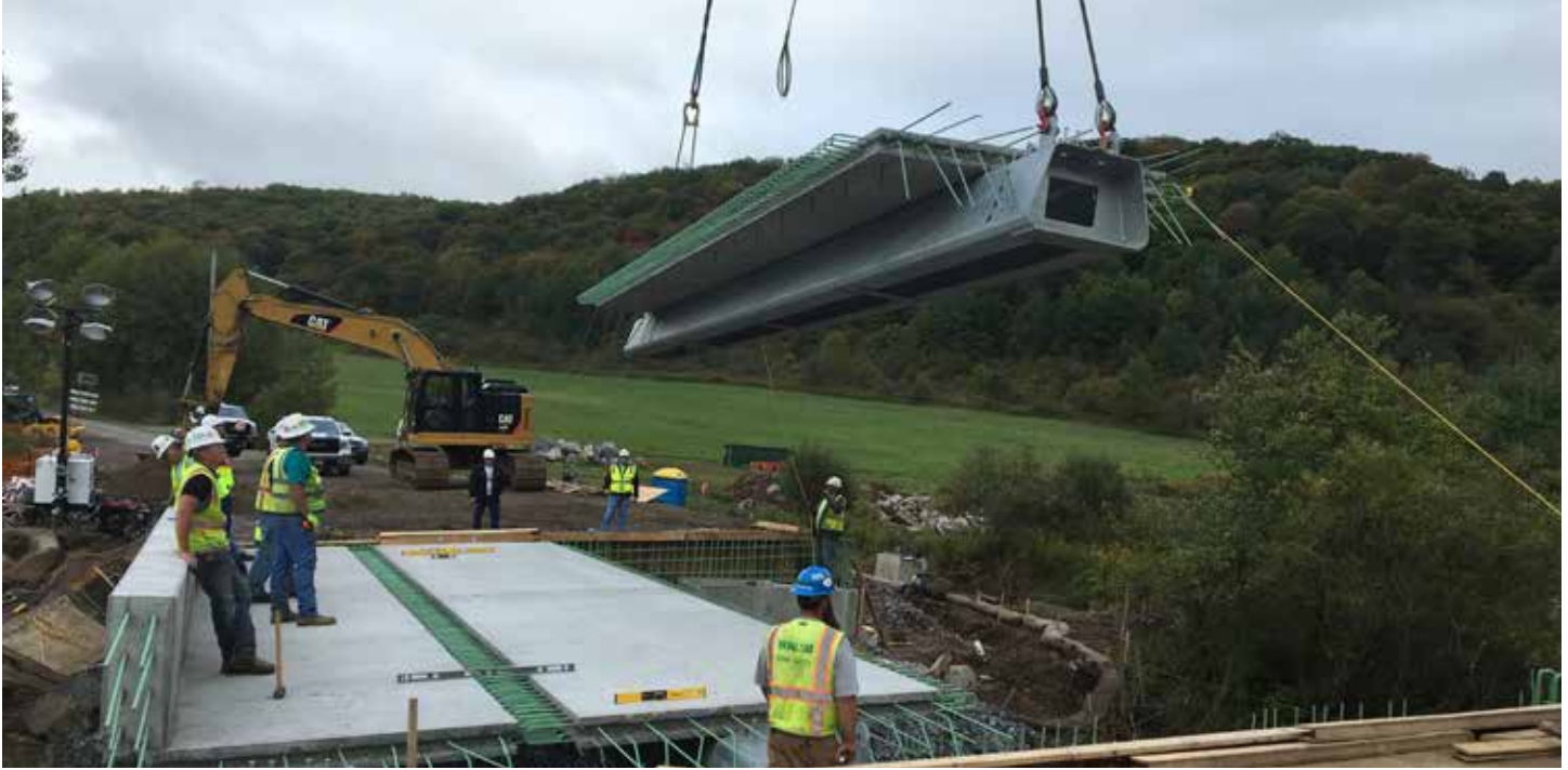
▲ Installing the third section.
