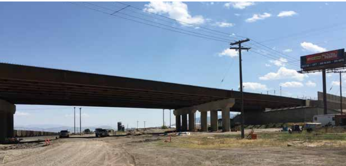
right: Driven steel piling was determined to be an adequate foundation type.
