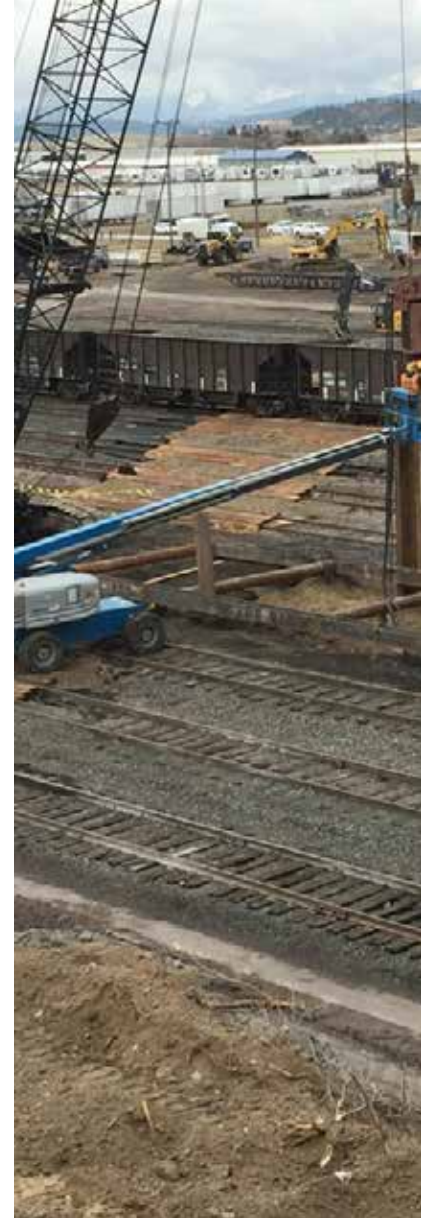
right: Driven steel piling was determined to be an adequate foundation type.
