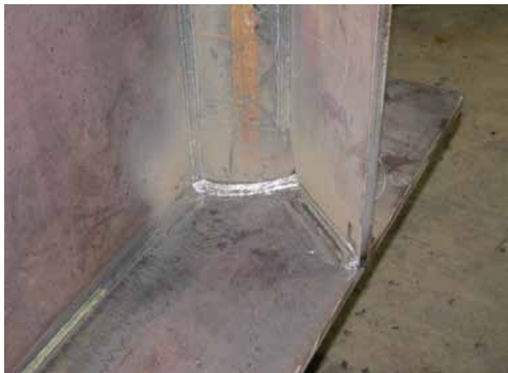
▲ Cross frame connection details at highly skewed support bearings. ▼ A weld detail at a web-to-flange connection (note that weld access is provided on the acute side).
