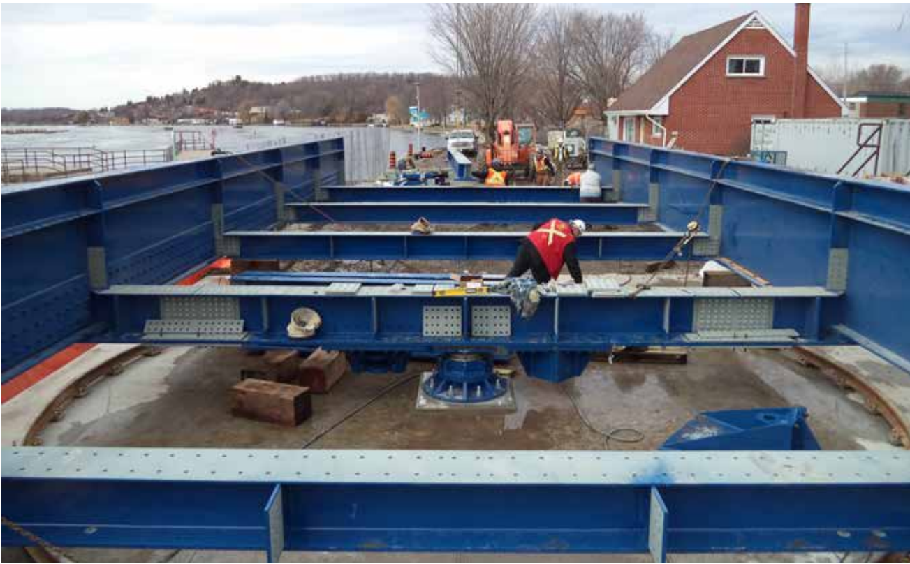
▲ A view of the steel superstructure prior to installing the OSD. The transverse floor beams of the OSD were used as a template to drill matching holes in the superstructure above.
