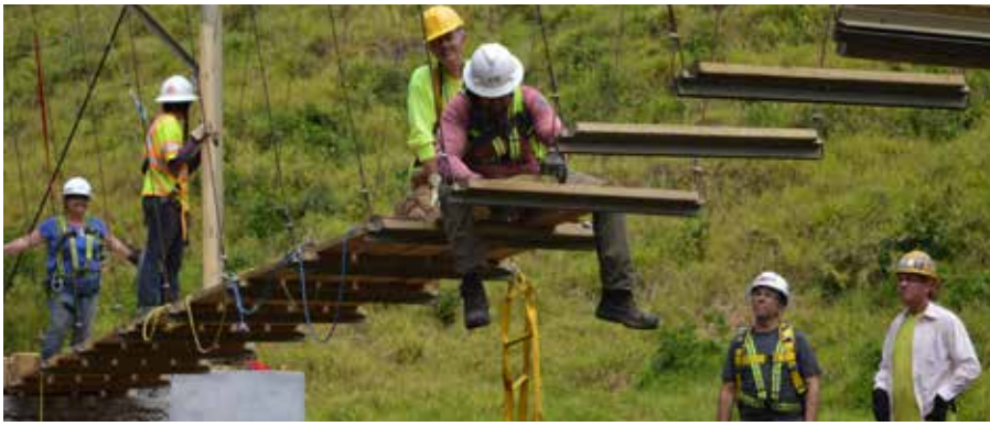
Carter Bearden and Gary Kinchen installing decking near the middle of the bridge span.
