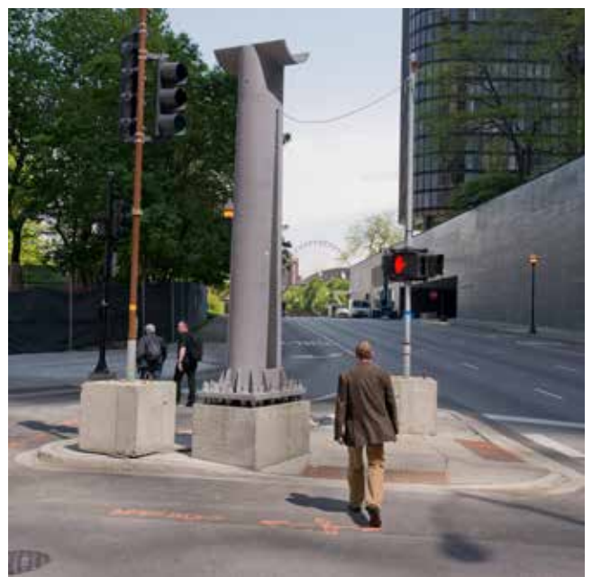
▼ The paint system is not the typical zinc/epoxy/urethane system used on highway bridges, but rather a three-coat system comprised of a primer, an intermediate coat and a fluoropolymer finish coat. Typically used on building applications, this system is highly durable and provides enhanced color and finish retention.
