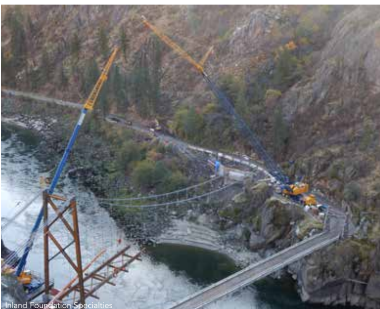
Inland Foundation Specialties
