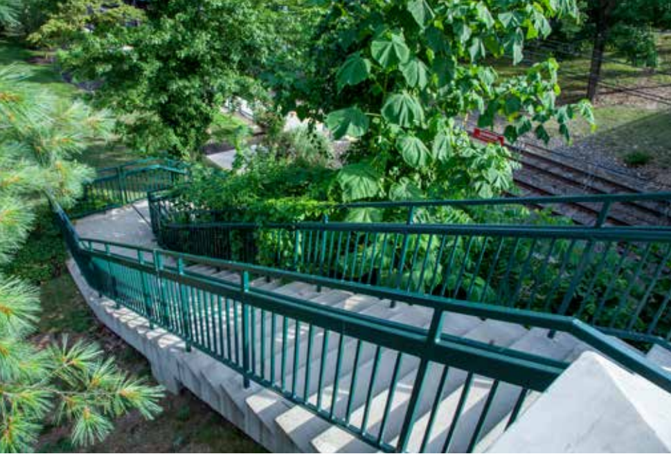
◀ Stairs from street level down to the SEPTA tracks.
