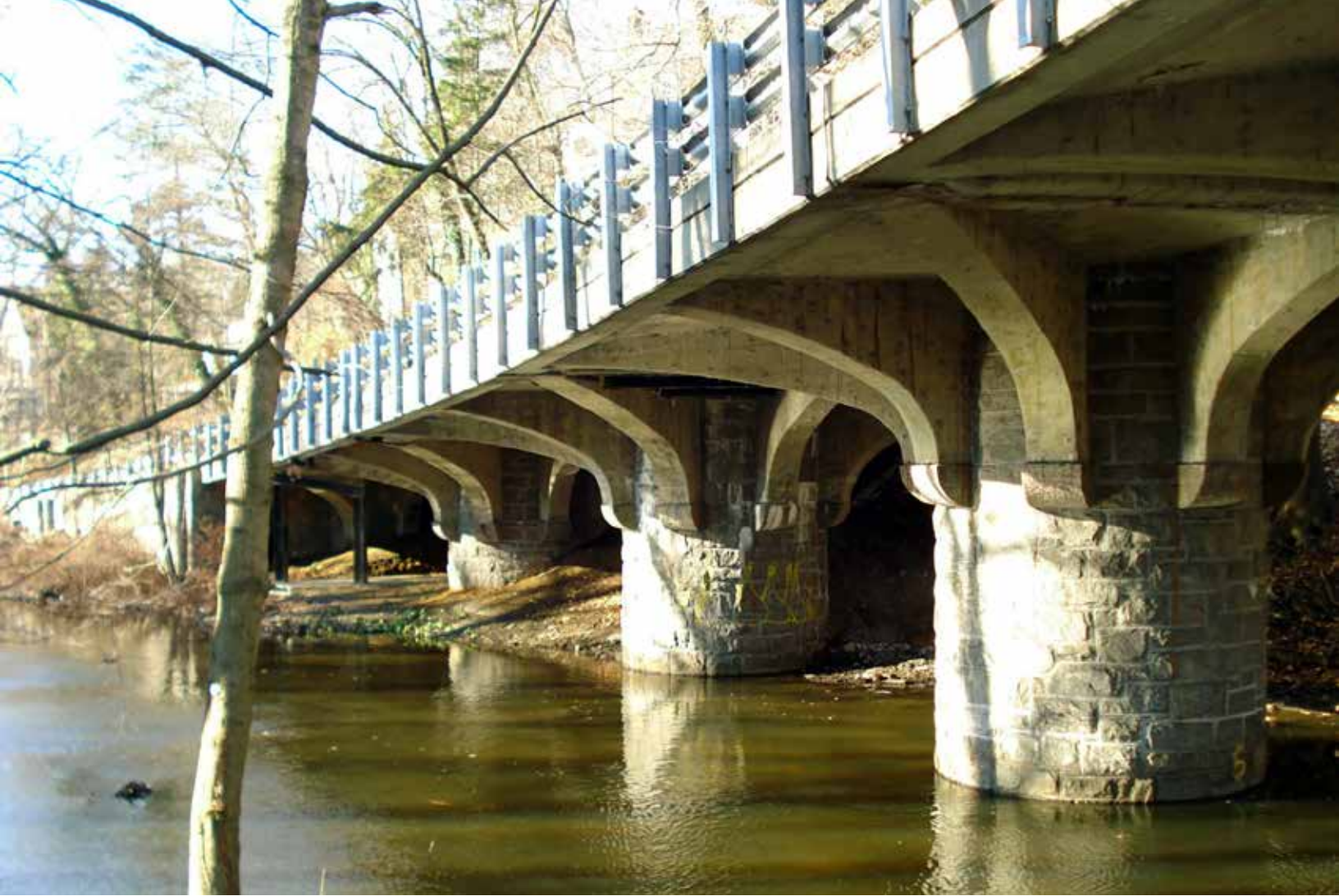
▲ The bridge's uniquely shaped piers gave it its Mushroom Bridge nickname.
