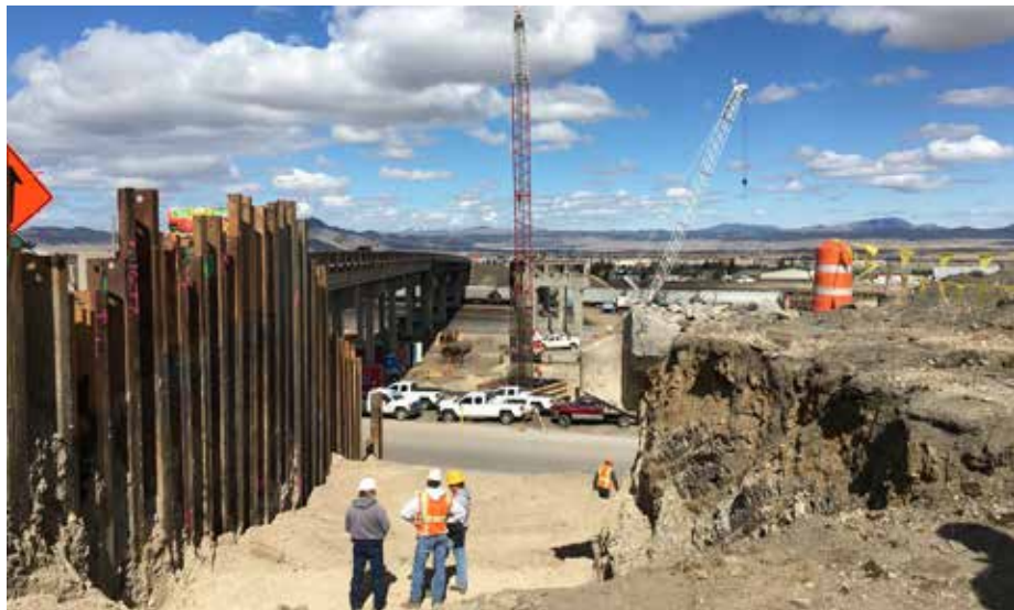
A critical part of the project sequencing was the requirement that the first new bridge be built during the first construction season.
