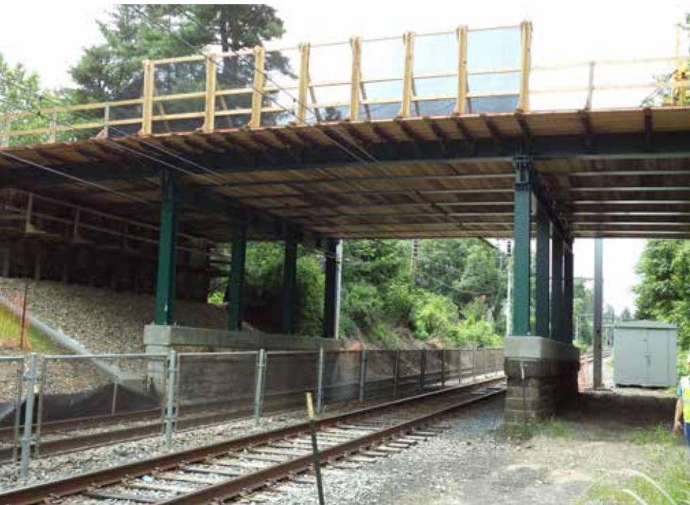
▲ The design scheme mimicked the existing configuration of very shallow, closely spaced stringers.
