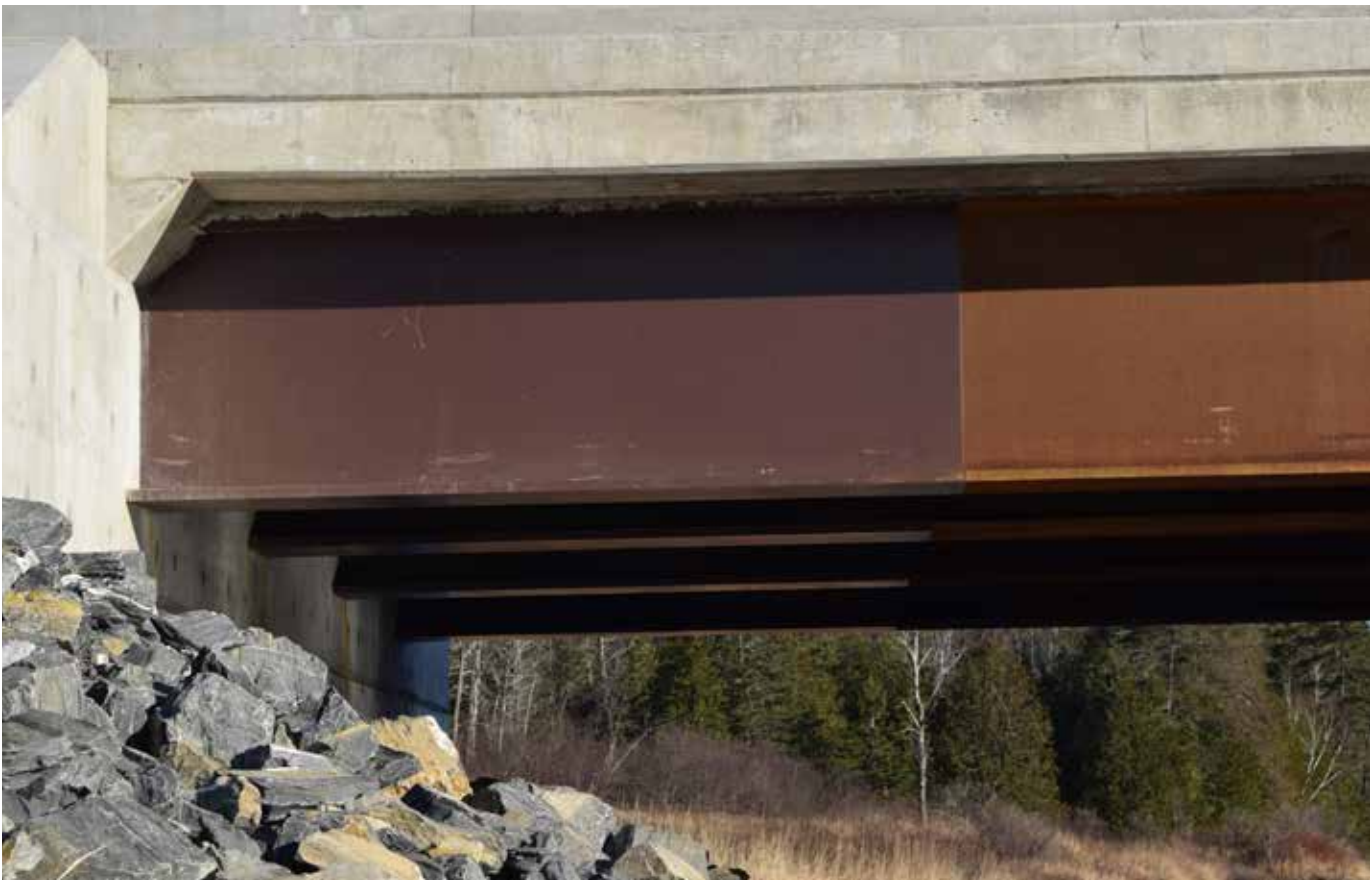
A close-up view of one of the painted beam ends on the Main St. bridge project.
