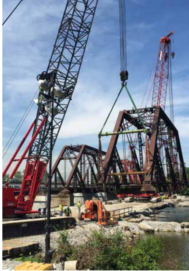
▲ Placing an old span on an island downstream to make way for the new spans.
