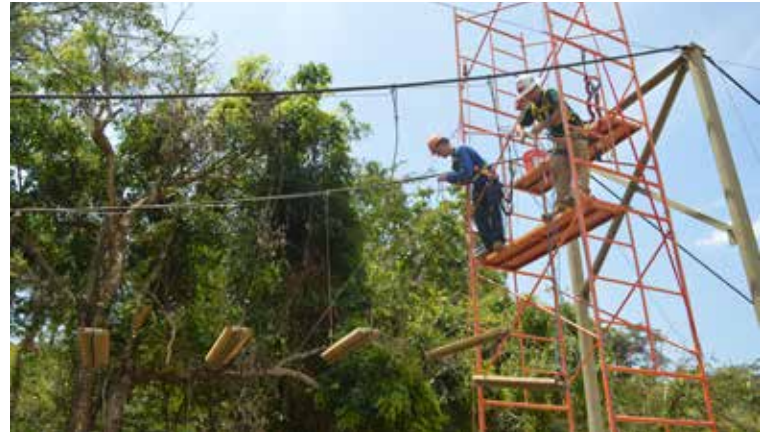
John Hastings and Jeff Carlson installing hanger assemblies.
