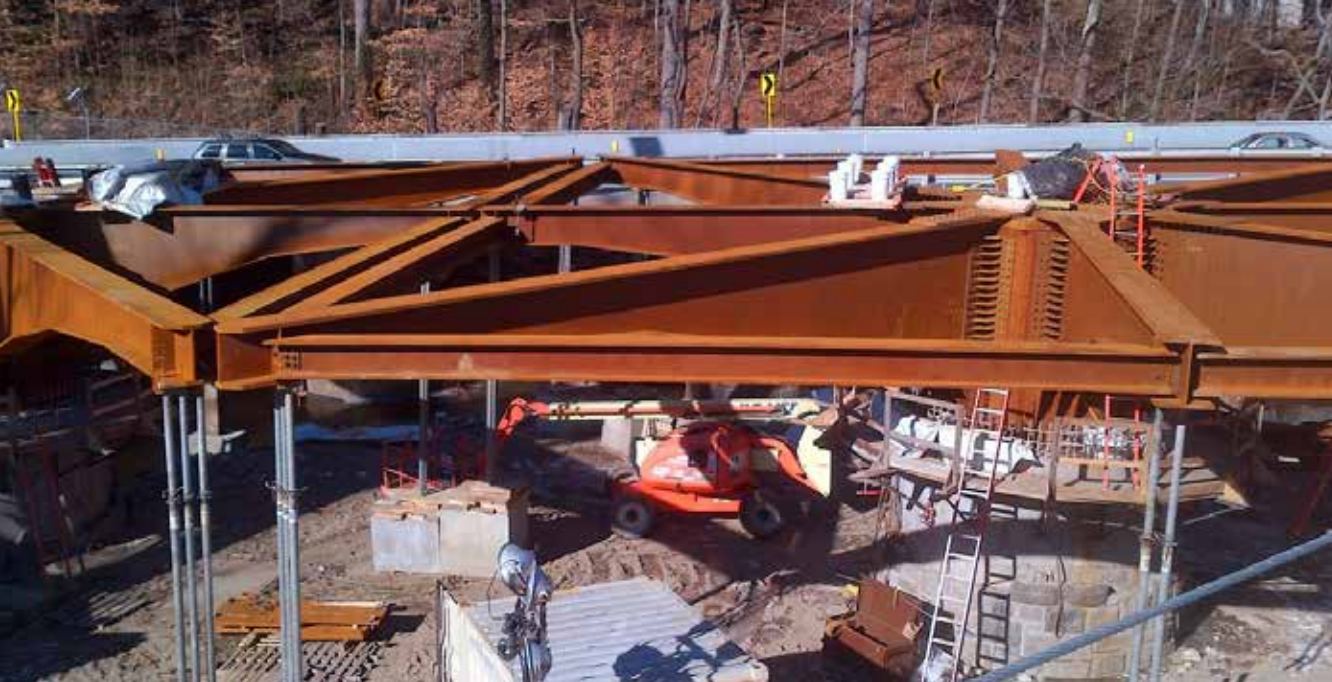
◀ The partially erected Mushroom Bridge, showing steel core and steel brackets.
