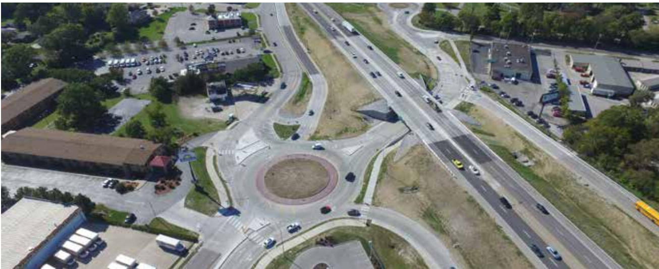
▲ An aerial view of the I-70 bridge over Business Loop, which replaced two existing bridges.
