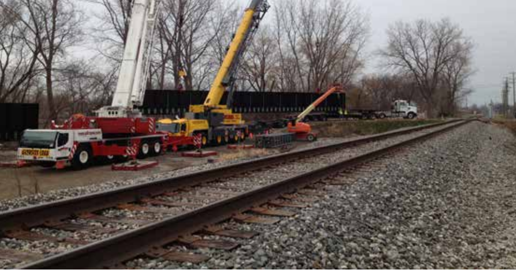
◀ Unloading steel in the lay-down yard.
