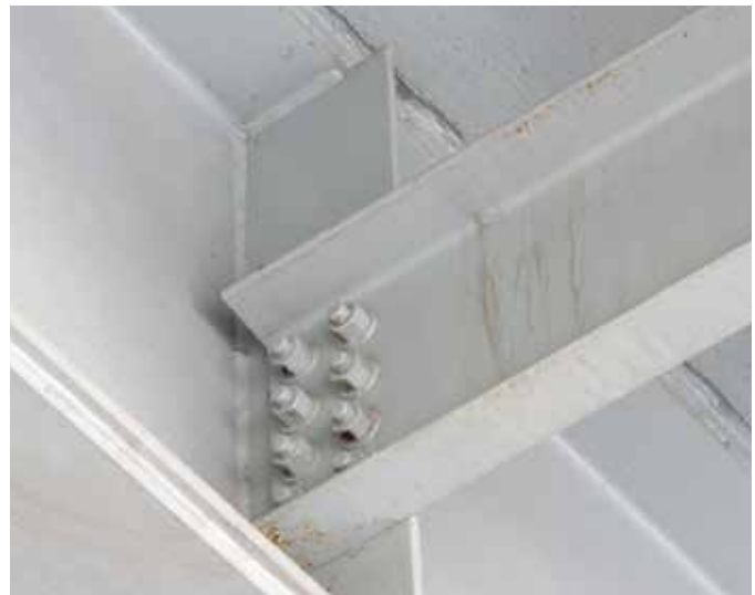
A Connecticut DOT project—I-75 over Starr Ave. in Danbury—was repainted in 2002 with a PAS system. After 15 years in service, minimal rust has been experienced.
