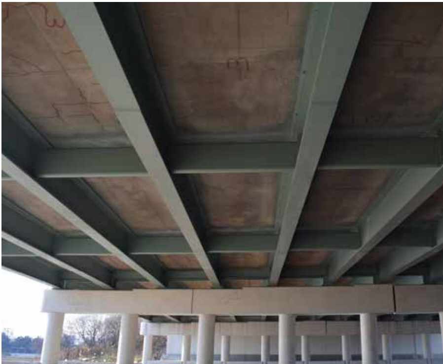
A Michigan DOT project—West Road over I-75 in Woodhaven, Mich.—was repainted with a PAS system in 2017.
