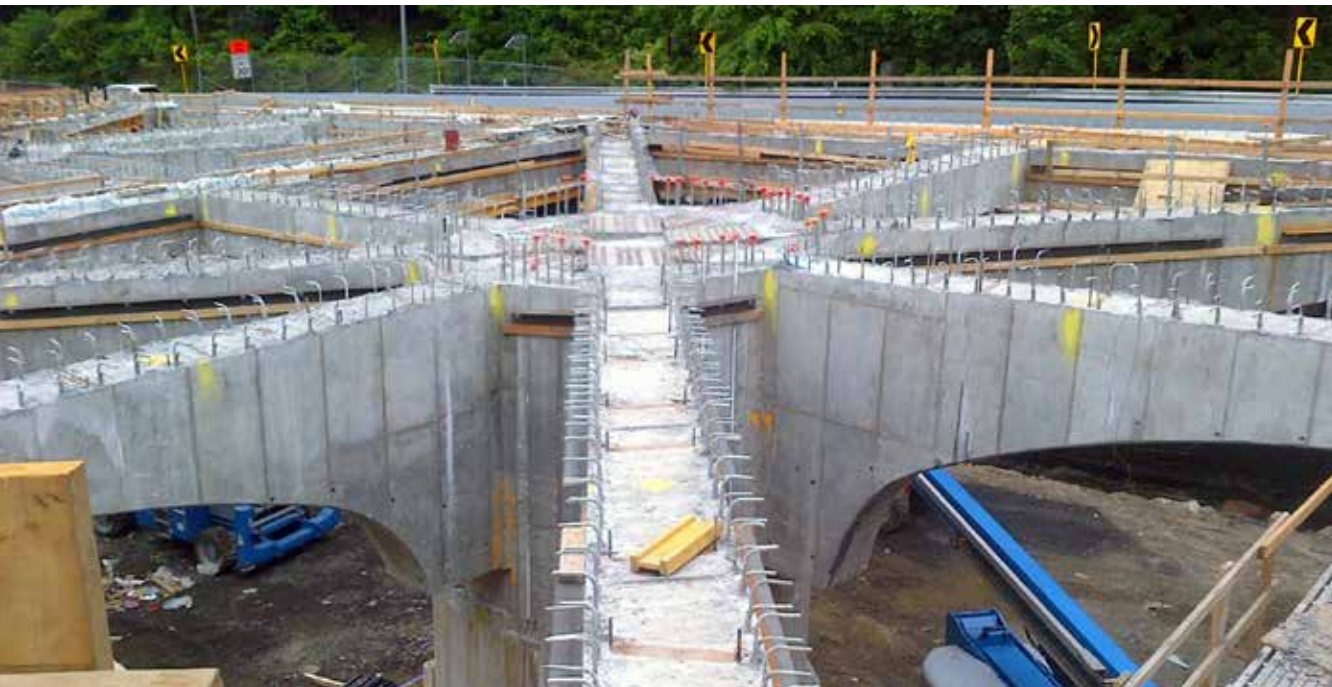
◀ The bridge's concrete-encased brackets and core.
