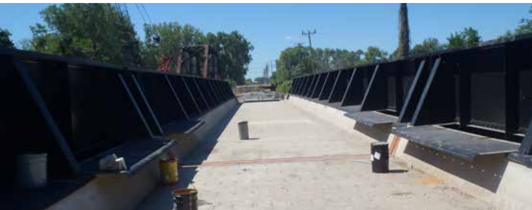
◀ A view, from the deck, of two new spans set onto new piers.
