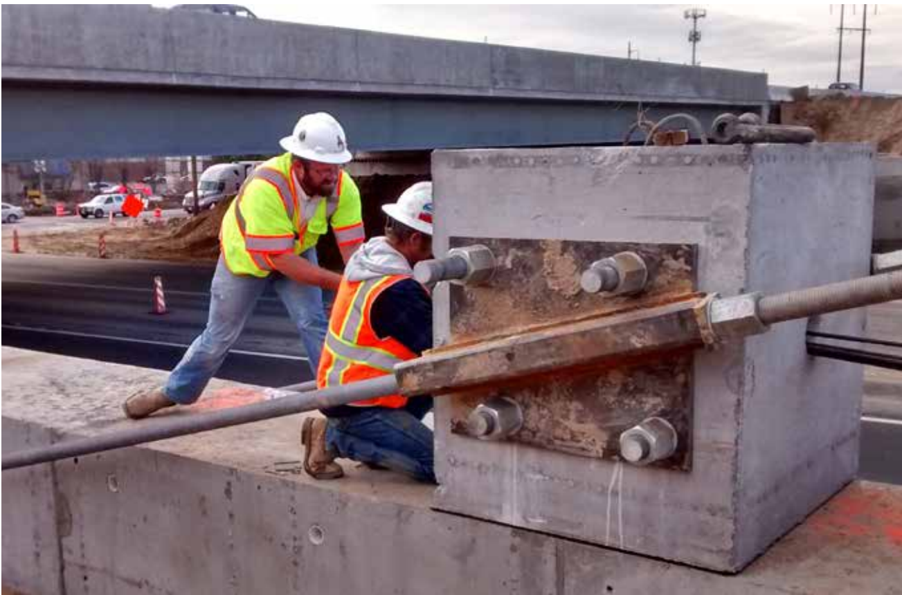
▲ The prestressing resistance anchor block used in the slide.
