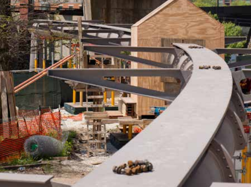
▲ Steel plate rib elements are connected to each side of the steel spine on 8-ft centers, tapering in depth from approximately 2 ft, 2 in. at the central spine to less than 5 in. at the outer deck edge.
