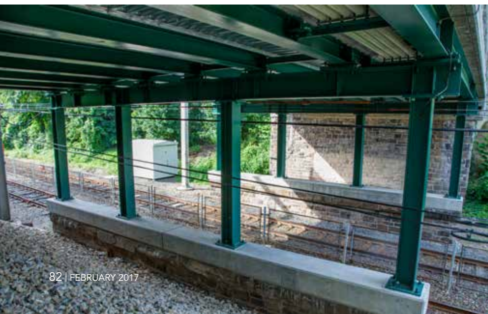
▲ The design scheme mimicked the existing configuration of very shallow, closely spaced stringers.
