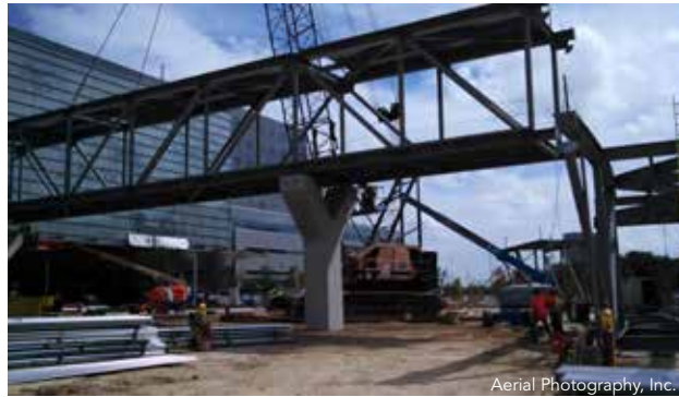
▲ Installing one of the truss segments.
