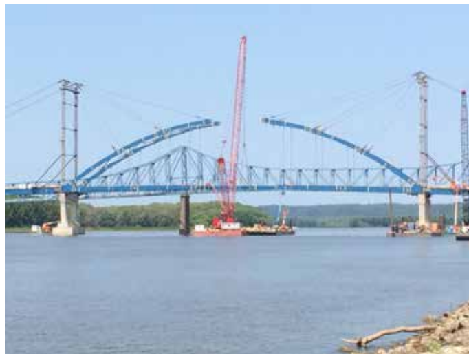
▼ Erection of the cantilever arch.
