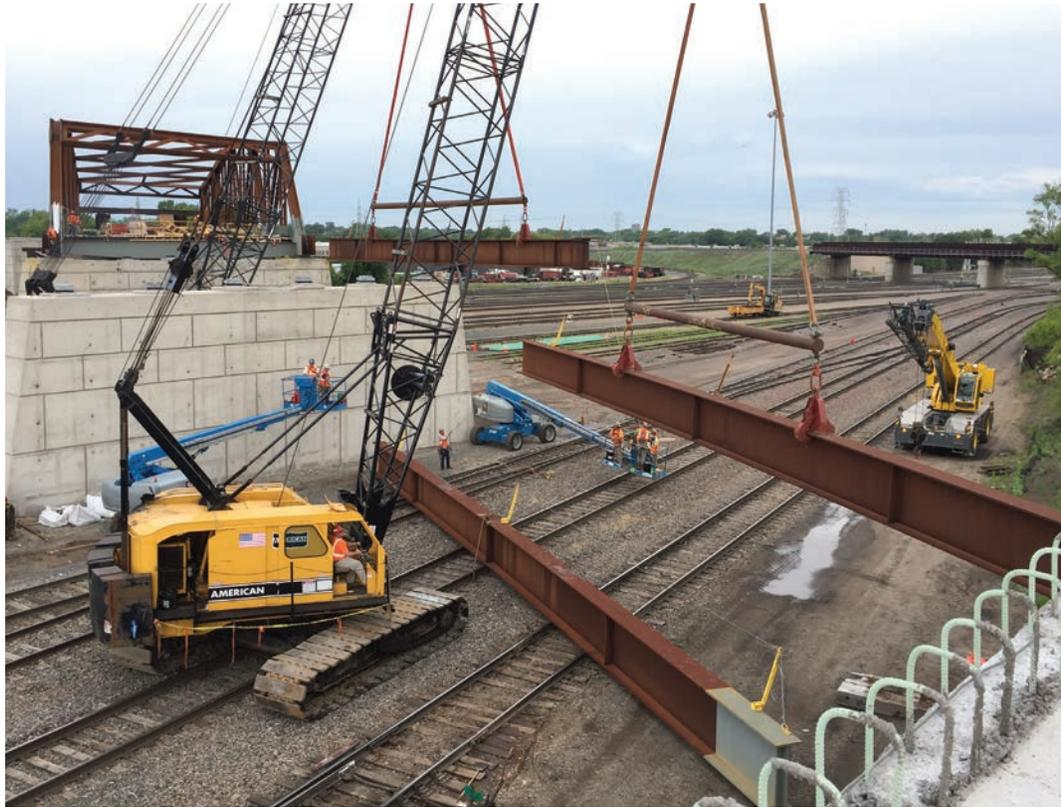
above: Erecting one of the two 127-ft-long approach spans, which are supported by conventional plate girders.
