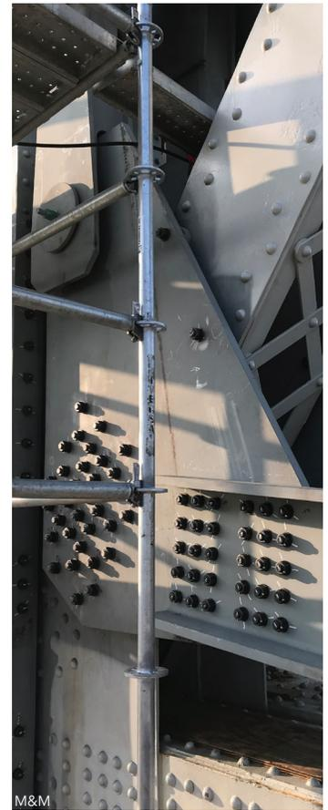
above: An outboard view of the knuckle plate on the Blue Water Bridge.
