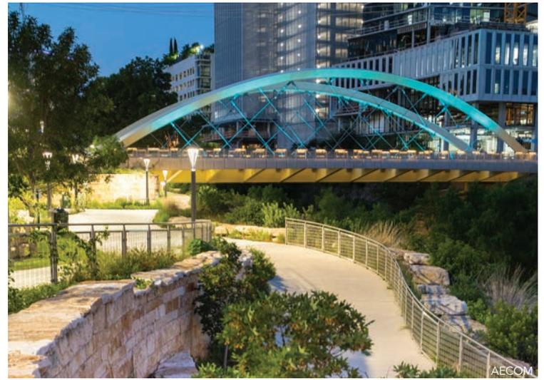
The cable hangers were fabricated off-site to the lengths specified in the contract documents. Each of the hanger cables was initially connected to the upper and lower pin plate with slack in the cable. The cables were then sequentially stressed to the target jacking forces provided by the erection engineer.
