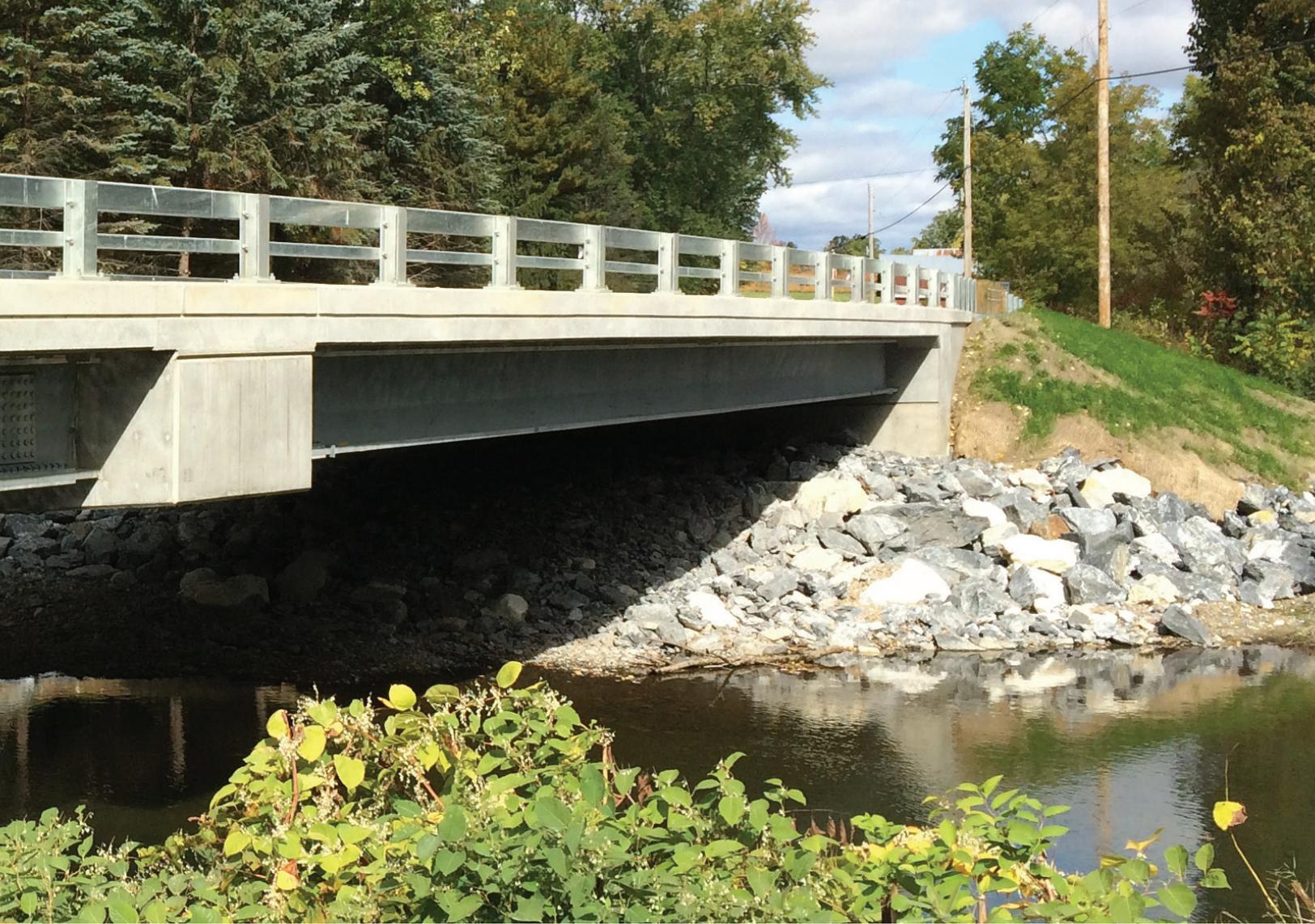
alignment was shifted to allow for a 6-ft, 6-in. shoulder on the inside of the curve to improve site distances and allow room for snowmobile passage across the bridge. The width of the pier cap matches that of the superstructure for clean lines and a pleasing aesthetic appearance.
