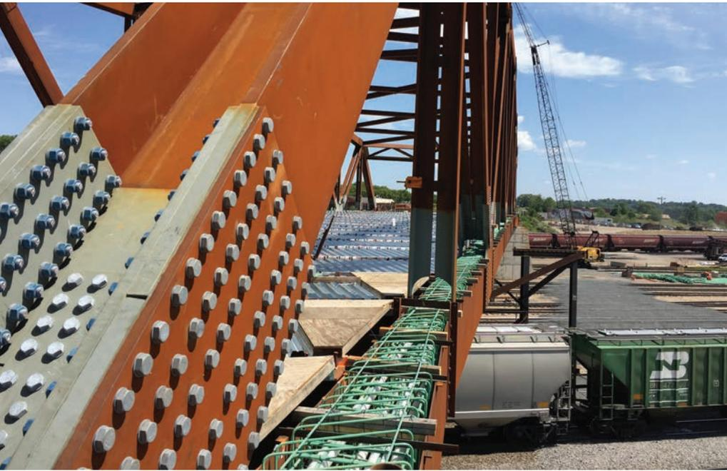
above and below: The bottom chord is a post-tensioned concrete member encased in a U-shaped steel shell.
