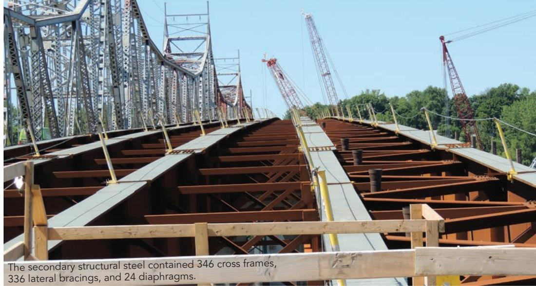
The secondary structural steel contained 346 cross frames, 336 lateral bracings, and 24 diaphragms.
