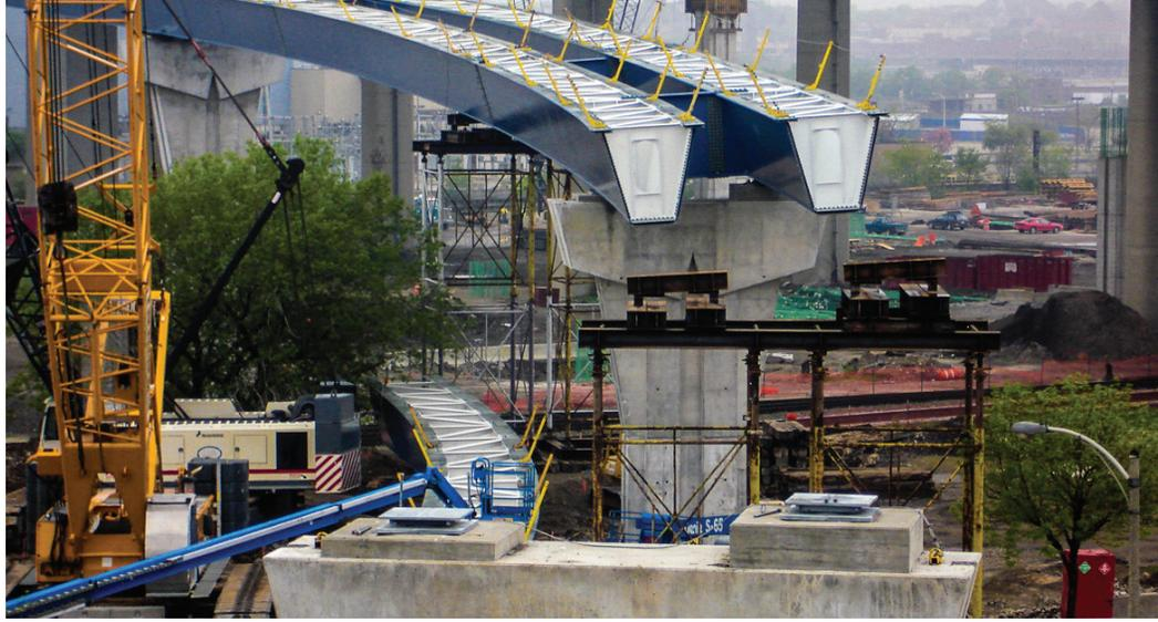
Milwaukee's Marquette Interchange twin-tub girder bridge project (to read about it, see "Steel Bridge News" in the March 2007 issue of *Modern Steel Construction*).
