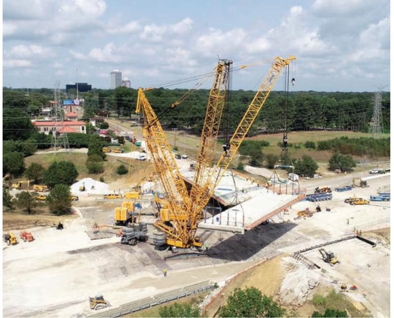
above and below: The Poplar Avenue roll-ins required only two 56-hour closures of I-240, significantly less time than would have been required had the bridges been built in place using concrete.
