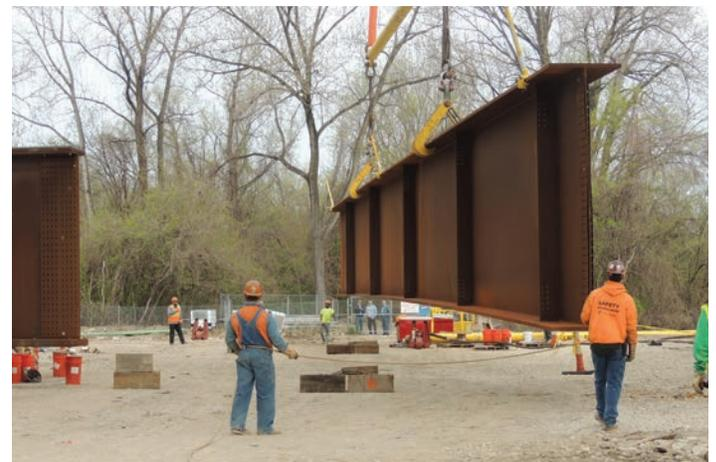
temporary support girder spanned between adjacent tower sections, and each hybrid tower—consisting of pipe piles, transition elements, and rented tower sections—was designed as a cantilevered column to eliminate the need for custom-fabricated, field-installed bracing between the towers.
