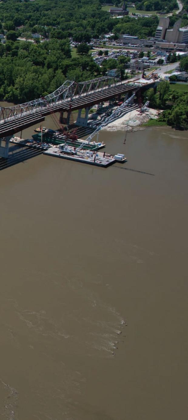
left: The superstructure for the new bridge, which uses 5,800 tons of structural steel in all, nearing completion.
