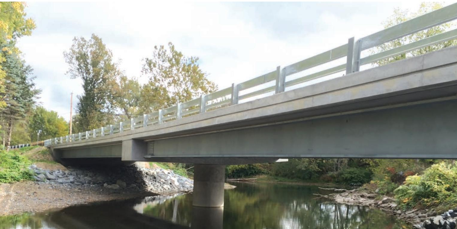
system was erected with full geometry control and all field splices and diaphragms were fully connected. Reinforcement was then tied, and the cap was cast around the girders. Once the cap had cured, the structural framing was disassembled and shipped to the project site.
