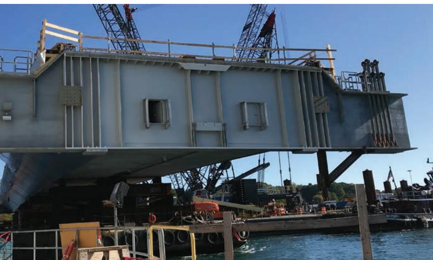
within the concrete deck, with minimal cover to the top of the steel, and the design team implemented a direct load path into the box section. In addition to providing a predictable load path, this alignment eliminated the need for supplemental track support structures and ultimately reduced the span weight.
