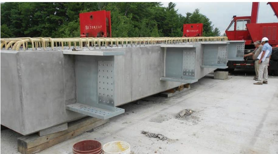
left: The precast cap with girder stubs being prepared for transport.
