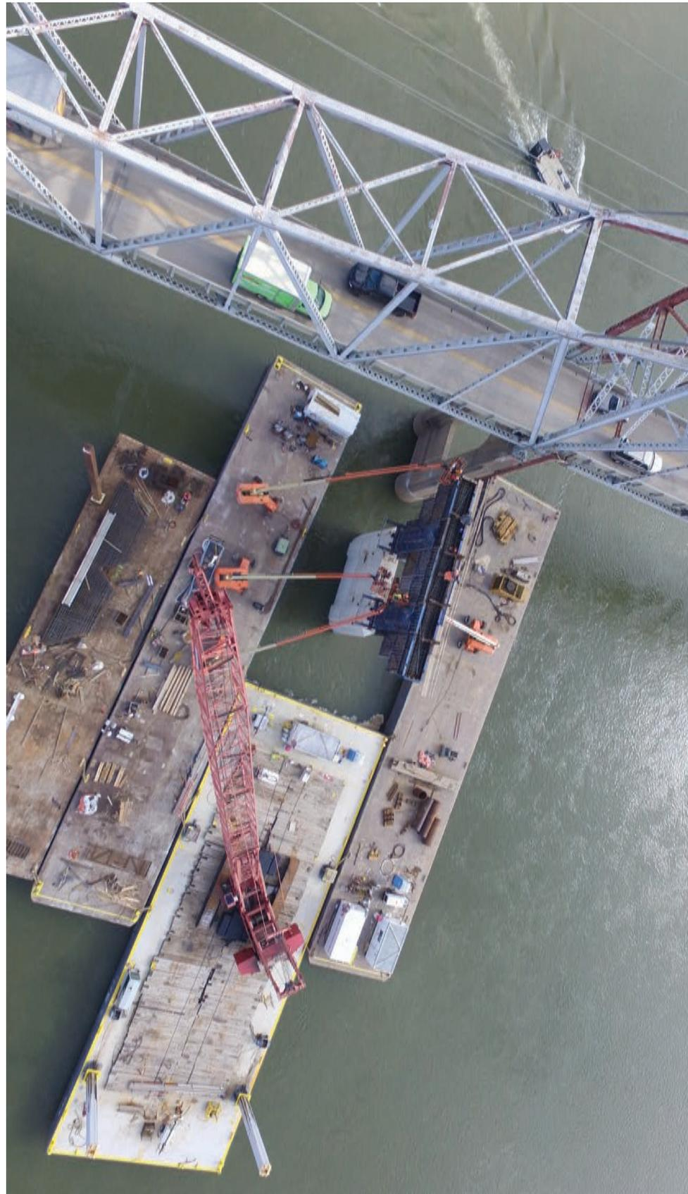
and temporary shoring for the bridge. A flexible support bracket system was developed to reduce the length of girder cantilevers during erection. The bracket system was designed to move from pier to pier, resulting in a significant weight savings in steel falsework and river-based shoring.
