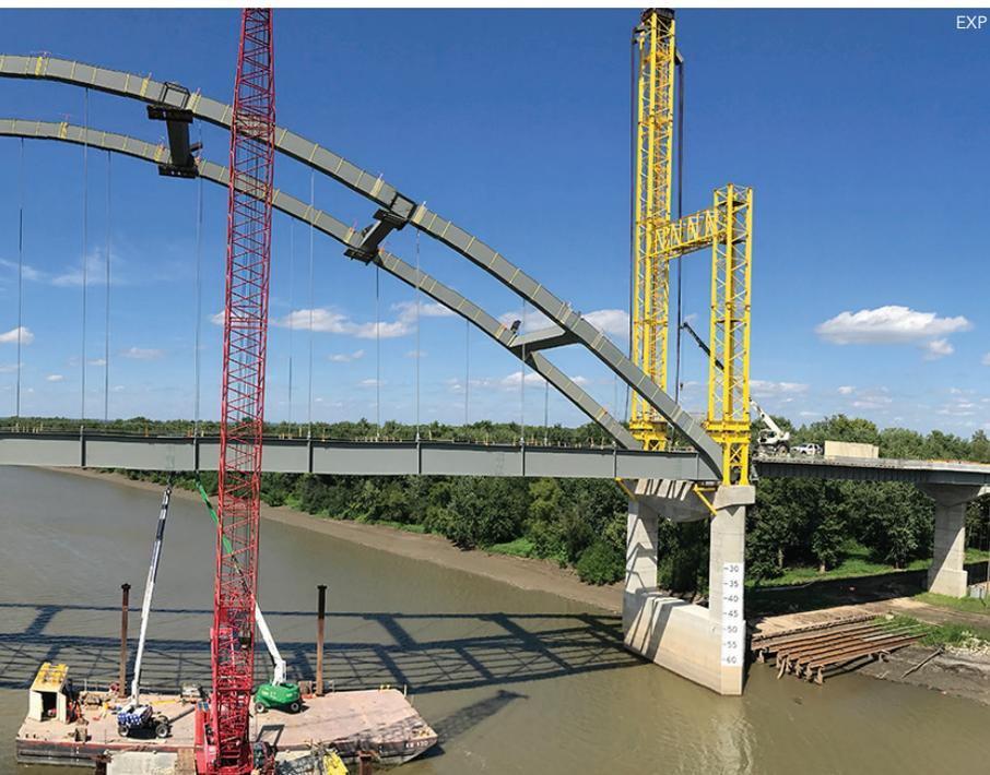
above and below: The new bridge carries two 12-ft lanes and two 10-ft shoulders and provides nearly 74 ft of vertical navigation clearance above normal pool. The bridge's design required complex analysis and used state-of-the-art programs to determine loads and perform design checks.
