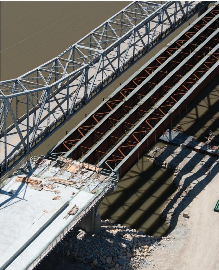
above and left: The bridge's superstructure is made up of 75 individual plate girders whose lengths vary from 100 ft to 140 ft and whose depths range from 18 ft at the support piers to 10 ft, 6 in. at the midspans.
