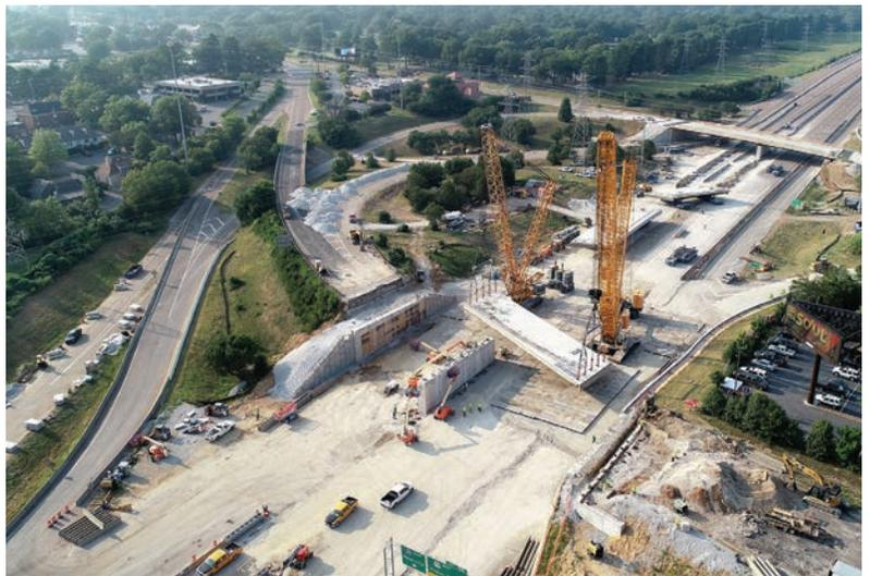
below: On average, opting for steel instead of concrete reduced the depth of the Poplar Avenue structures by about 30% and the weight by more than half.
