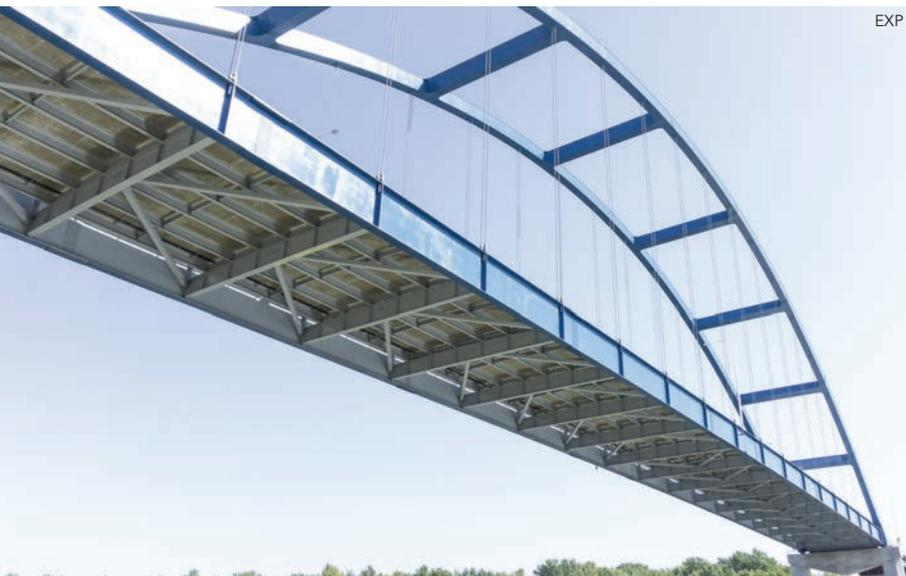
The substructures consist of stub-type abutments and architecturally enhanced hammer-head approach piers and dual-column portals for the main span, all founded on steel H-pile foundations. The foundations were designed with all vertical H-piles counting on the soil-structure interaction to resist lateral loads. Using all vertical H-piles as opposed to conventional batter piles resulted in a simple and constructable pier and cofferdam system, and helped reduce foundation costs by 40%.
