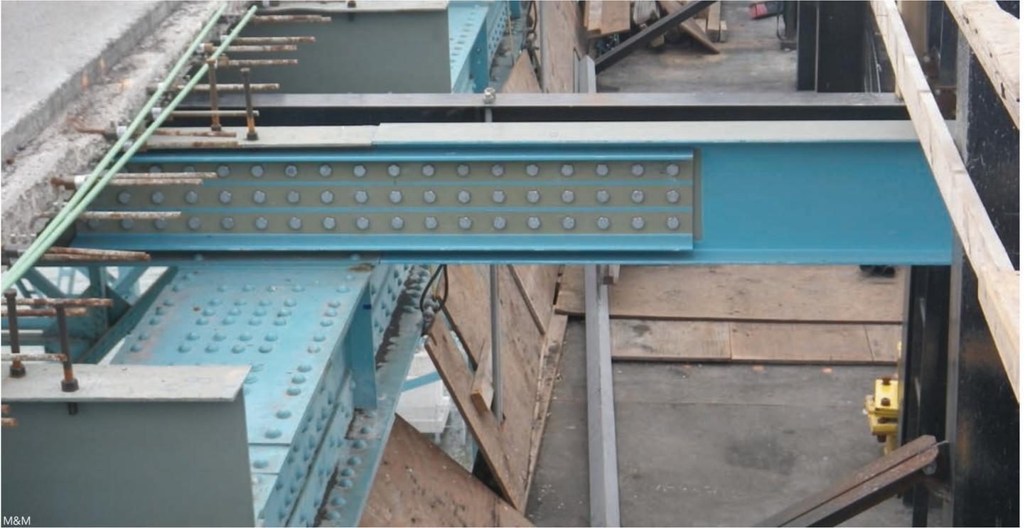
A primer with a cure time of 19 hours was used on a steel railing replacement project on the Ambassador Bridge between Detroit and Windsor, Canada.
