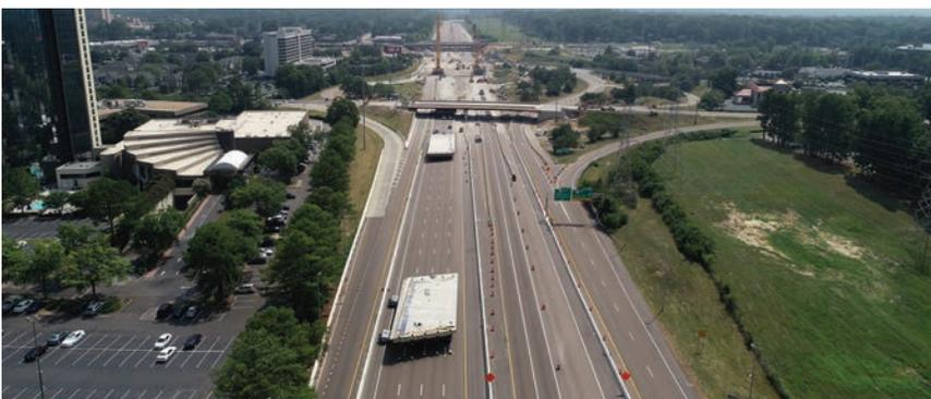
above: Following construction at the bridge farm, the Poplar Avenue structures were rolled two miles down I-240 to the project site on self-propelled modular transporters (SPMTs).
