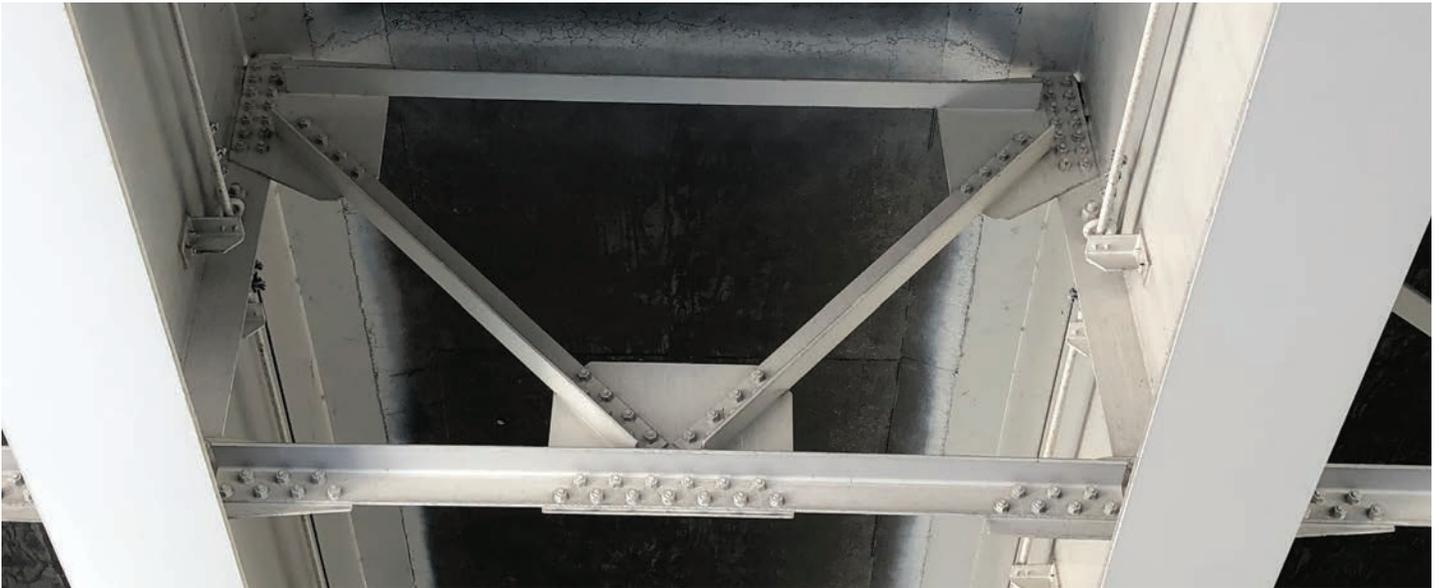
A K-type cross-frame with bolted end connections—not recommended unless absolutely necessary.
