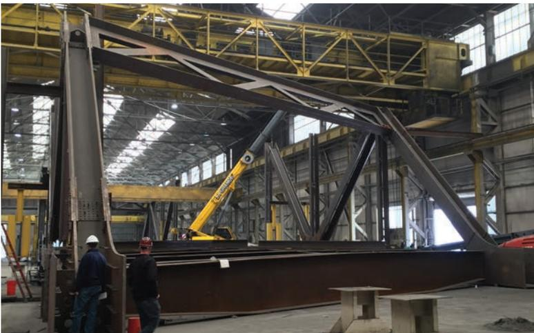
above and below: Fabricator Industrial Steel Construction, Inc. (ISC) first assembled the bridge trusses in its Gary, Ind., shop to ensure that everything fit together. The steel was then disassembled and trucked to the bridge site.
