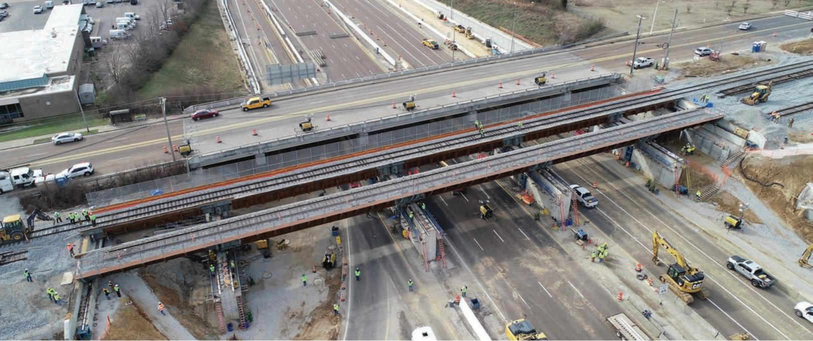
above: Sliding in the second NSR bridge. This replacement railroad crossing comprised a total steel weight of 950 tons and a maximum span of 88 ft.
