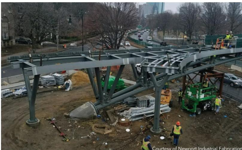
fixed supports, and applying a service live load since the design load of 120 psf would be unlikely at a temperature of  $-30^{\circ}\text{F}$ .
