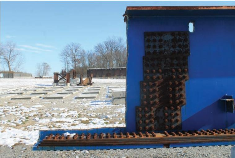
This is a portion of an all-welded 1956 railway bridge from the Pennsylvania Railroad in New Jersey. The girder sustained a brittle fracture at a detail now known to be susceptible to constraint-induced fracture (CIF). The girder sports a complex bolted repair. Though unrelated to the fracture, holes were drilled to arrest the fatigue cracks at the top of the vertical stiffener.
