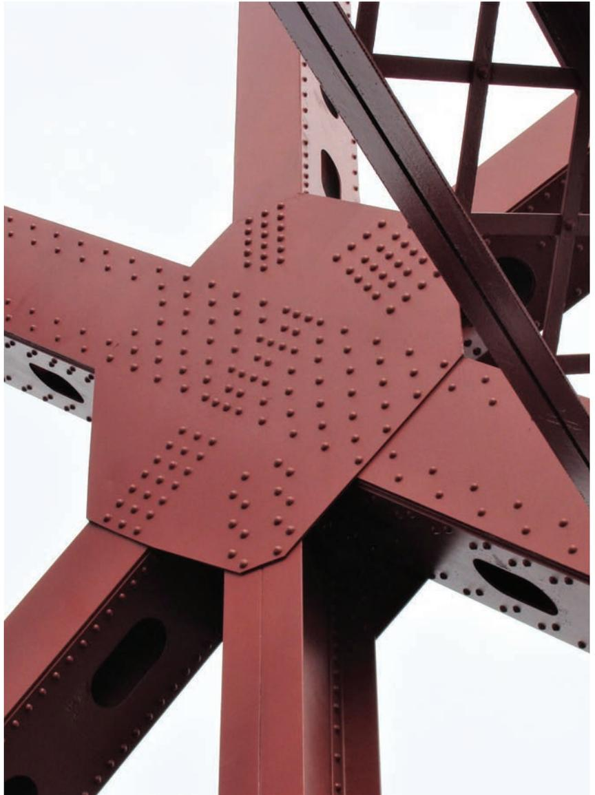
above: A riveted built-up connection on the Mathews Bridge over the St. Johns River in Jacksonville, Fla., showing built-up tension members.
