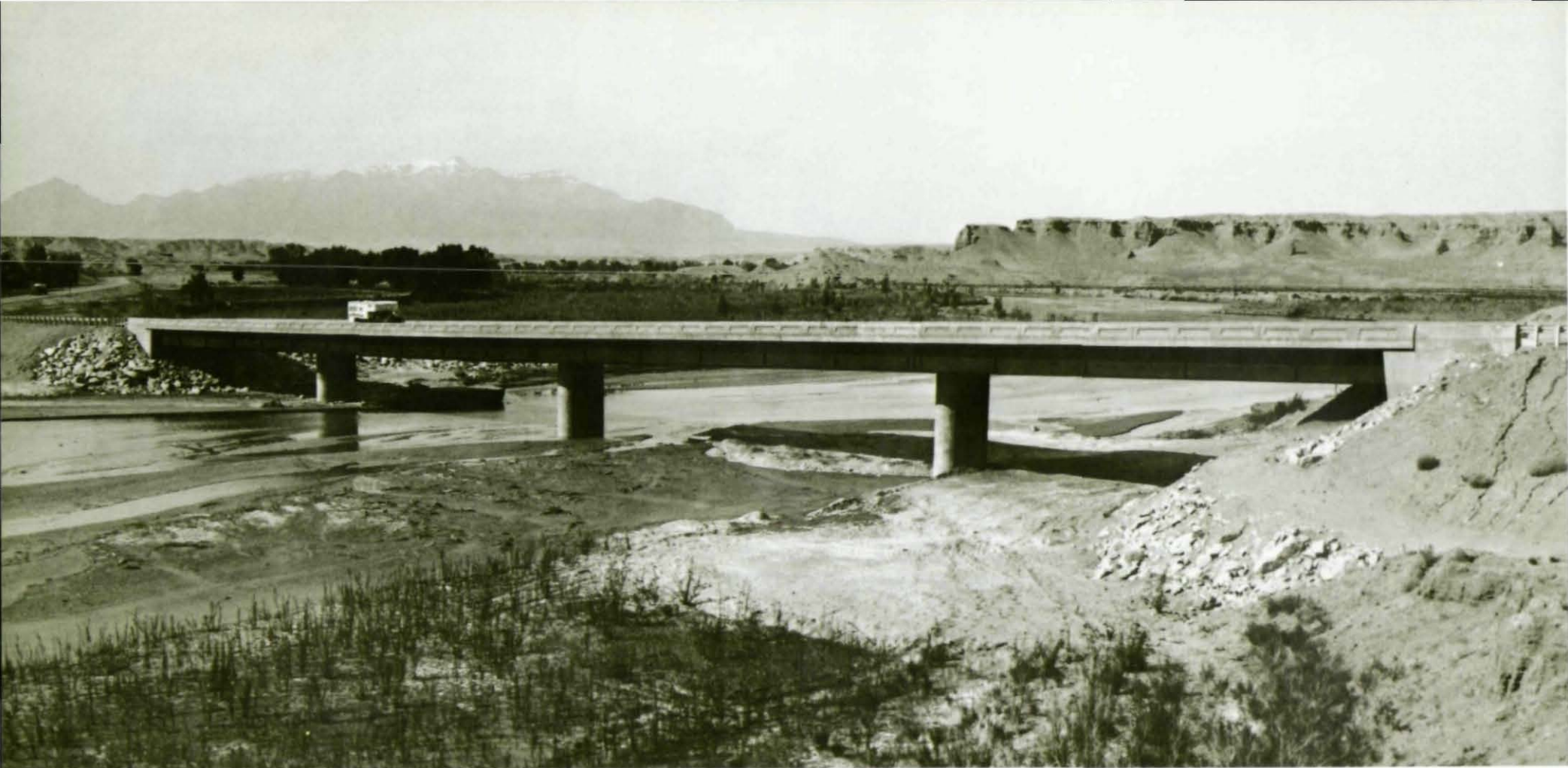
State Route 24, near Hanksville, Utah Span Lengths: 104'—2 at 130'—104'
