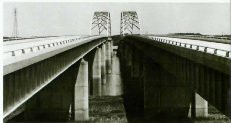
Marshall and Livingston Counties, Kentucky Span Lengths: 4 at 195'—534'—4 at 195'
