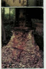
The seriousness of America's bridge problems is typified by the arch bridge above. Deterioration of the deck (above right) permits an observer to put a hand through a hole. The pier (above) originally had 6 in. of concrete over the reinforcing bars. This bridge had to be closed. On another bridge, pad supporting a steel column (bottom) has spalled away.
