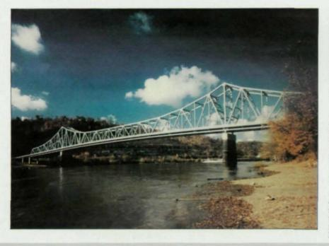
The original 70-year-old Sewickley Bridge needed replacing and the primary requirement was to minimize closure time. By using the two original river piers, portions of the original abutments, and a steel structure, the new bridge was in use only 17 months after closing. Steel was used to minimize structure weight and depth, yet the new bridge is 4 ft. wider than the old.
