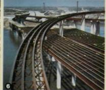
5. Large-Scale Production HSSI's facilities accommodate the most complex projects, like these curved trough girders, assembled in yard for reaming to insure a proper fit in the field.
