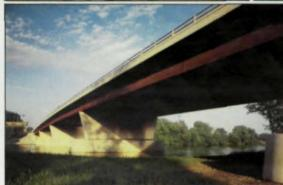
New designs in truss bridges (top and above) and box girder bridges (left) demonstrate steel's ability to combine beauty and construction economy, Weathering steel bridges of either design blend into the environment and offer reduced maintenance.
