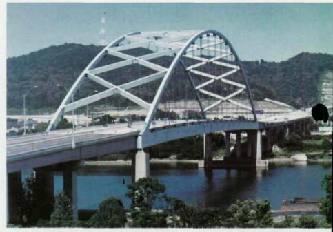
The 1984 Prize Bridge winner in the long span category, this single-span tied arch bridge carries traffic over the Ohio River south of Wheeling, West Virginia. A century of experience in building bridges with steel is now "built in", promising structural integrity and displaying the evolution towards simplicity and economy.
