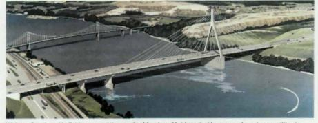
Weirton-Steubenville Bridge, one of the steel cable-stayed bridges that has proved most competitive in bidding on alternative designs.
