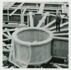
Stainless steel substructures for fusion reactor at Princeton, New Jersey.
