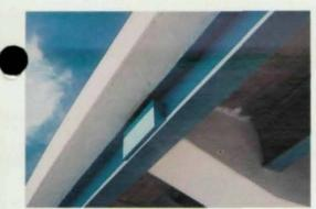
Innovative design idea: integral, steelgirder, prestressed concrete cap, was used where vertical and horizontal clearance problems prevented the use of conventional dropped caps.
