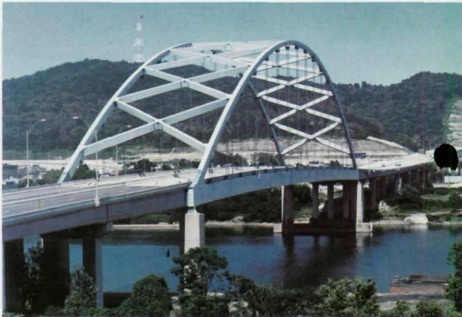
The 1984 Prize Bridge winner in the long span category, this single-span tied arch bridge carries traffic over the Ohio River south of Wheeling, West Virginia. A century of experience in building bridges with steel is now "built in", promising structural integrity and displaying the evolution towards simplicity and economy.
