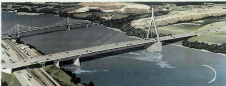
Weirton-Stuebenville Bridge, one of the steel cable-stayed bridges that has proved most competitive in bidding on alternative designs.
