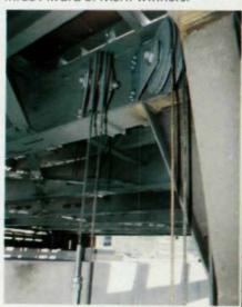
Partially opened lift span shows the double diagonal equalizer system in the Wells Street vertical lift bridge, Milwaukee, W1. (1986 Prize Bridge, Movable Span)
