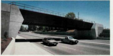
The Vista Avenue Railroad Bridge in Boise, Idaho (a 1986 Prize Bridge) utilizes weathering steel in a trapezodial steel box girder. Railroad tracks are supported from bottom of box
