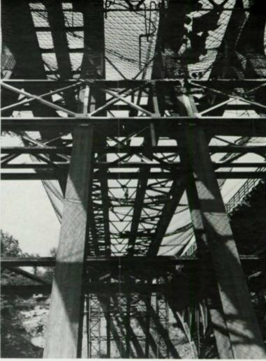
SINCO Nets protect ironworkers during steel erection on Rte 9W Bridge, Albany, NY.
