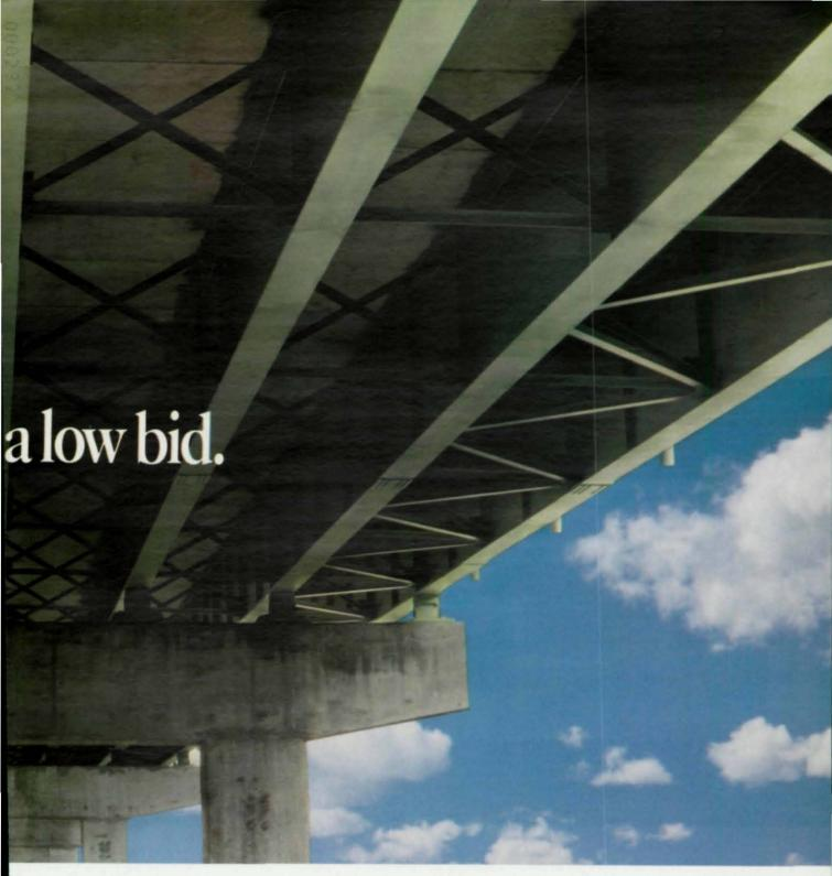
alent concrete section would weigh 200 tons and take four days to install. The use of steel also permitted a reduction in the number of piles and the amount of concrete required for the foundations.
