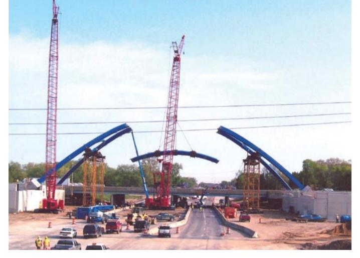
will be difficult. Therefore, the arch ribs are pressurized with air to prevent any internal moisture in an effort to prevent corrosion.
